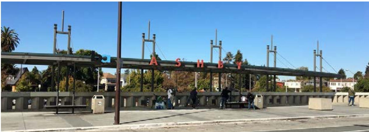
The Ashby BART Station
