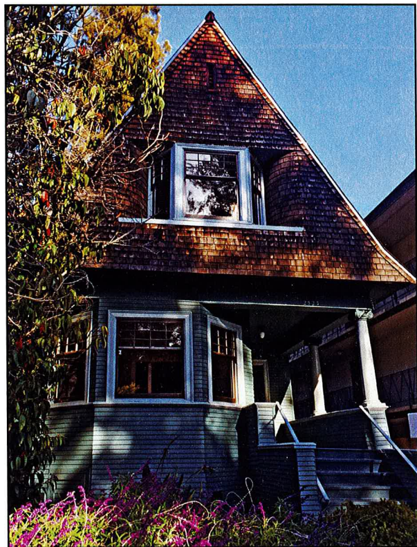
Fig. 6. Front façade. Anthony Bruce, 2021
