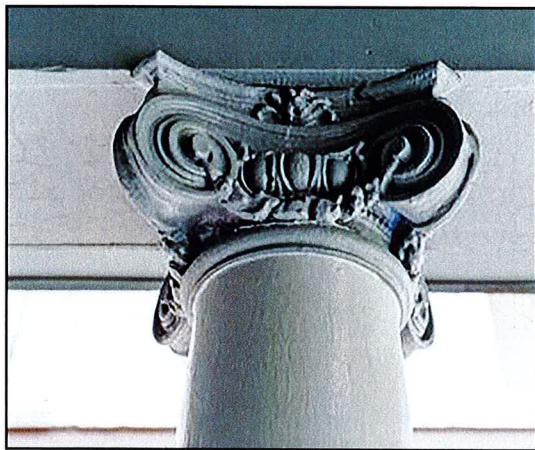
Fig. 8. An Ionic capital on a porch column. The Grubb Company listing photo, 2021
