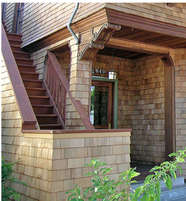
Figure 21. Porch openings, June 2021
