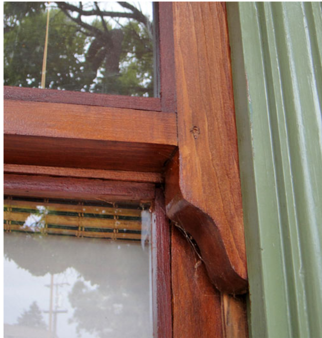
Figure 32. Restored window detail
