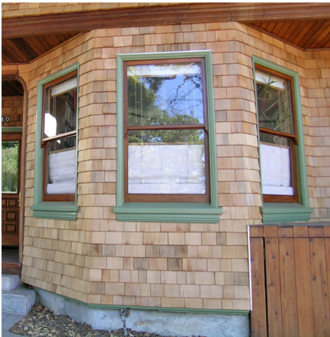
Figure 16. Skirt molding, soffit & scrolled bracket
