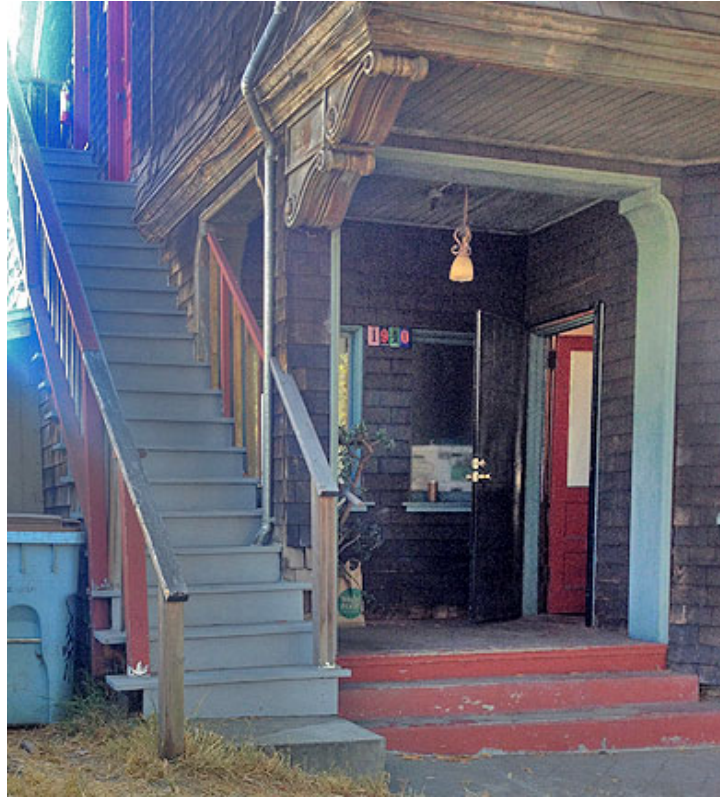
Figure 22. The porch pre-restoration, June 2018 (photo by owners)
