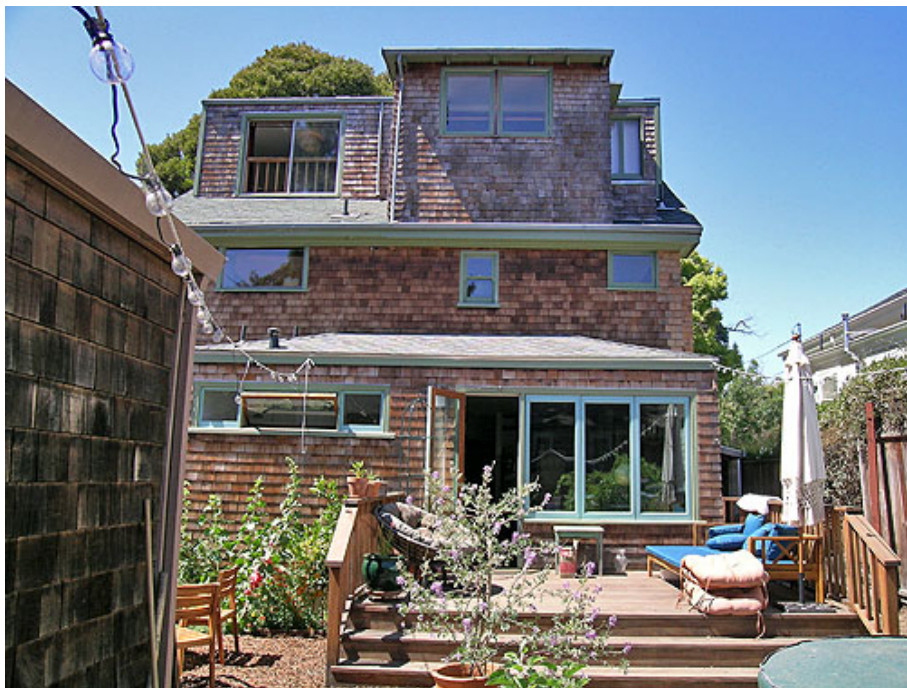
Figure 28. Rear façade post-renovation, June 2021
