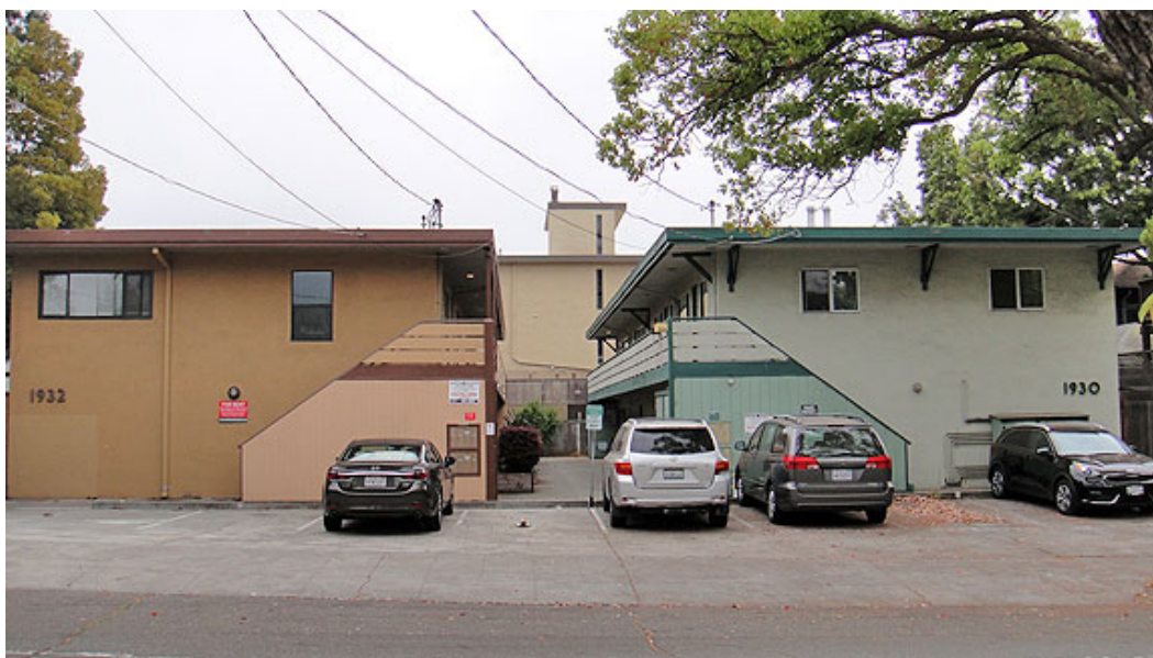
Figure 74. Apartments, 1930 & 1932 Hearst Avenue, built in 1955
