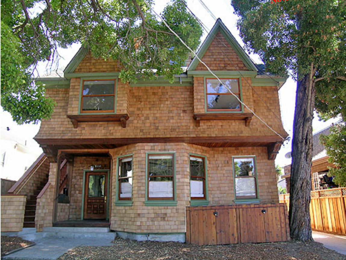
Figure 1. Street façade, June 2021
