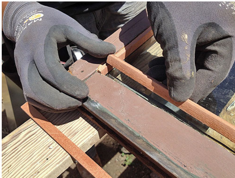
Figure 30. Window restoration work (photo by owners)
