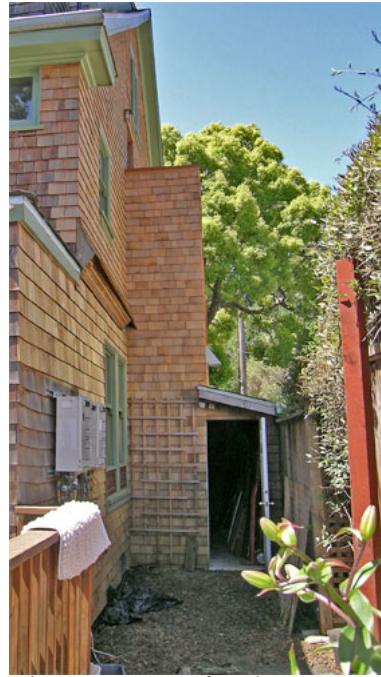
Figure 25. East façade, rear
