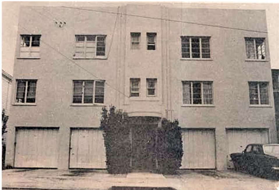
Figure 73. Reid Apartments (1946), 1915 Bonita Ave., in 1972 (Donogh files, BAHA)
