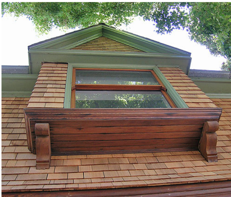
Figure 15. Boxed window, soffit & corbels
