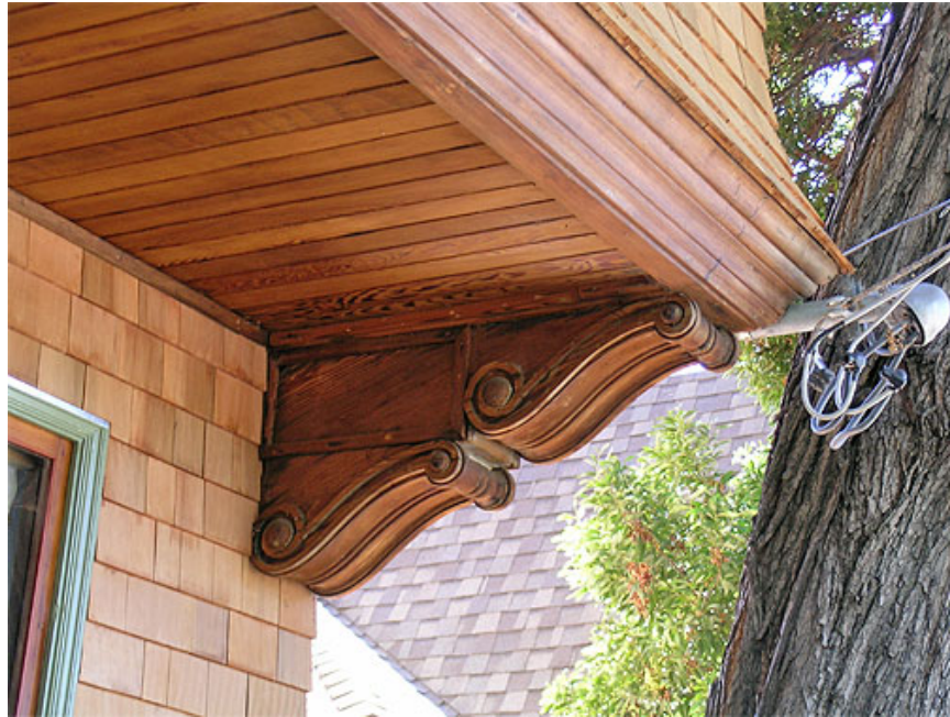
Figure 16. Skirt molding, soffit & scrolled bracket
