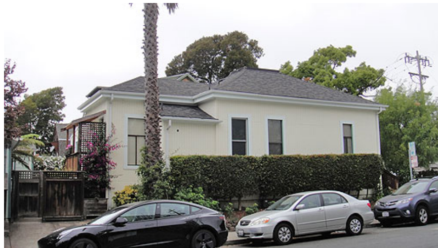
Figure 67. Joseph Clapp House, Milvia Street façade
