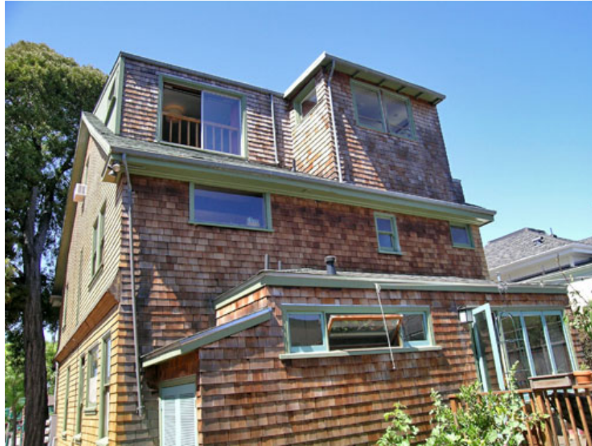
Figure 27. West & rear façades post-renovation, June 2021
