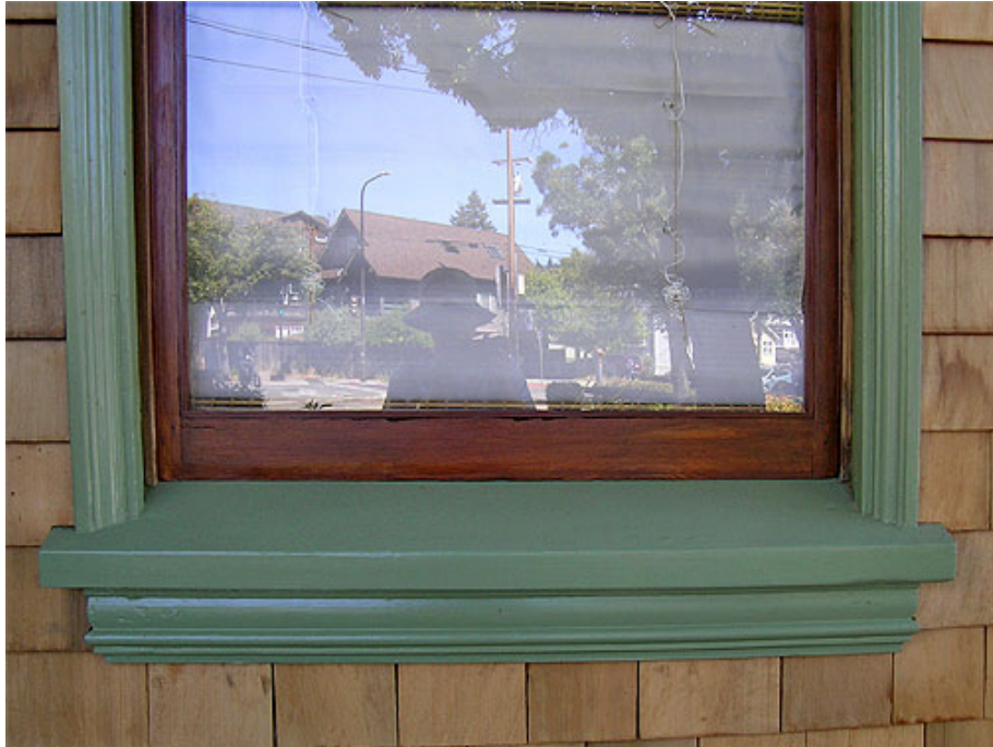
Figure 18. Window sash, trim & sill detail
