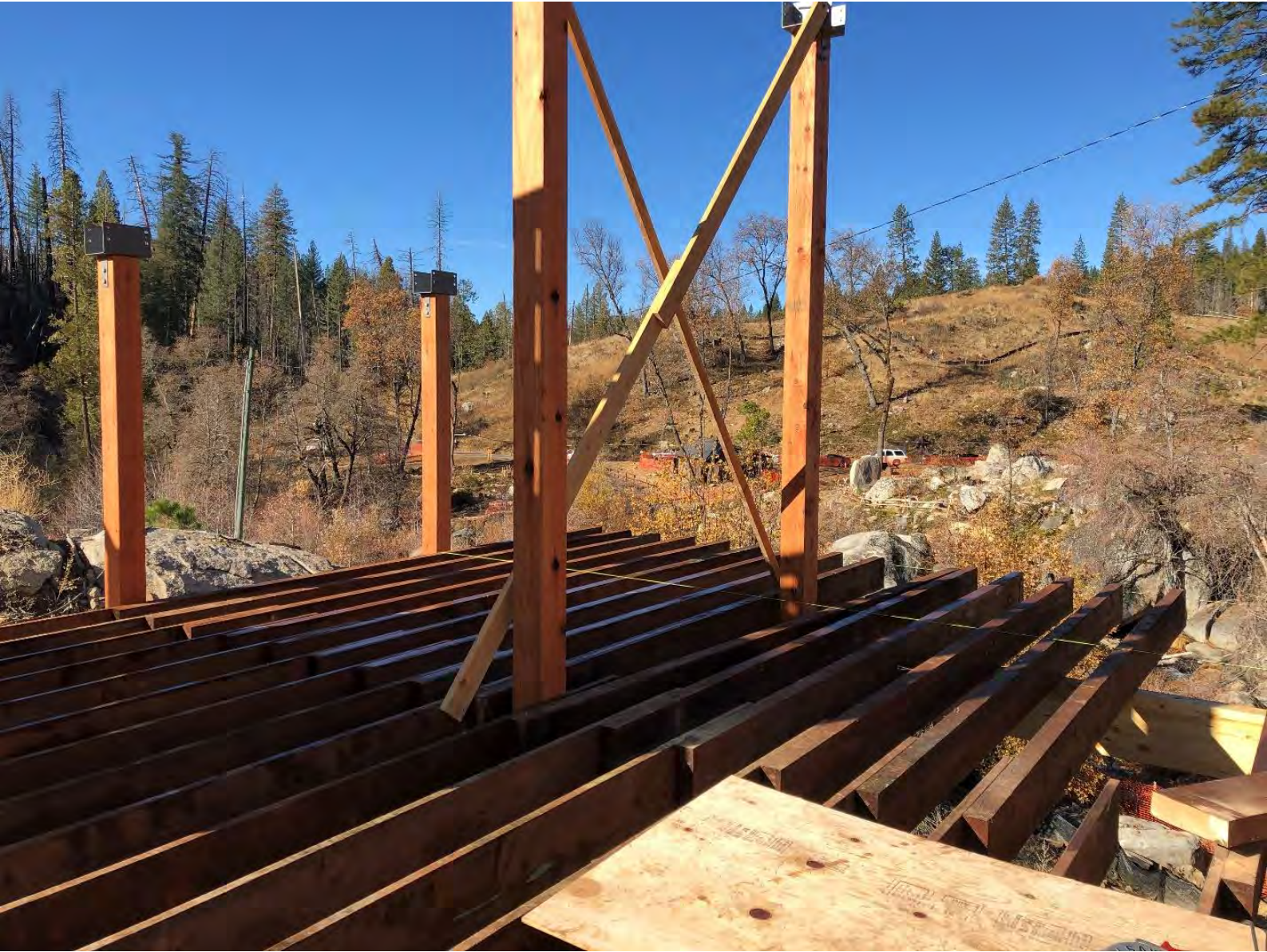
View from new Recreation Hall Deck
