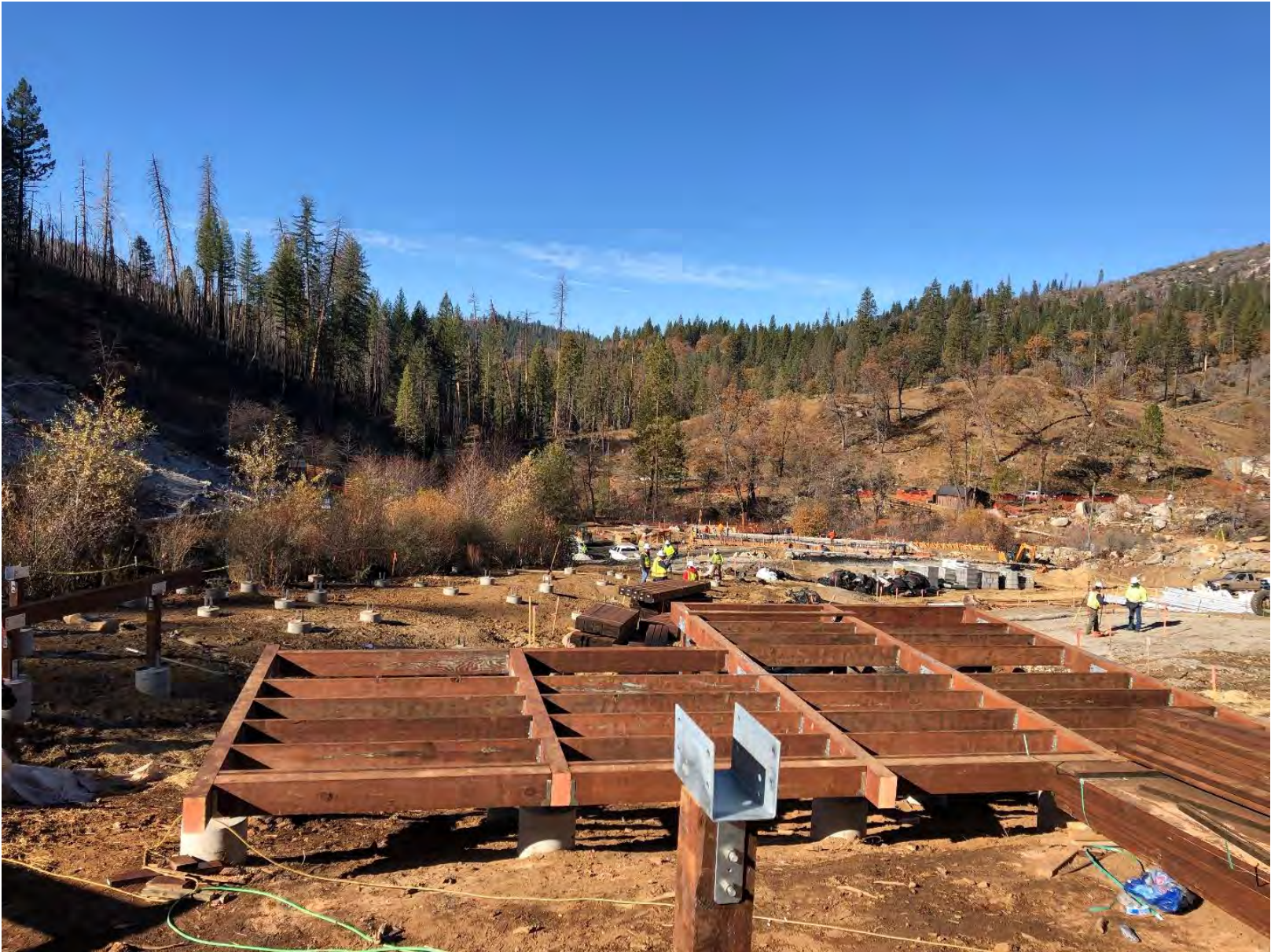
Floor / Deck for new Tent Cabin
