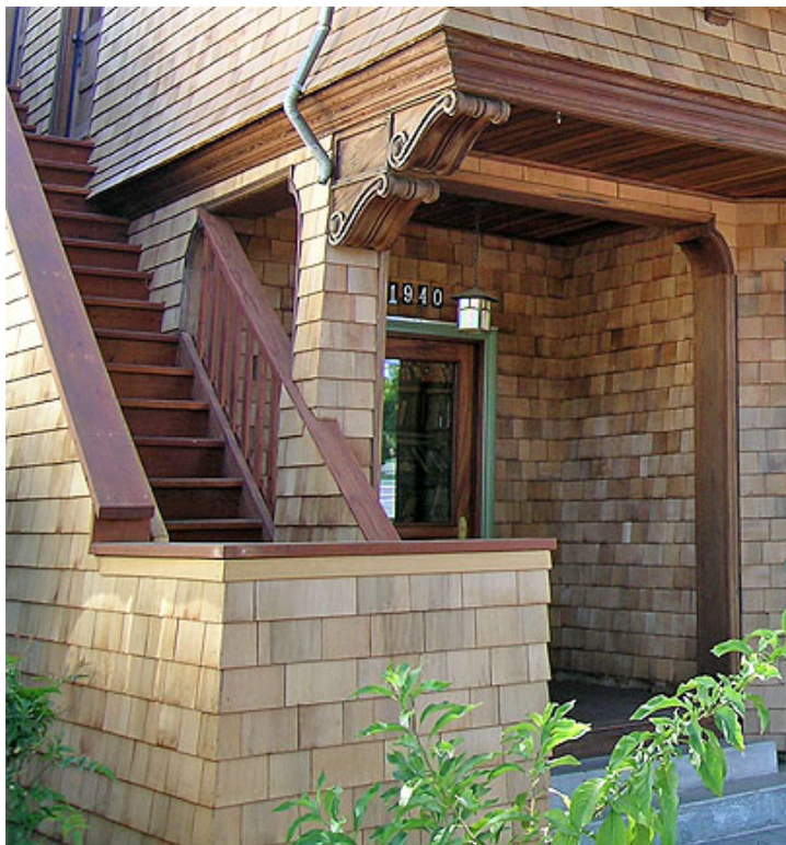
Figure 21. Porch openings, June 2021
