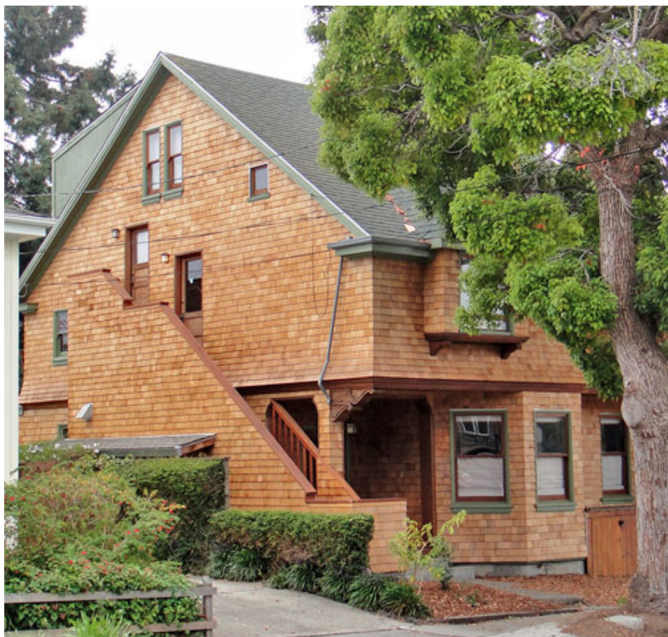
Figure 23. East façade & rebuilt staircase
