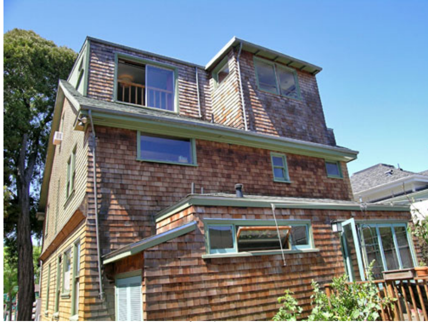
Figure 27. West & rear façades post-renovation, June 2021
