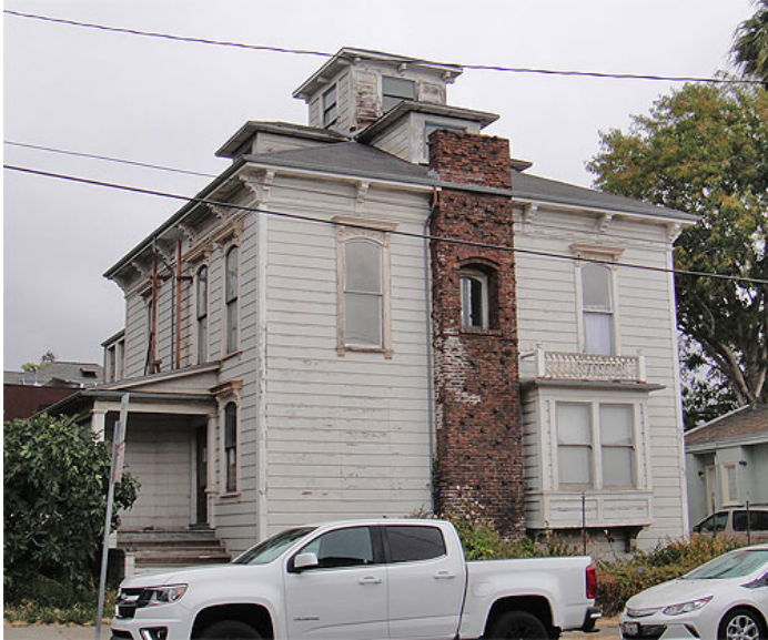
Figure 93. William G. Black House, 1930 Delaware Street
