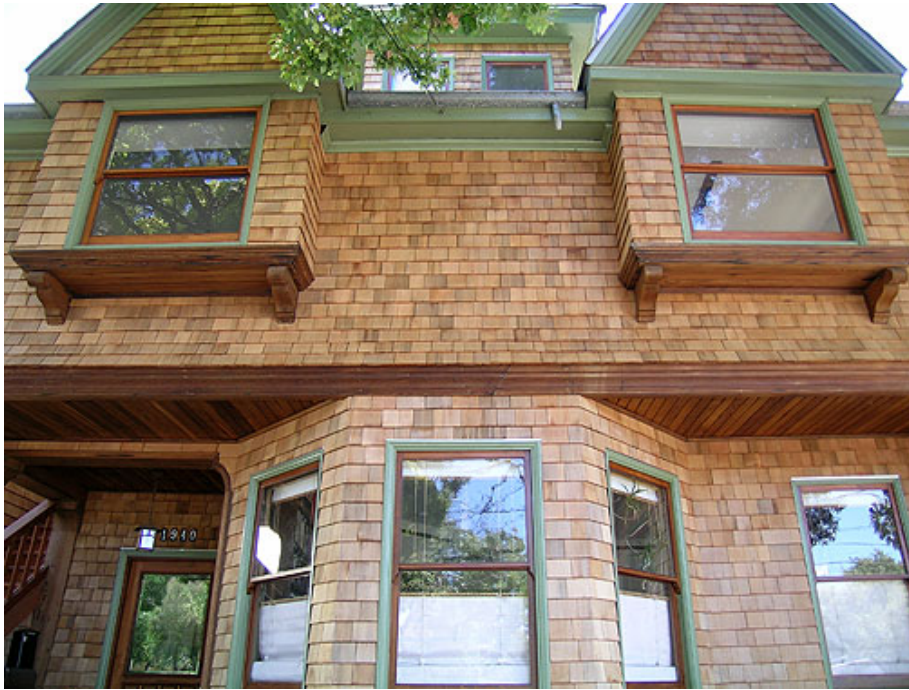
Figure 14. Front façade closeup view
