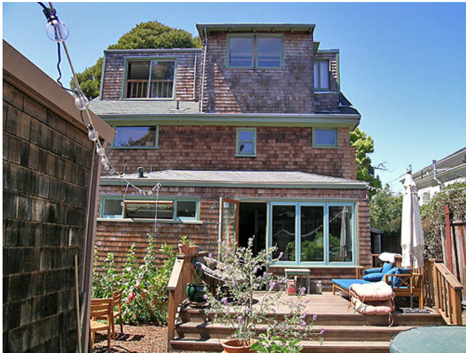
Figure 28. Rear façade post-renovation, June 2021
