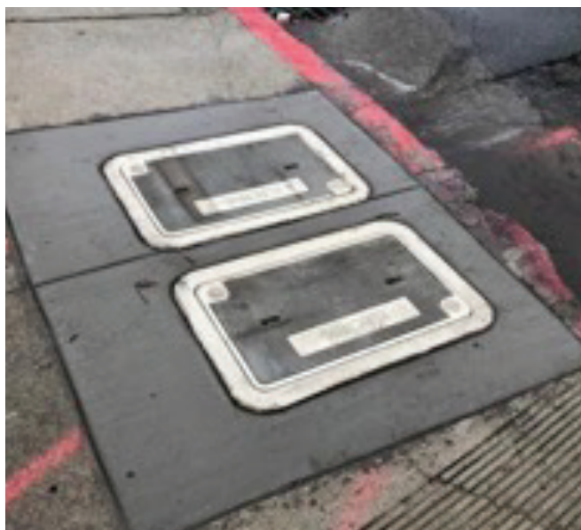
Sidewalk hazard repaired
