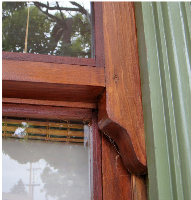
Figure 32. Restored window detail
