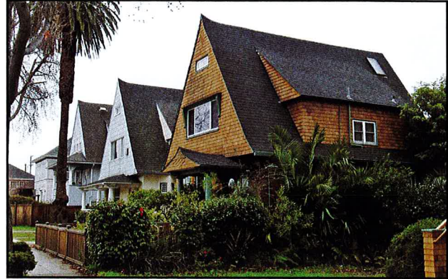
Fig. 22. Three High-Peaked Colonial Revival houses in a row in the 3000 block of Martin Luther King, Jr. Way. Daniella Thompson, 2005.
