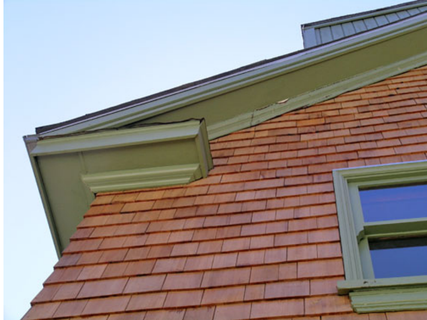
Figure 12. Closed roof eaves & gable-end return
