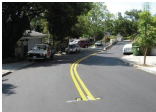
Completed street surface overlay
