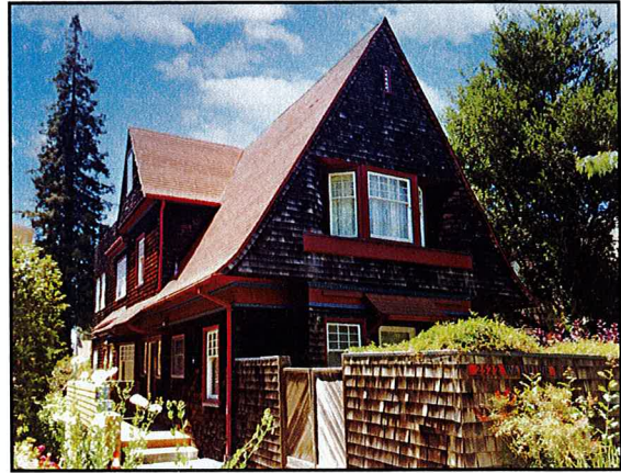
Fig. 29. The other High-Peaked Colonial Revival house that the Wurts’ built on Lot 5, directly behind the Wurts-Lenfest House. Anthony Bruce, 2021.
