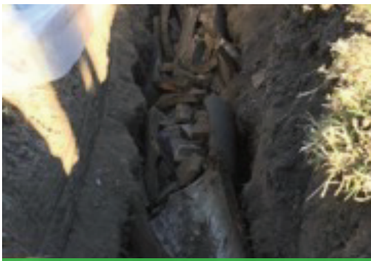
Deteriorated pipe
