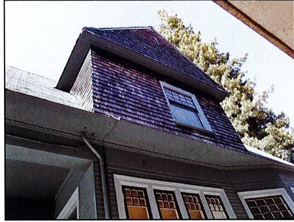
Fig. 5. The south dormer over the group of four entry hall windows. Daniella Thompson, 2021
