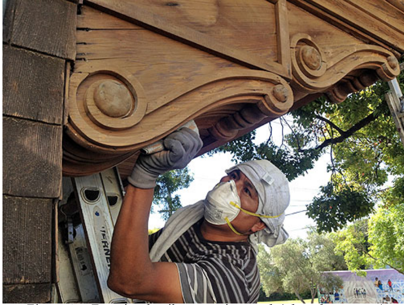
Figure 31. Exterior detail restoration work (photo by owners)
