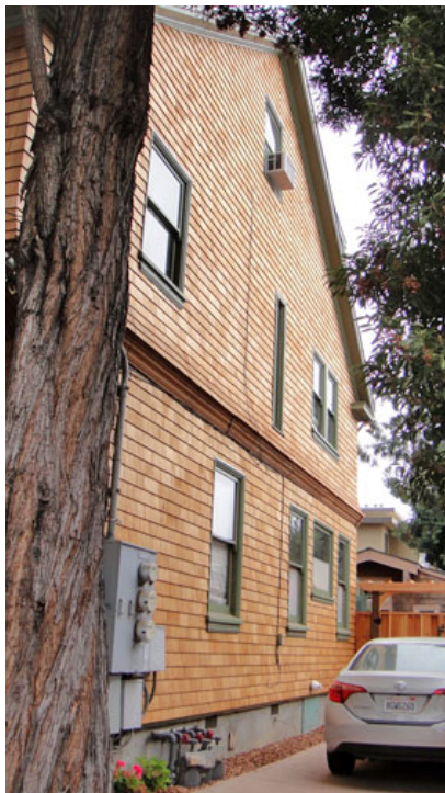
Figure 26. West façade post-restoration
