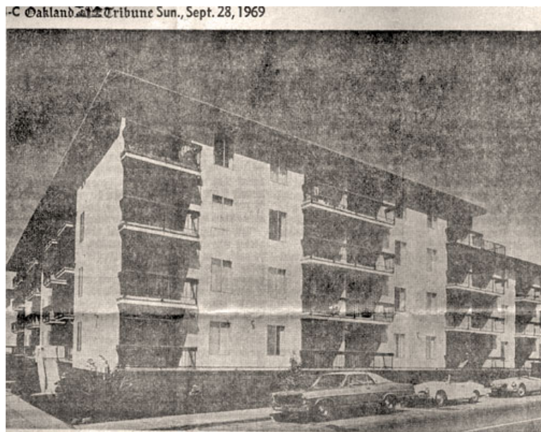
Figure 77. Smith & Haley apartments, 1945 Berkeley Way (Oakland Tribune, 28 Sept. 1969)
