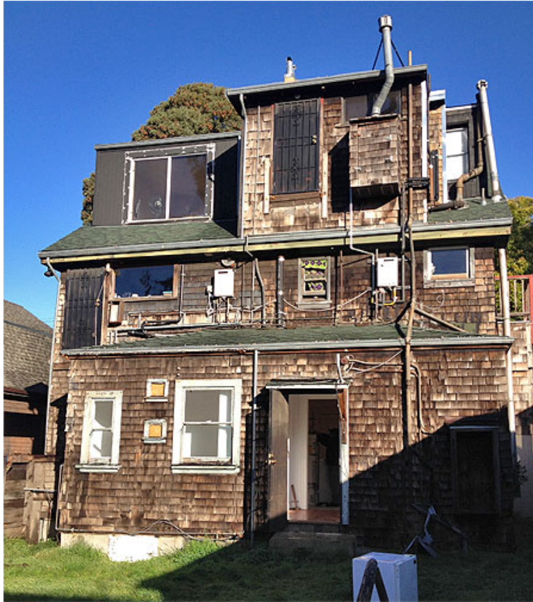
Figure 29. Rear façade in November 2017 (photo by owners)
