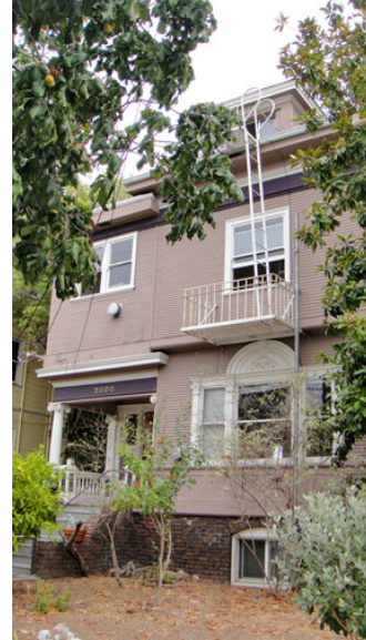
Figure 94. William H. Wharff House, 2000 Delaware Street
