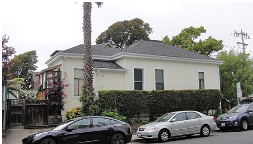
Figure 67. Joseph Clapp House, Milvia Street façade
