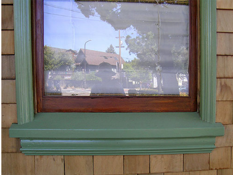
Figure 18. Window sash, trim & sill detail
