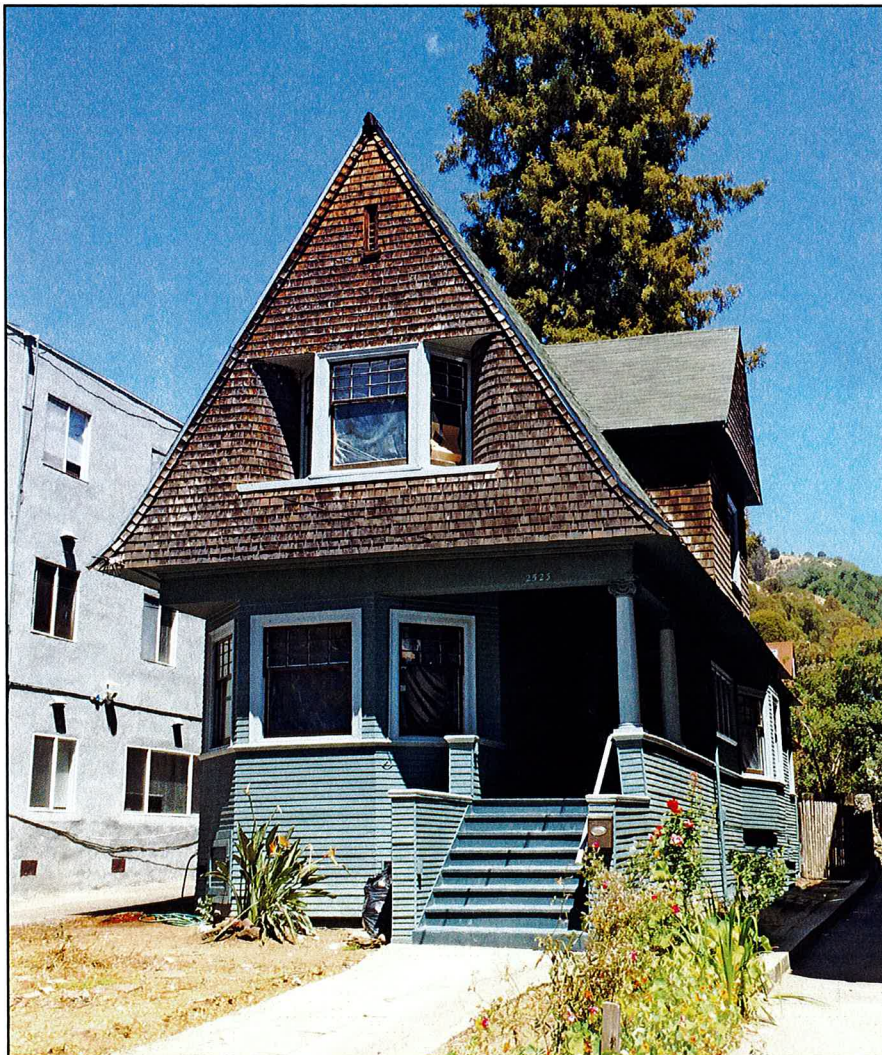
Figure 1. Street (west) façade of the Wurts-Lenfest House. Anthony Bruce, 2021
