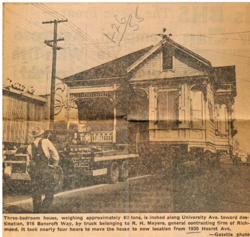
Figure 68. Dam House being moved from 1930 Hearst Ave. to 916 Bancroft Way (Berkeley Daily Gazette, 26 January 1955)
