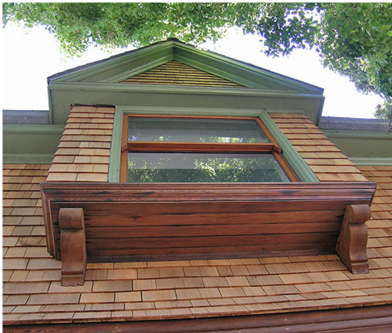
Figure 15. Boxed window, soffit & corbels
