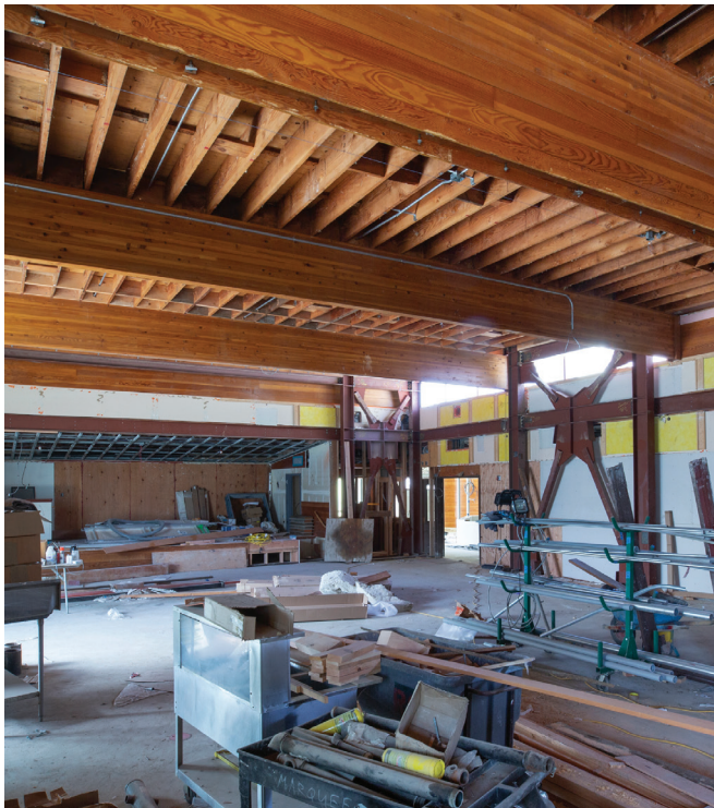
North Berkeley Senior Center in Construction
