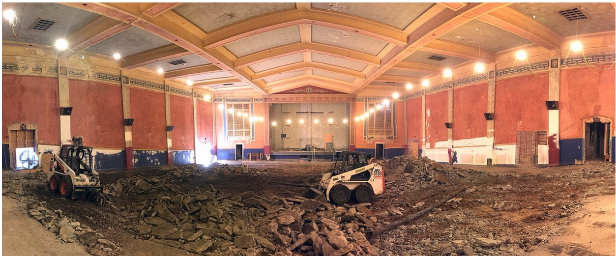
The UC Theatre 2015 (Started Renovation)
