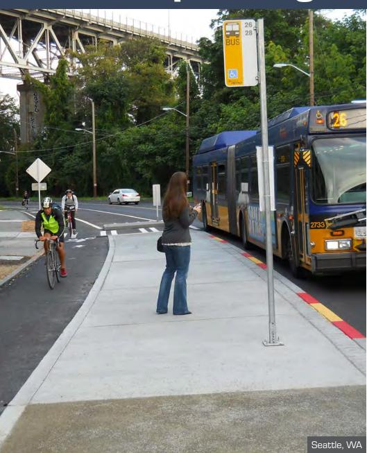
Designing a safe, comfortable, and functional bus stop for all users with special consideration to bicycle users is a primary purpose of this guide. Local jurisdictions are implementing more separated bike lanes on transit corridors and need design guidance to safely and seamlessly maintain bikeways through the bus stop. Based on common roadway and bikeway configurations, transit operations, and other considerations, five bus stop design typologies have been identified:
