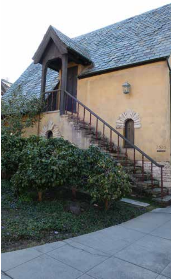
Fig.48 - Carriage house front (north)
