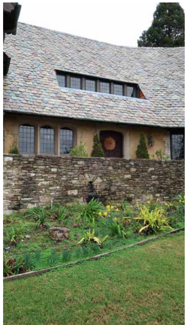
Fig.18 - Front terrace, entry way and roof
