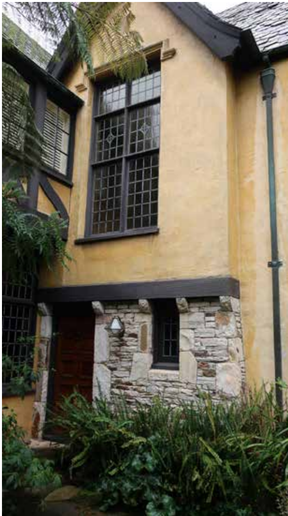
Fig.42 - Rear (east) entry
