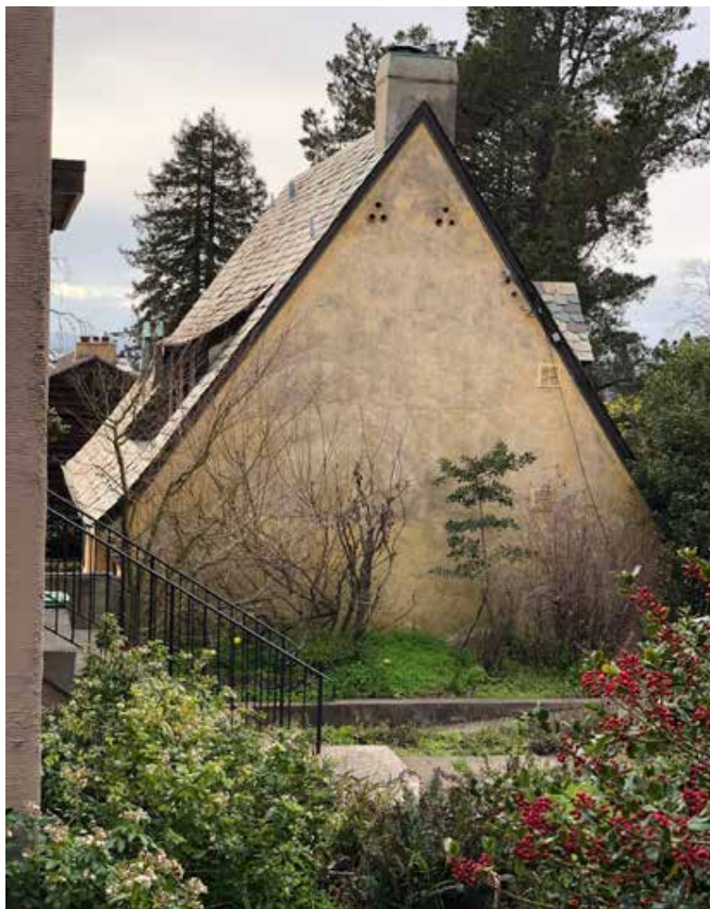
Fig.51 - Carriage house east side
