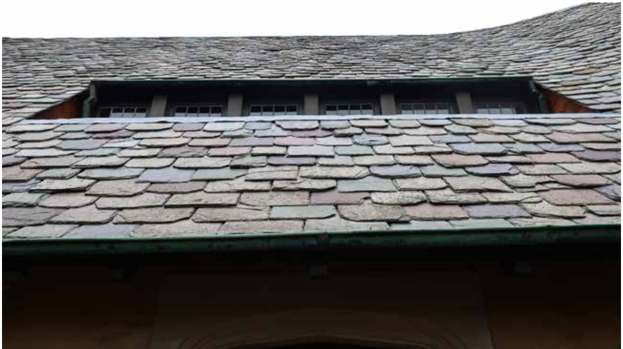
Fig.26 - Window opening at front roof
