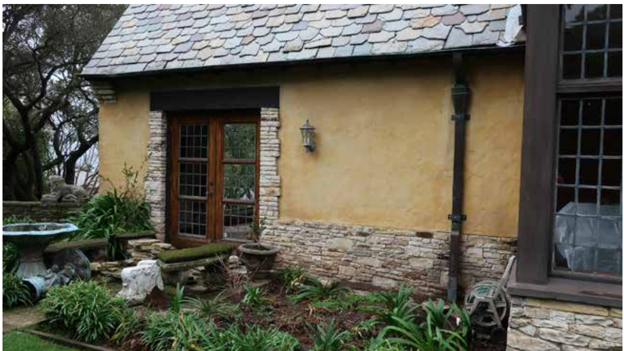
Fig.46 - South end rear elevation
