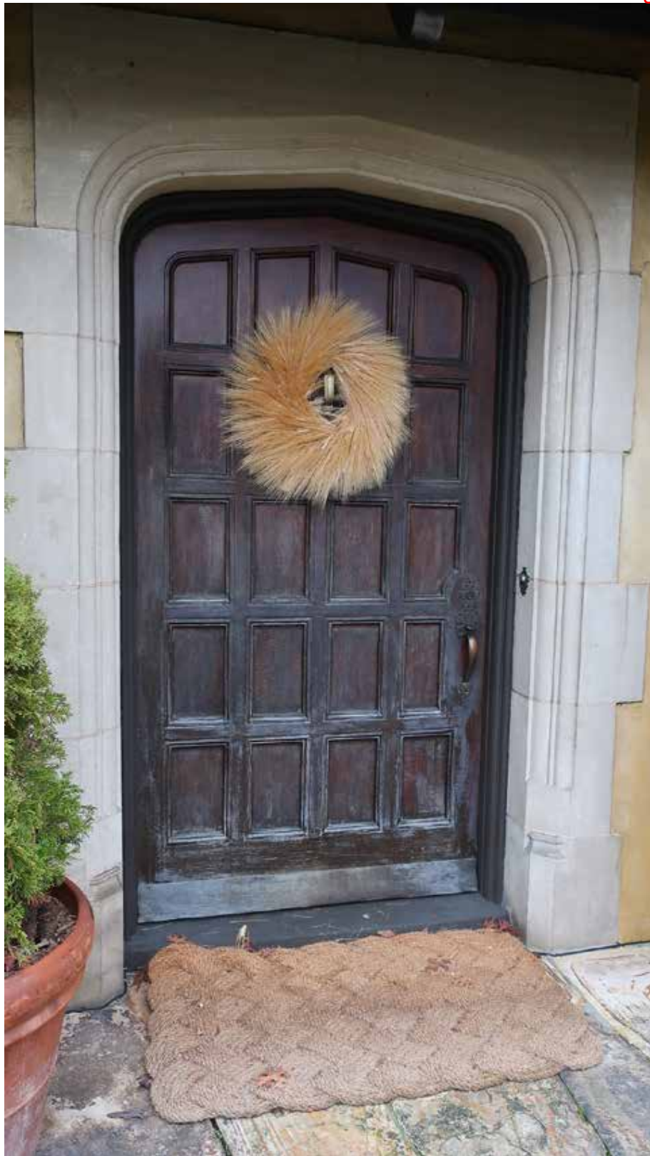
Fig.22 - Front entry door
