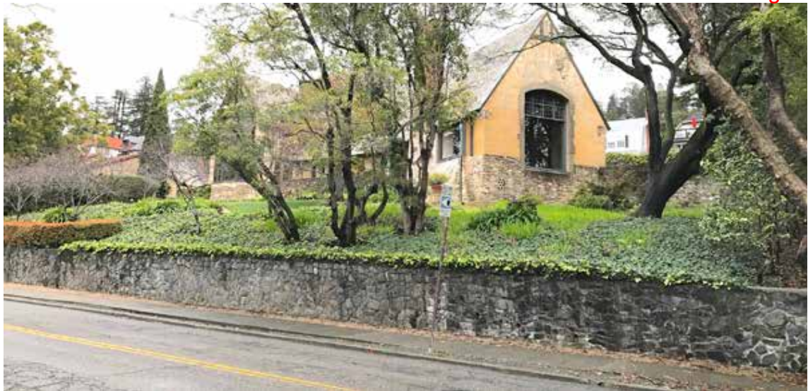
Fig.5 – 2526 Hawthorne, from Euclid Ave. with c1909 retaining wall in foreground
