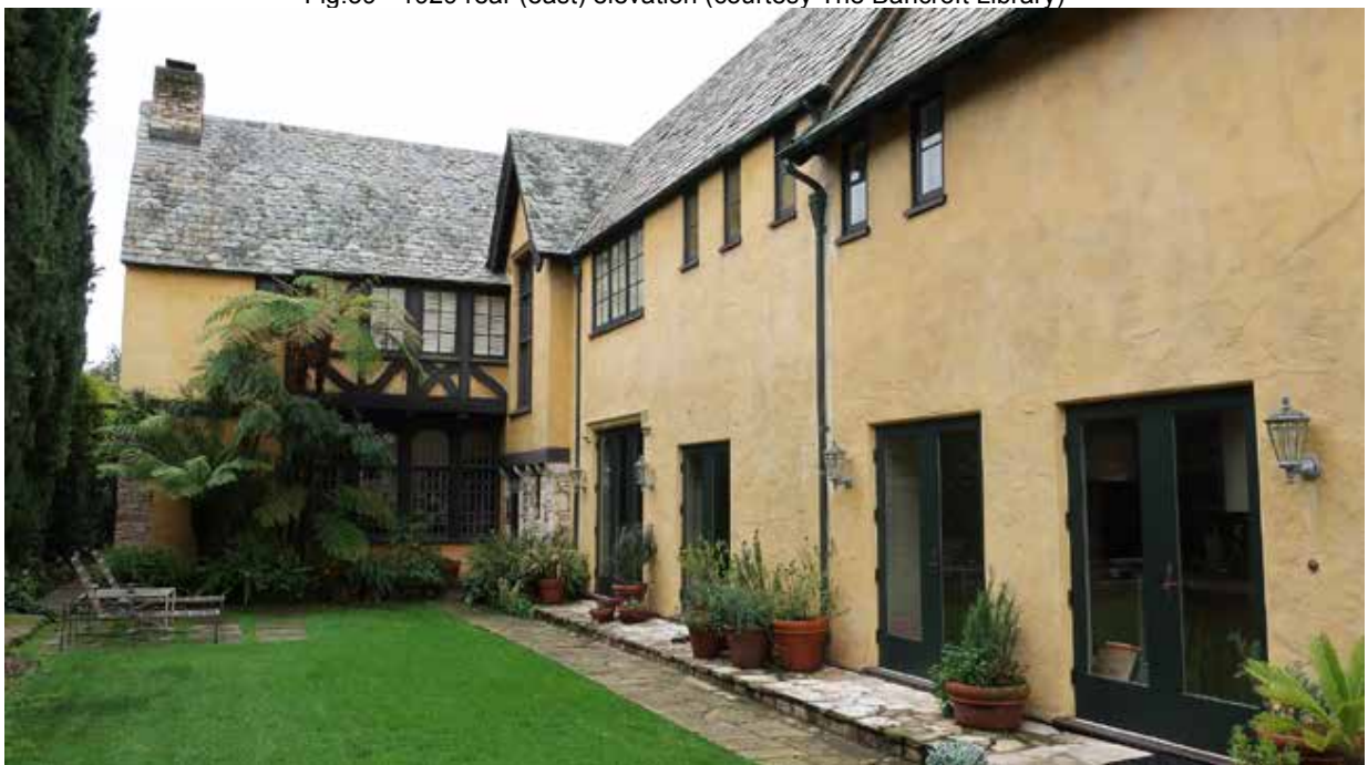
Fig.40 – Rear (northern side)
