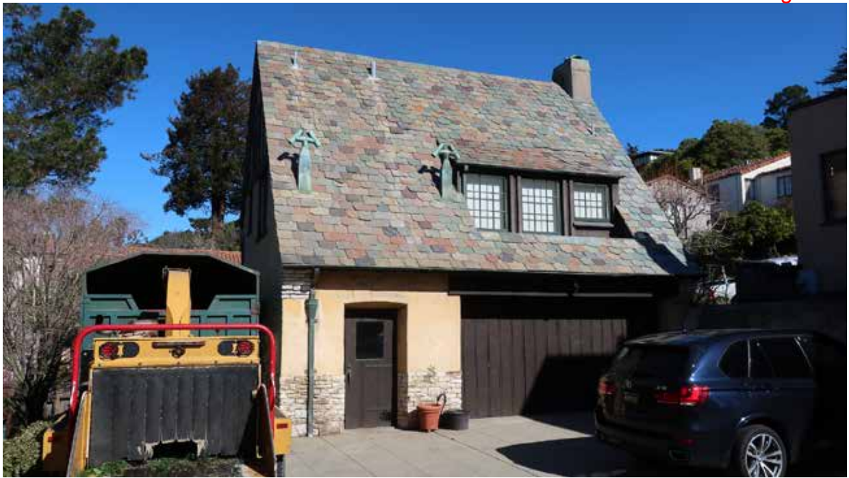
Fig.50 - Carriage house rear (south)
