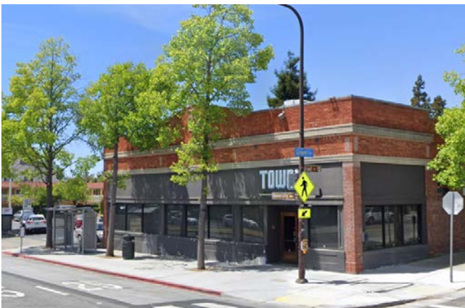
Figure 3.1. Bus Bulb at University Ave and Grant Street. (Source: Google)
