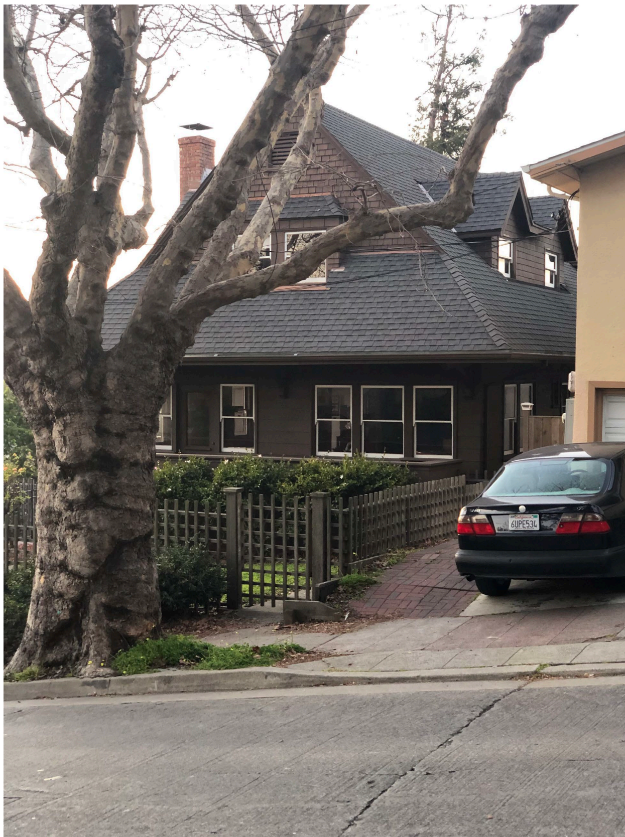
Fig.13 – 2119 Marin Ave. – Front and part east side
