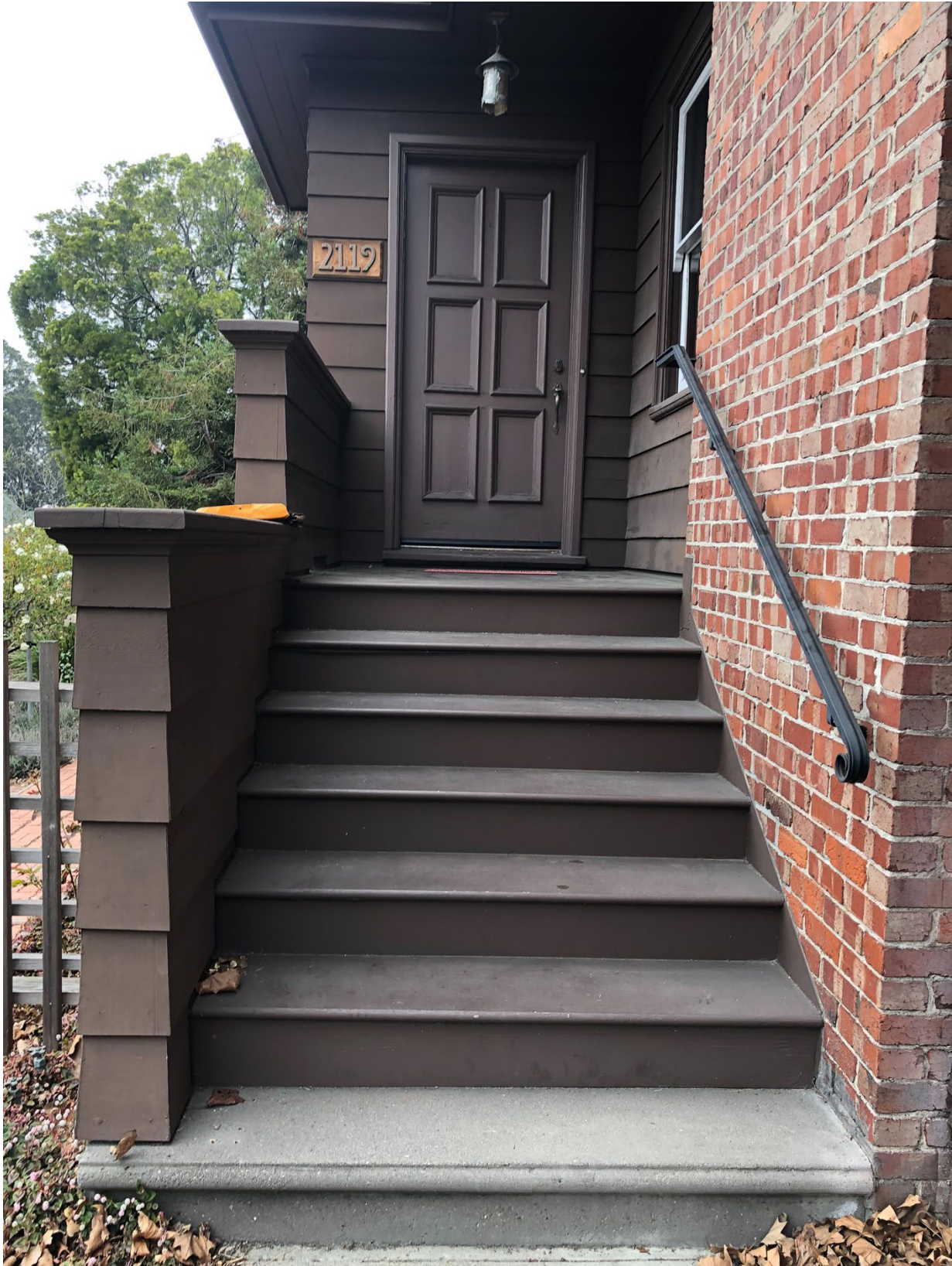
Fig.17 – 2119 Marin Ave. – West side entry
