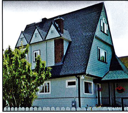
Fig.19. The earliest known true High-Peaked Colonial Revival house, at 2354 East 23rd Street in Oakland, designed by Hugo Storch in 1895. Google Street View.
