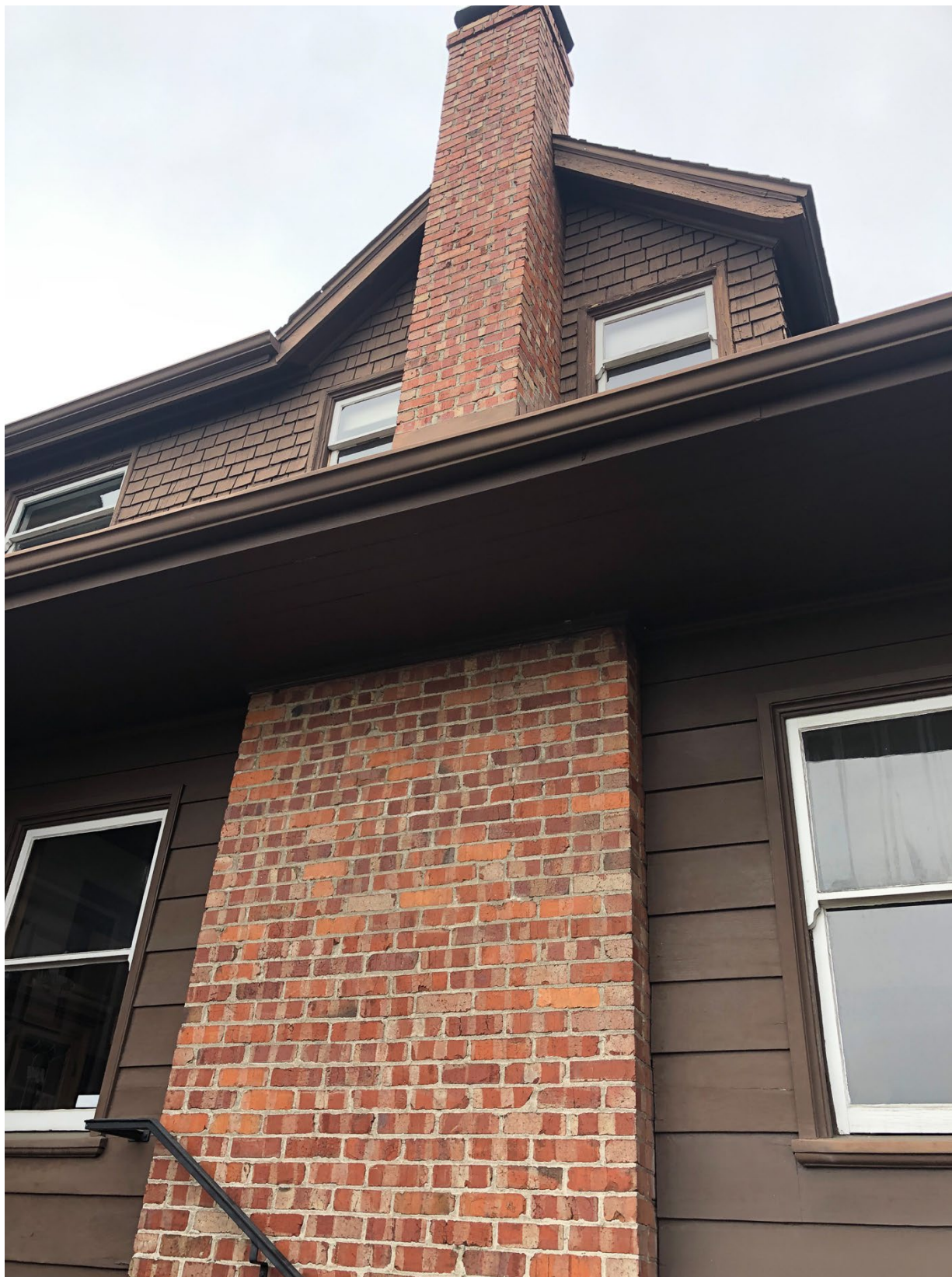
Fig.21 – 2119 Marin Ave. – Chimney at west side
