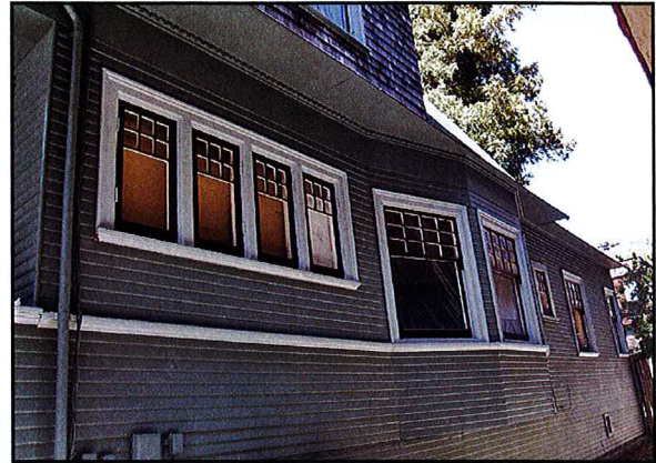
Fig. 10. South façade, looking east. Daniella Thompson, 2021
