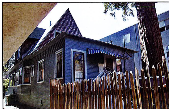
Fig. 3. The one-story extension of the ground floor at the rear. Daniella Thompson, 2021
