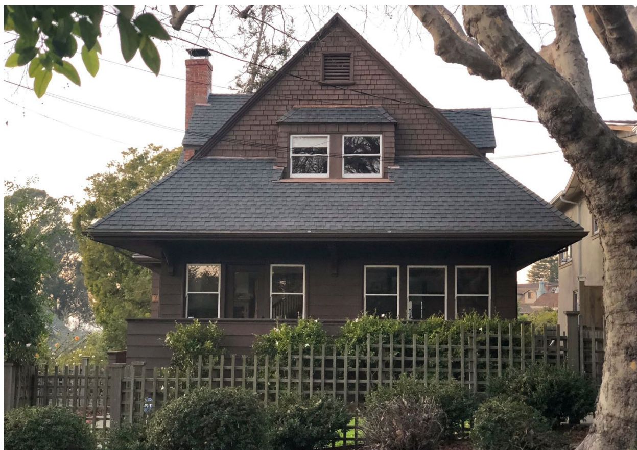
Fig.11 – 2119 Marin Ave. – Front of house from street (figs.11-24, MH 2022)
