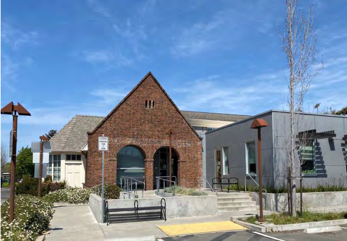
Corporation Yard Building
