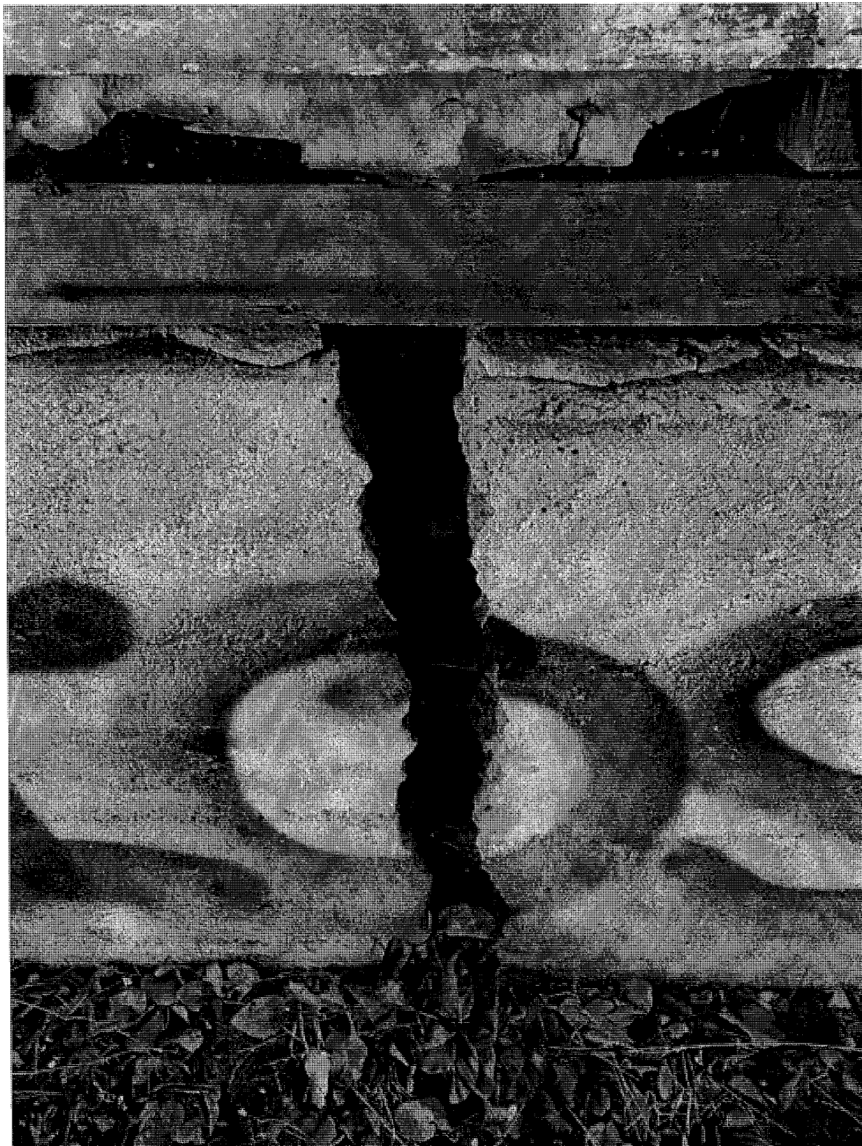
Fig.9 – 639 Arlington Ave. – West side foundations
