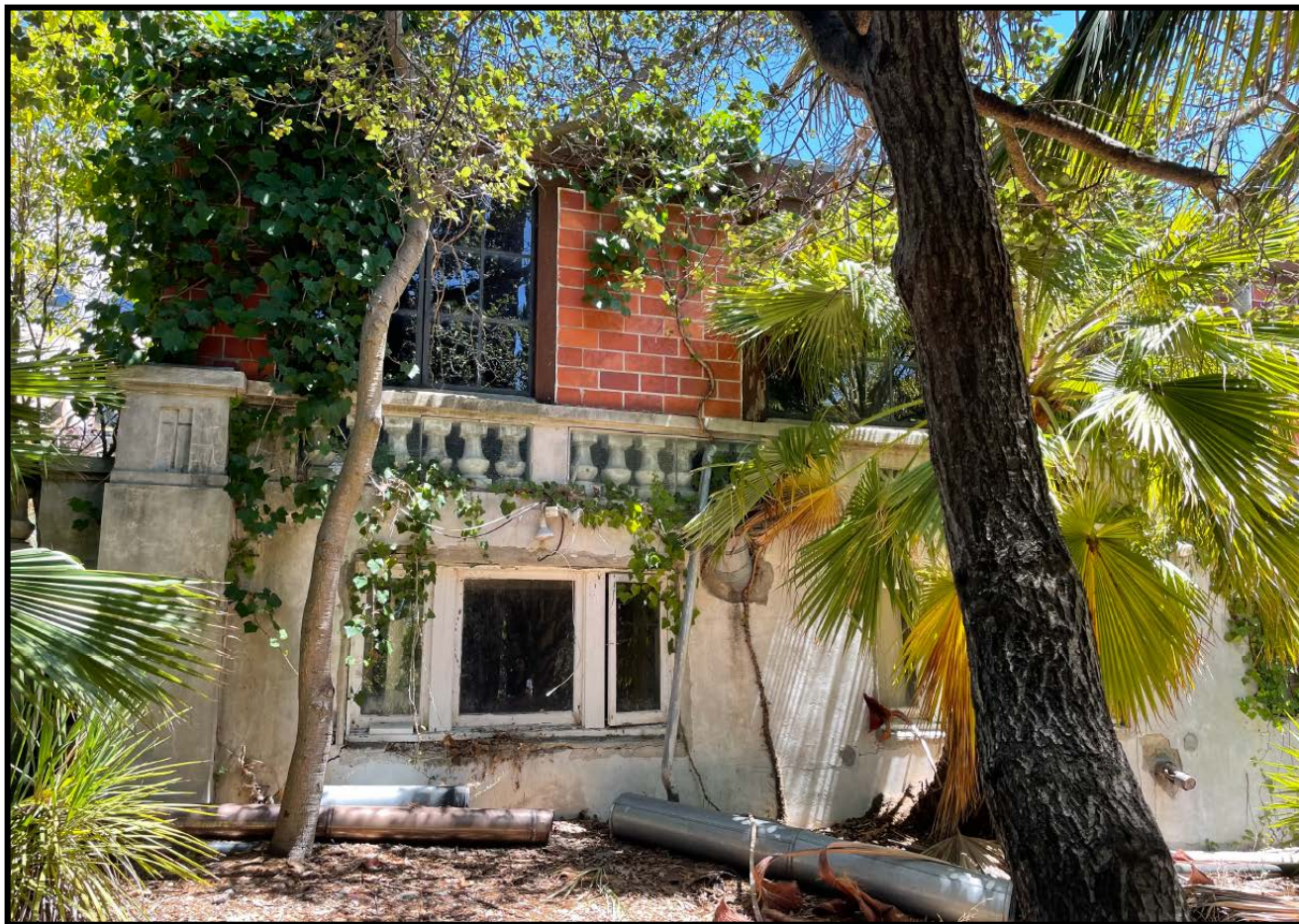
Figure 5: Subject property, west elevation of addition off west terrace. Upper level cafeteria/auditorium to be demolished to restore the southwest terrace. Game room below the terrace to be rehabilitated (2022).
