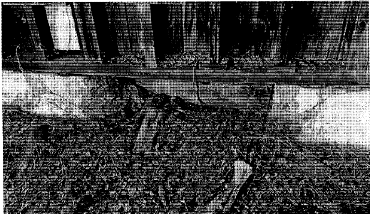
Fig.6 – 639 Arlington Ave. – West side foundations
