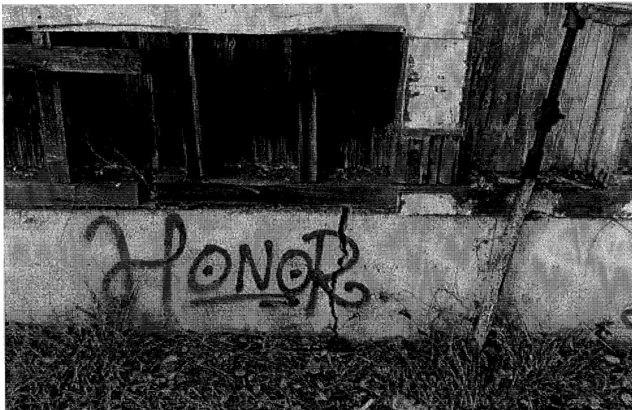
Fig.7 – 639 Arlington Ave. – West side foundations
