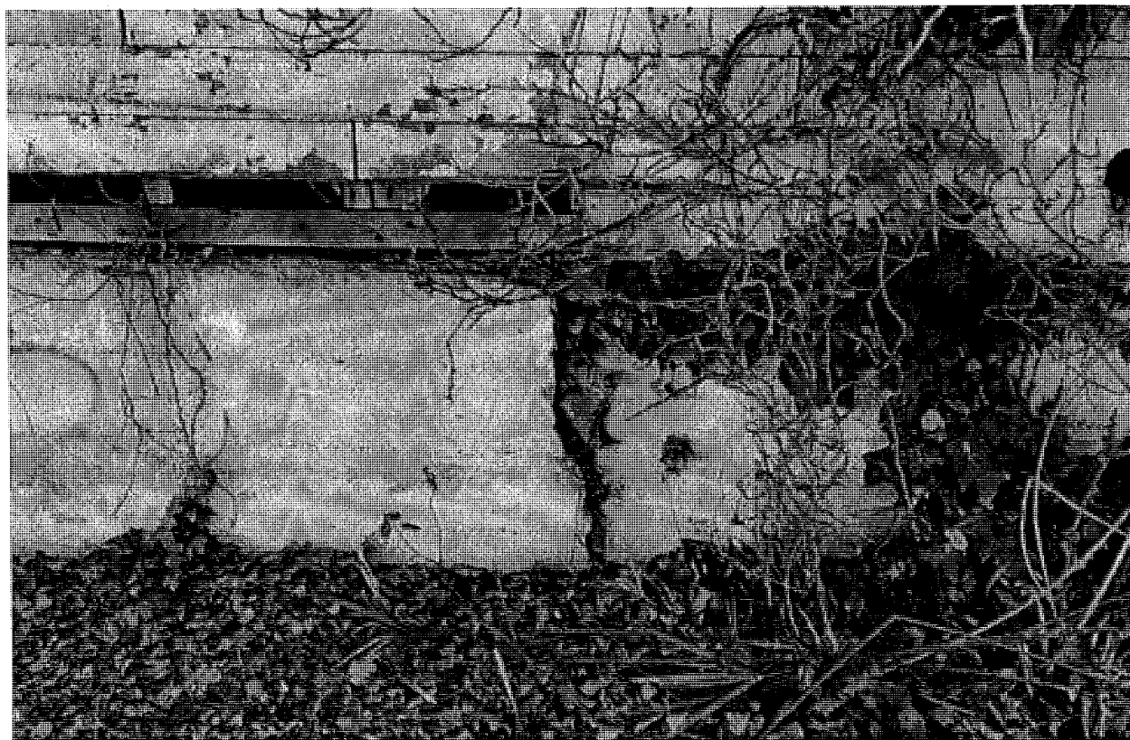
Fig.8 – 639 Arlington Ave. – West side foundations
