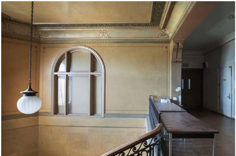
Central Stair at Second Floor
