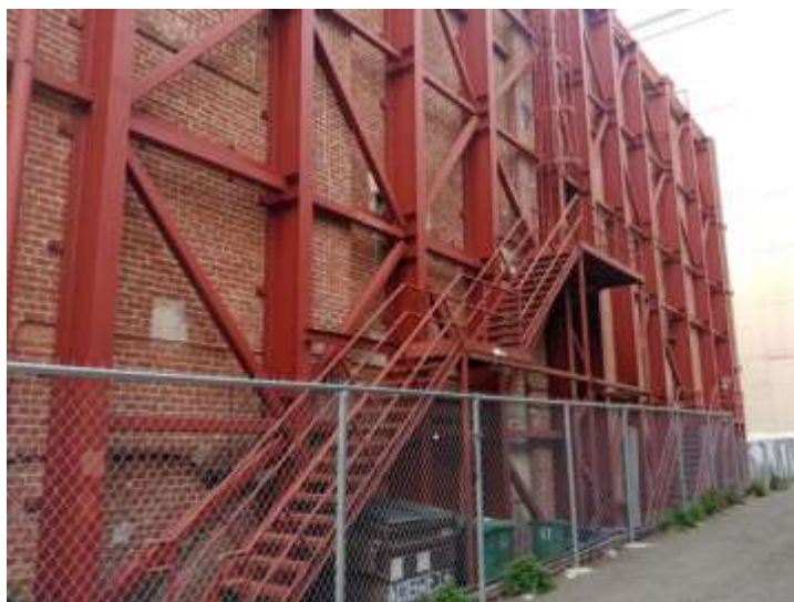
Figure 6. Side walls, right side, of the California Theatre, November, 2021. Photo: Therese Poletti
