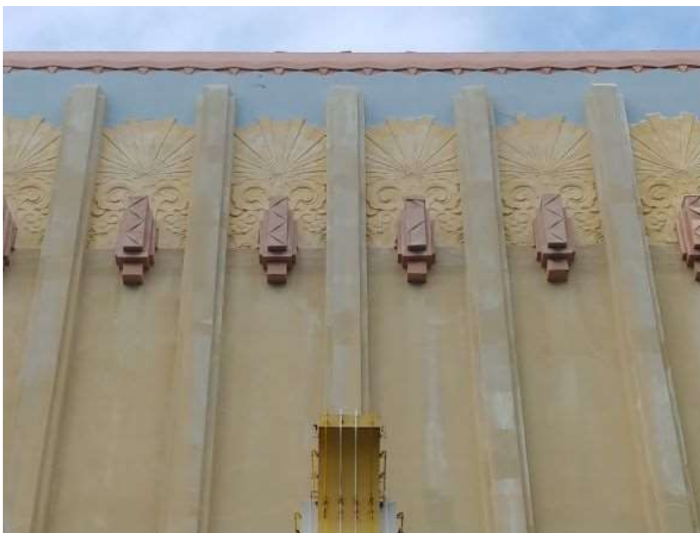
Figure 4. Art Deco details on façade, including piers, rectangular corbels, and “frozen fountain” bas-reliefs, November 2021. Photo: Therese Poletti
