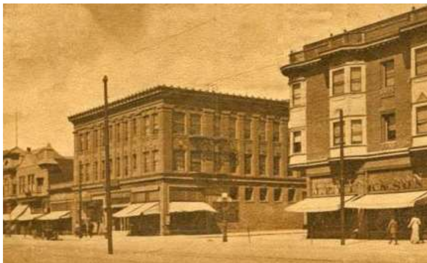
Figure 36. Postcard circa 1907, showing corner of Shattuck and Kittredge, with Brooks Apartments (left) and Wanger Block (right), courtesy Daniella Thompson
