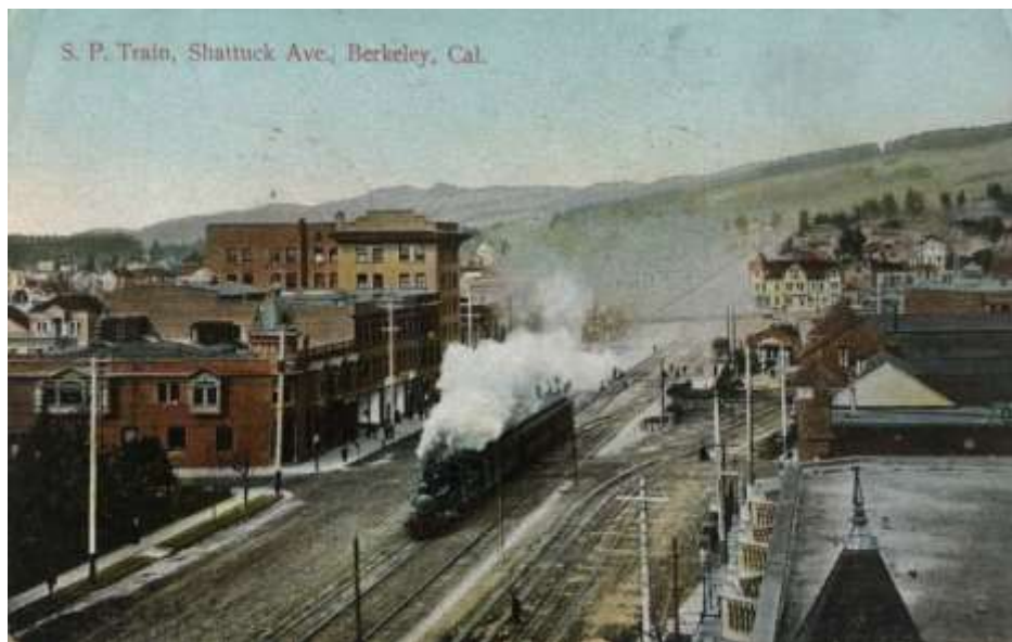
Figure 9. Southern Pacific station on Shattuck Avenue, circa 1909
