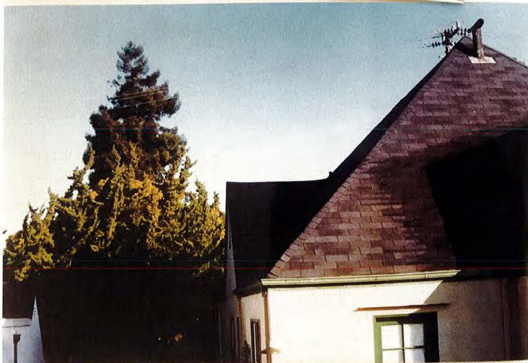
1710 SONOMA AVE. BEFORE ADDITION
