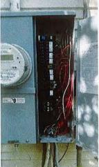
Item 002 - Electrical Service Panel - Visible Signs of Damaged Wiring
