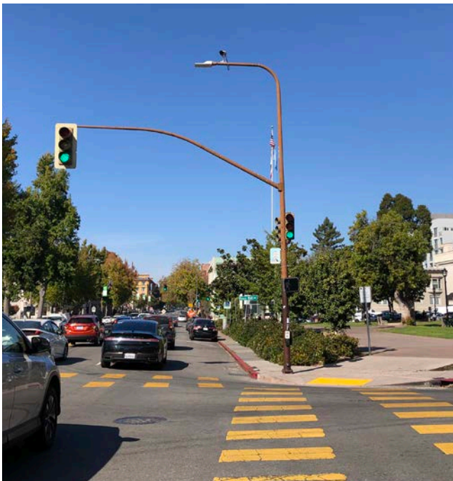
View at MLK Jr. Way & Allston Way Intersection looking North
