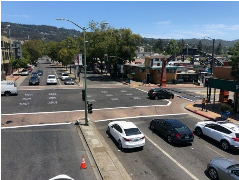
Botts' dots installed at an intersection to deter sideshows.
