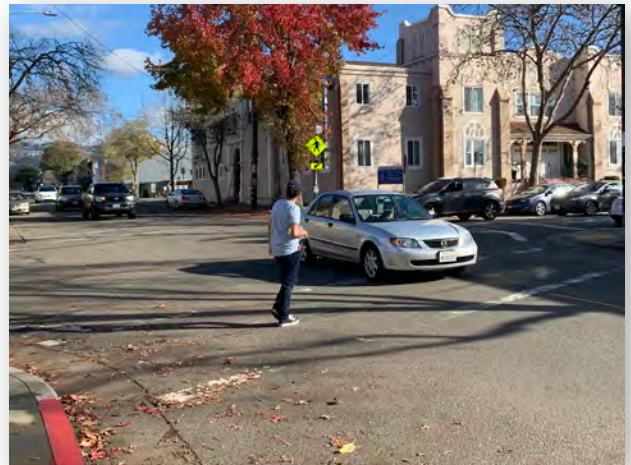
Alcatraz Avenue at King Street. Faded crosswalk markings decrease pedestrian visibility and awareness.
