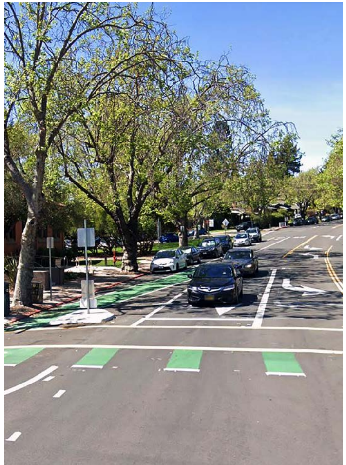
Protected intersection at The Alameda and Hopkins Street
