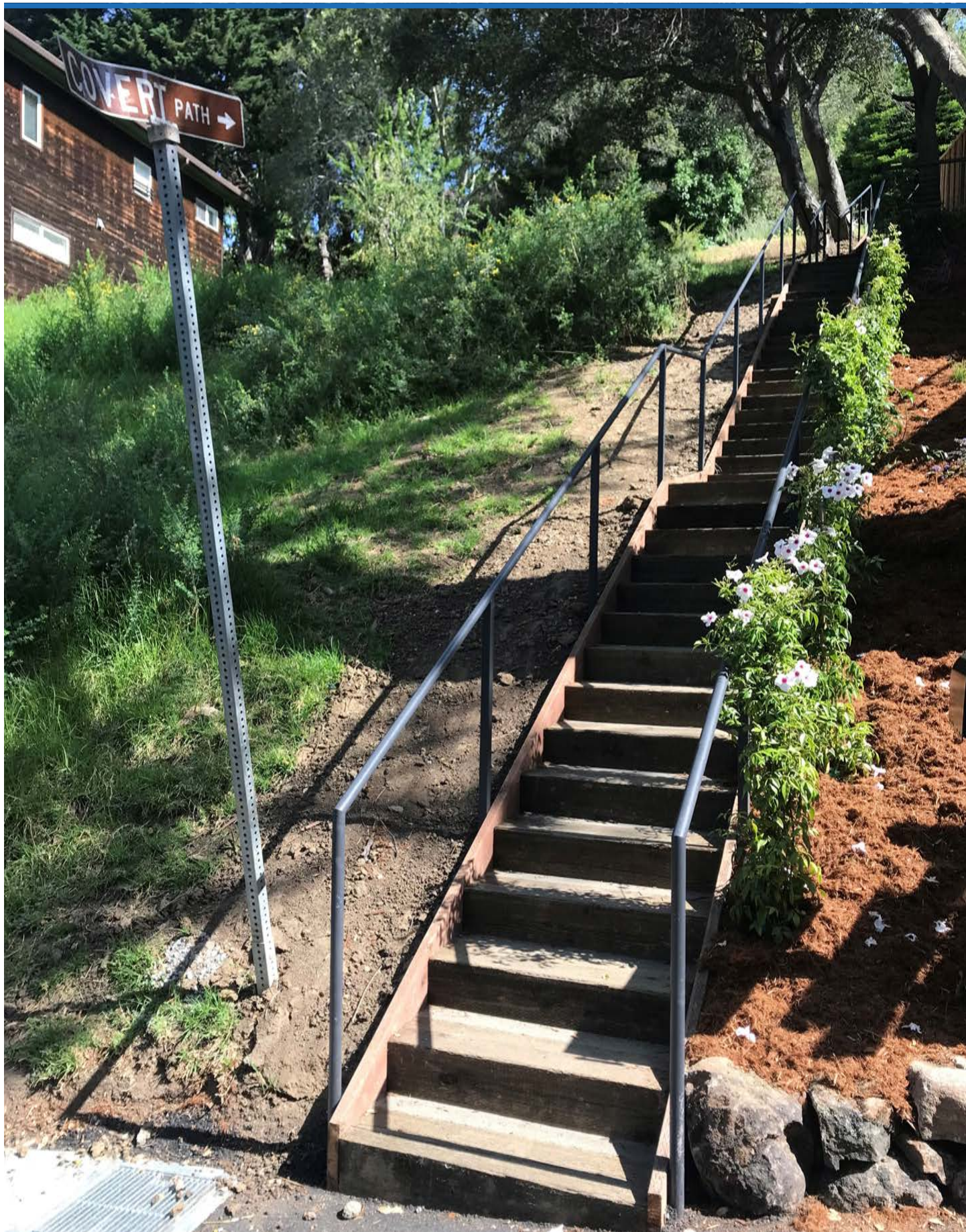
Covert Path provides a connection between Keith Avenue, Cragmont Avenue, and Keeler Avenue in the North Berkeley Hills. Photo: Amanda Leahy, Kittelson.
