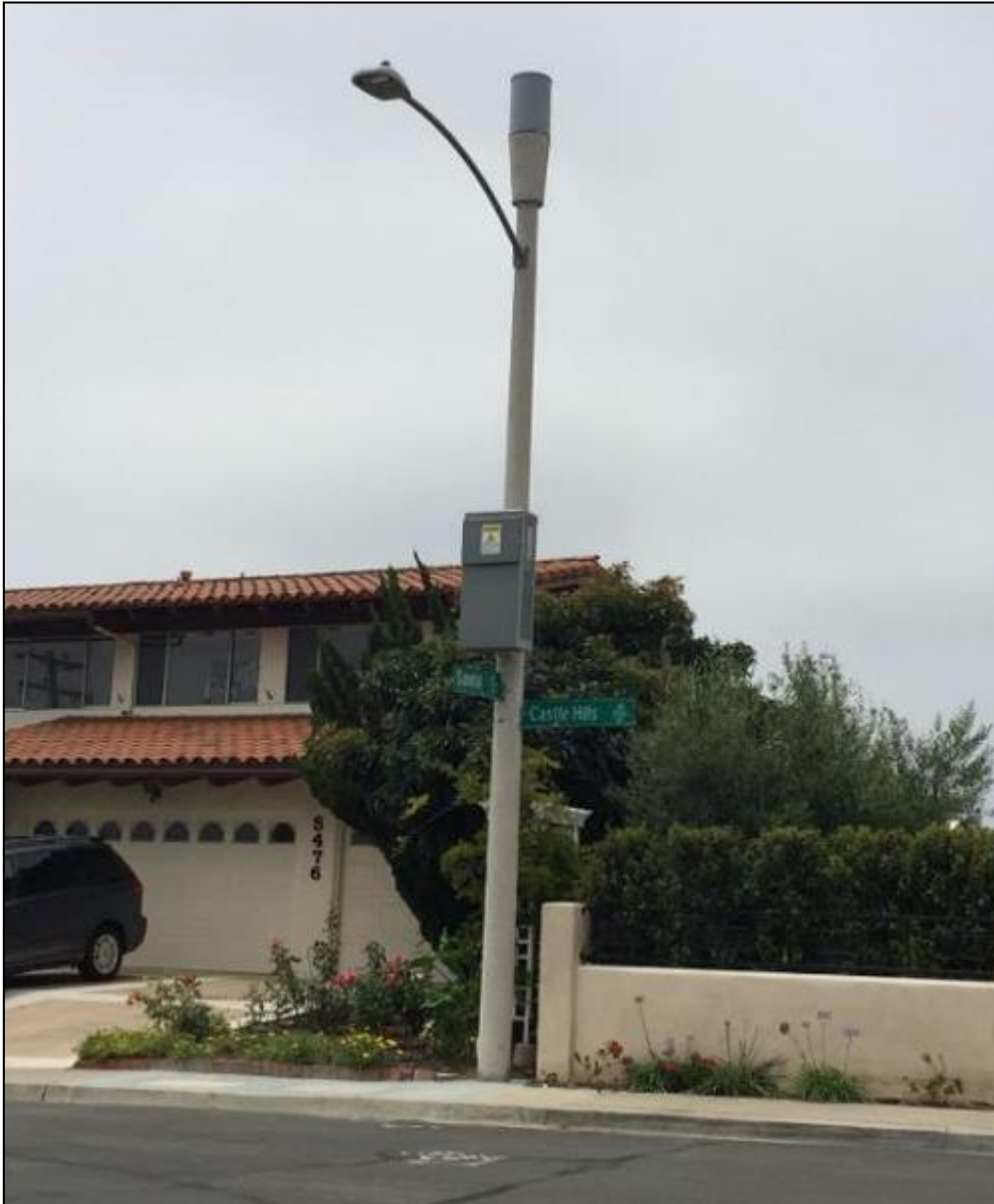
Figure 1: Antenna concealed within a single shroud (or radome) with a tapered cable shroud between the antenna and pole-top
