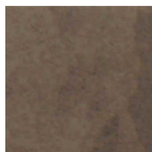
INTEGRAL COLOR STUCCO STEEL HARD TROWEL FINISH
