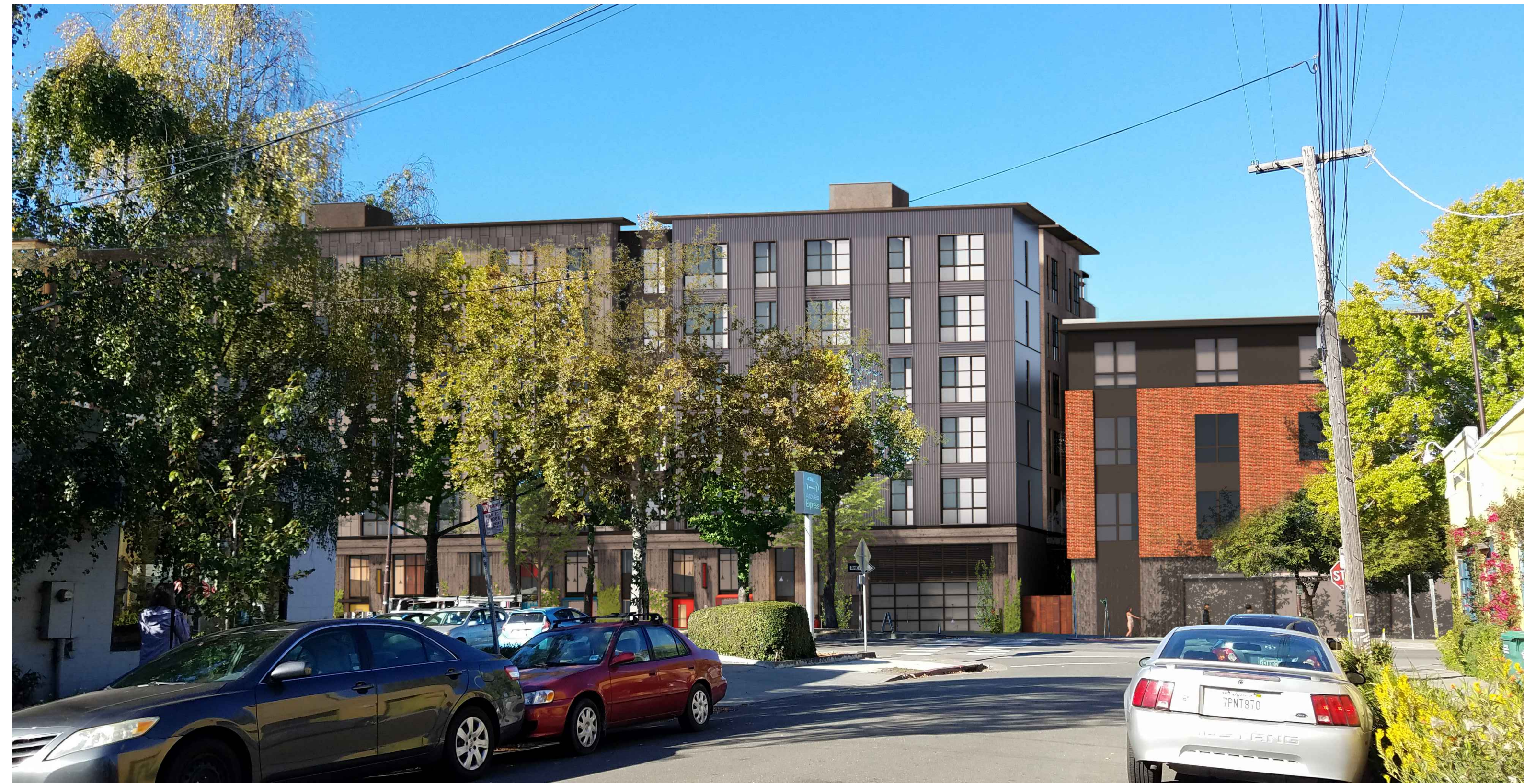
2 COWPER LOOKING WEST - AFTER
