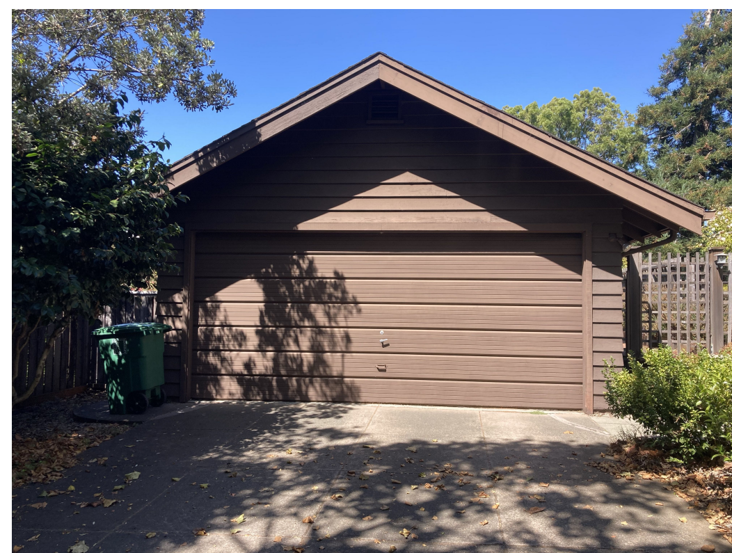
6. EXISTING GARAGE PHOTO - SOUTH ELEVATION
