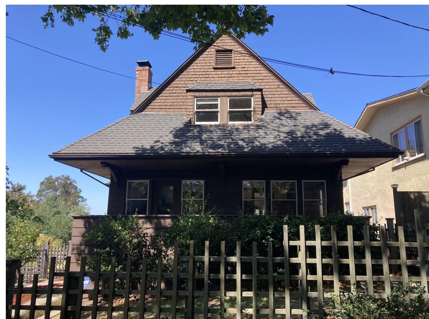
2. EXISTING HOUSE PHOTO - SOUTH ELEVATION
