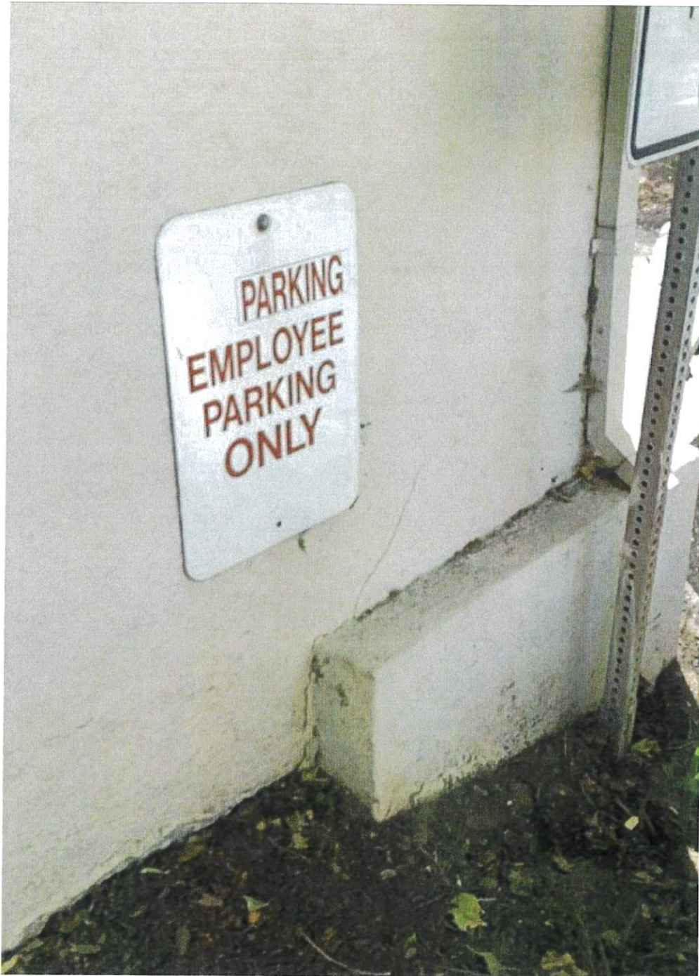
Photo 2 – Crack in Exterior Wall
