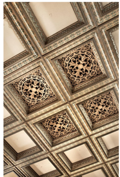
Veterans Memorial Building Ceiling
