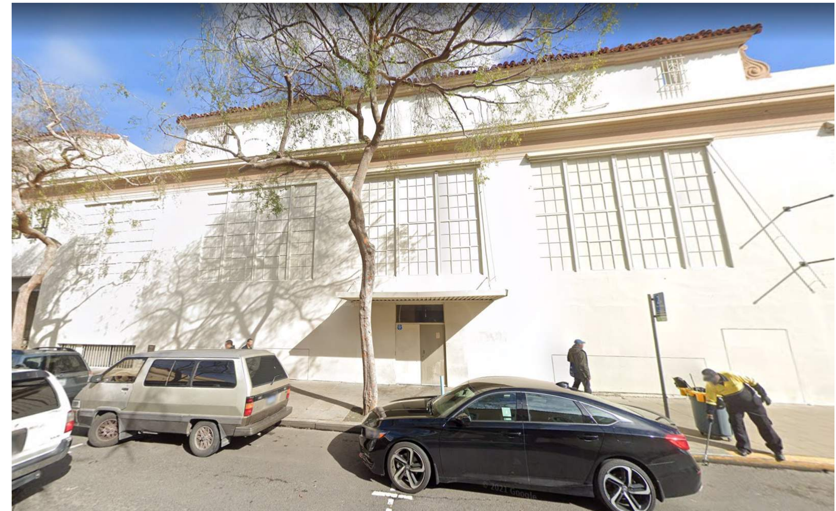
3 SITE PHOTO - HAROLD WAY SOUTH FACADE A0-002 12" = 1'-0"
