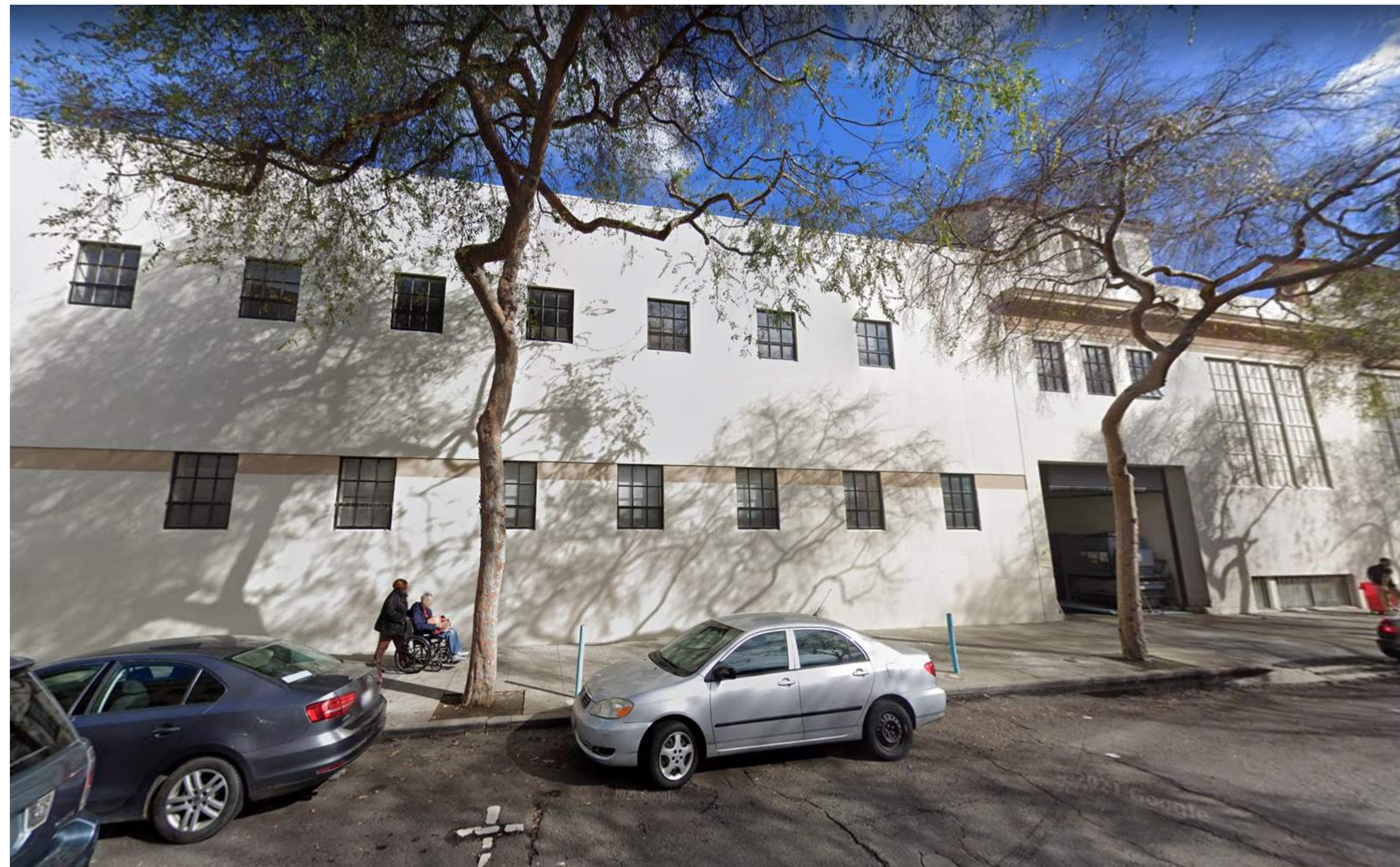
2 SITE PHOTO - HAROLD WAY NORTH FACADE A0-002 12" = 1'-0"
