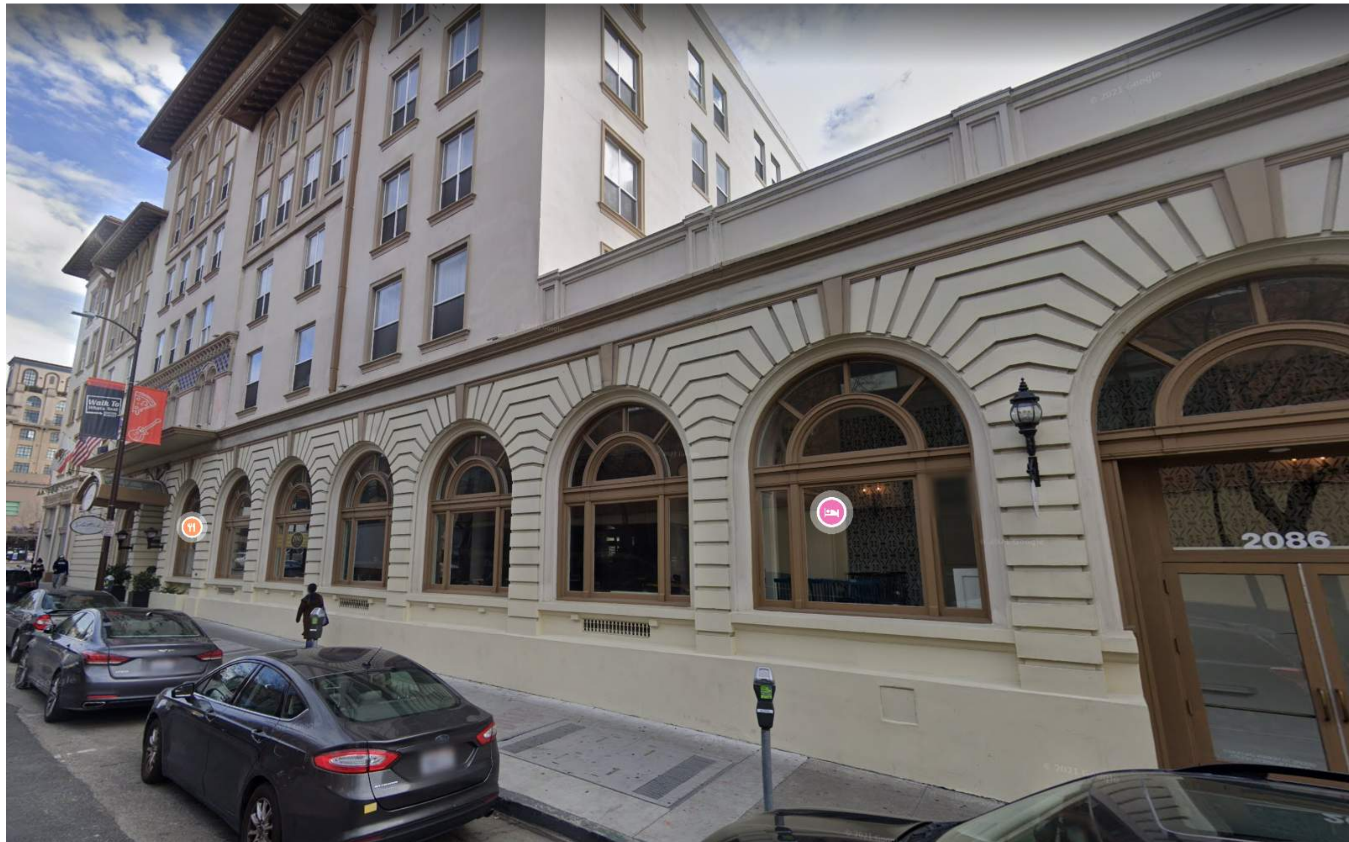
1 SITE PHOTO - ALLSTON WAY - EXISTING HOTEL A0-003 12" = 1'-0"
