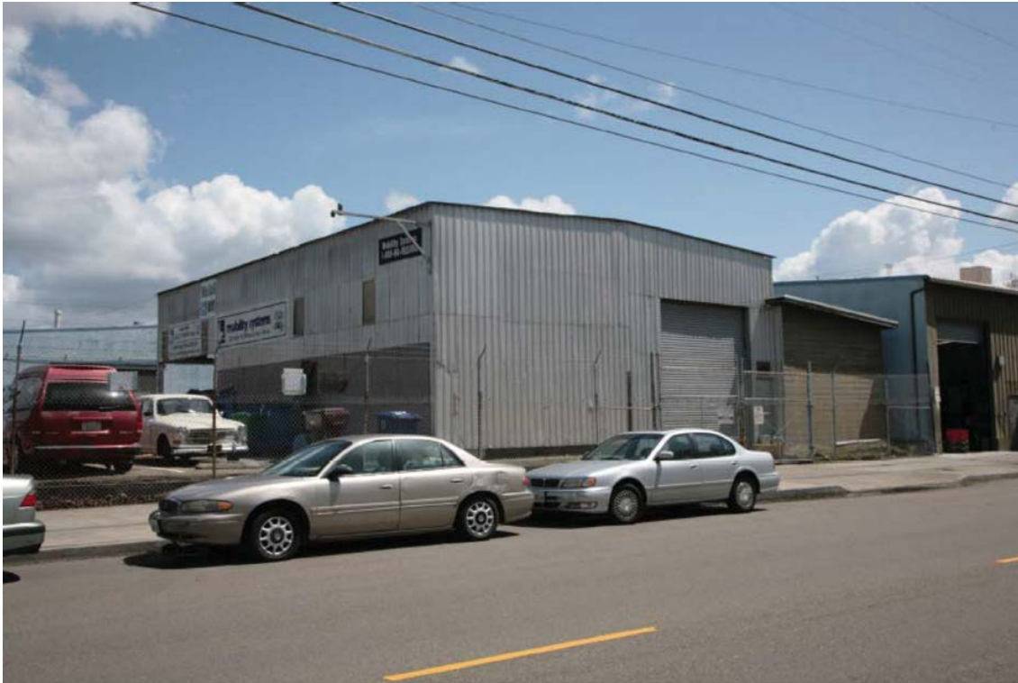
Photo 3: Storage shed, looking east. (Shayne Watson, 2018)
