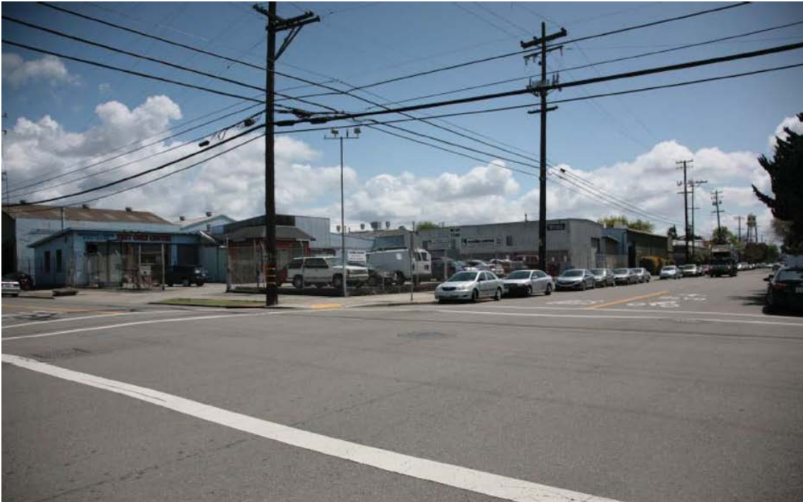
Photo 1: 1000-1010 Carleton Street, looking southeast. Original repair shop is at left. Storage shed at right. (Shayne Watson, 2018)
