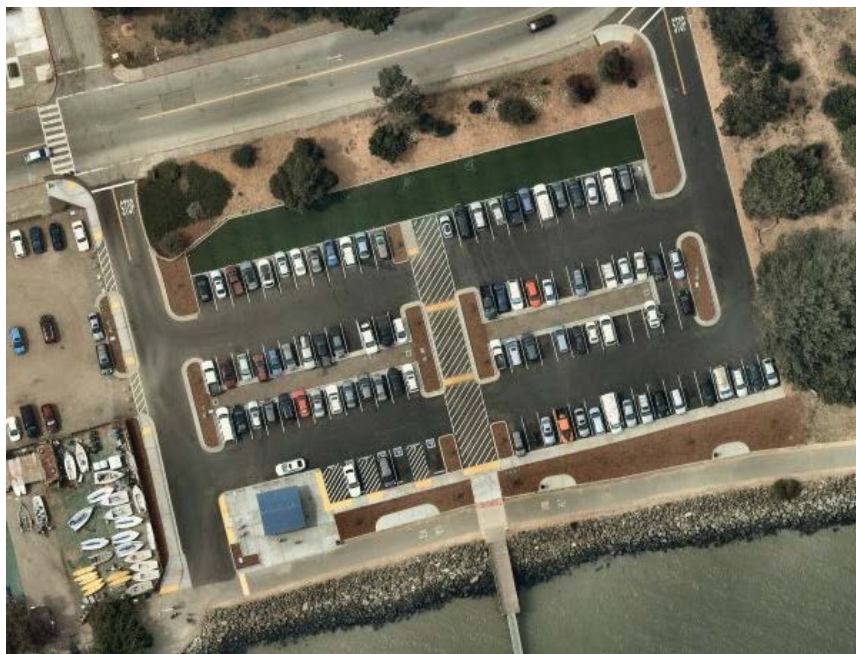
Figure 2 Aerial of South Cove East Lot after Reconstruction (July 7th, 2018) 11
