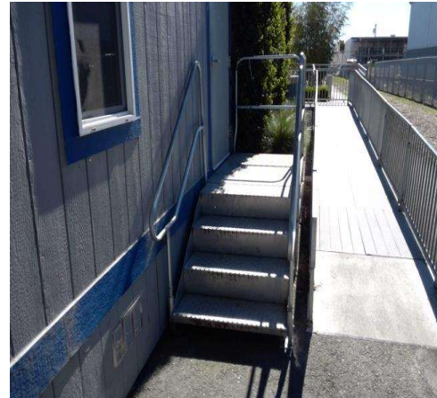
Stairway , Handrail : Handrail Bottom Extension
