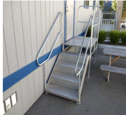
Stairway , Handrail : Handrail Bottom Extension
