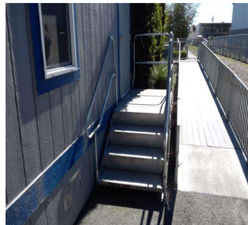
Stairway , Handrails : Handrail Extension Length
