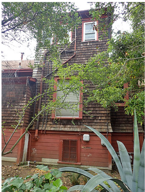
Figure 27. East façade, central section
