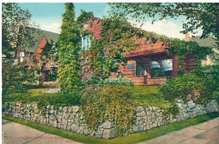
Figure 59. First Unitarian Church (A.C. Schweinfurth, architect, 1898)
