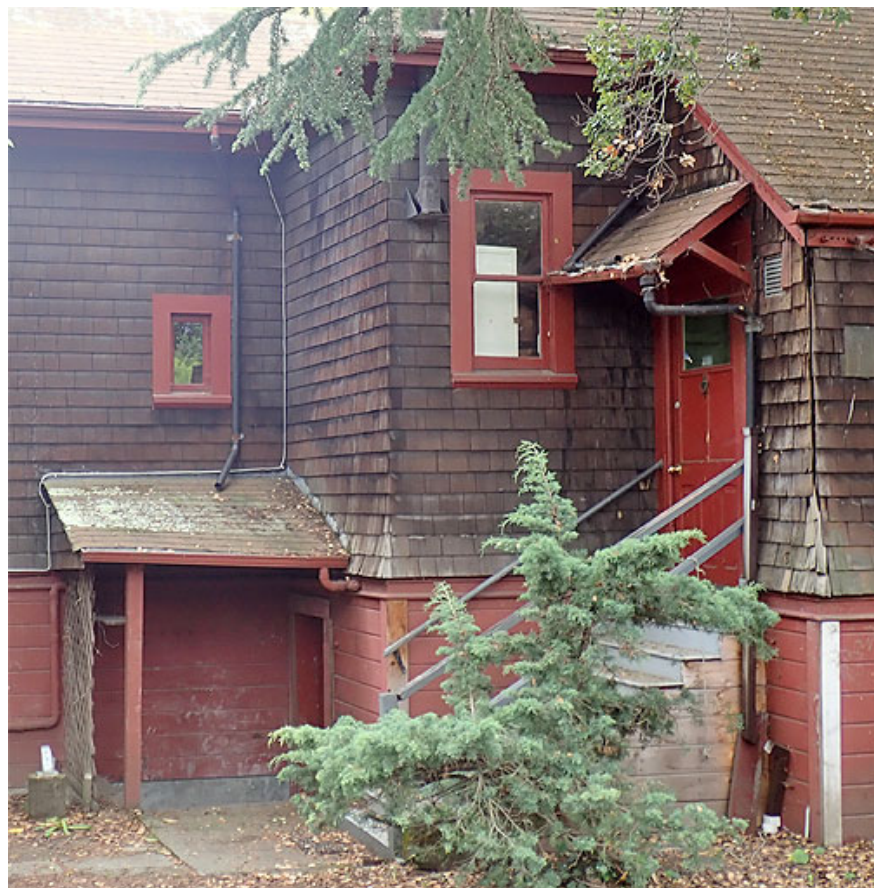
Figure 32. Cellar & service entrances
