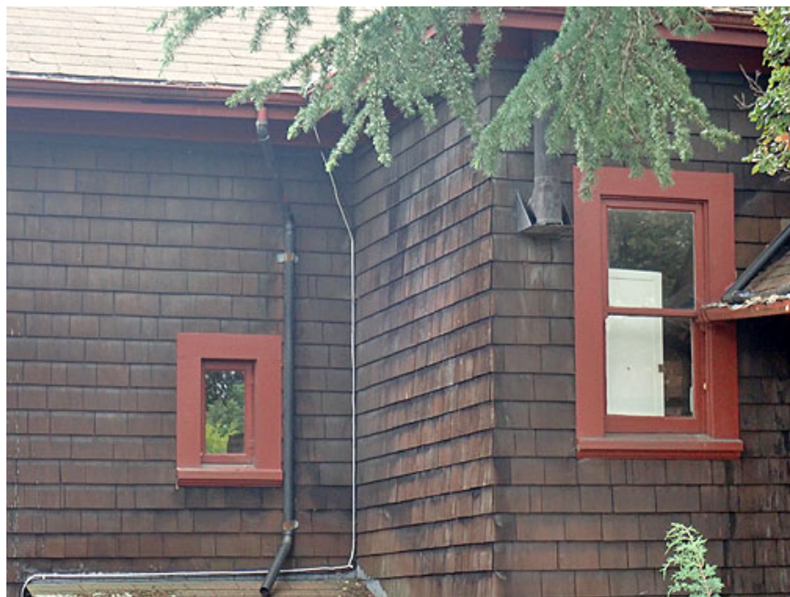
Figure 33. Windows, north façade
