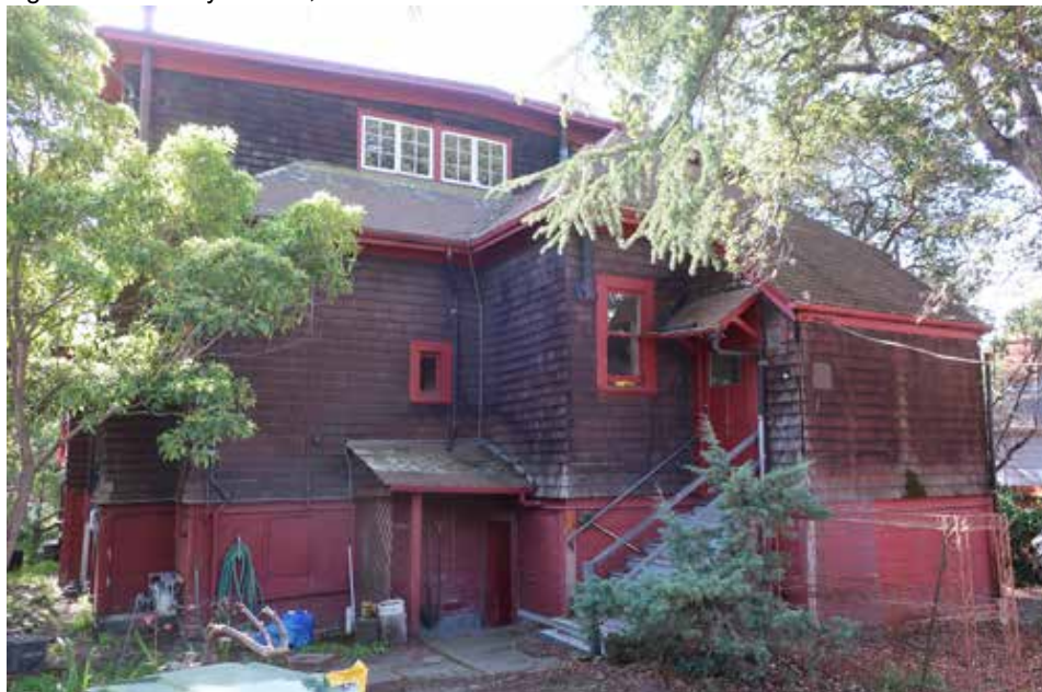
Fig.7 – 1915 Berryman St., rear (north) from rear driveway
