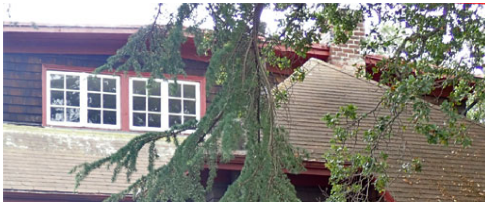
Figure 31. Brick chimney, north side
