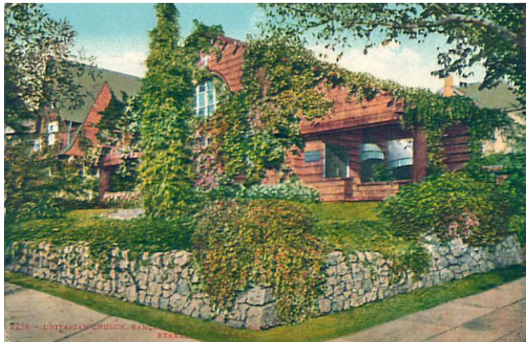
Figure 59. First Unitarian Church (A.C. Schweinfurth, architect, 1898)
