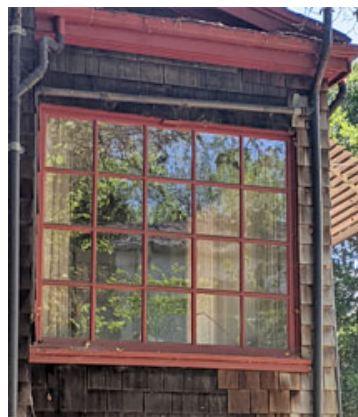
Figure 15. West-facing window in front porch
