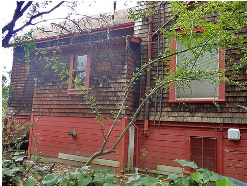
Figure 25. Circa 1940s addition, east façade
