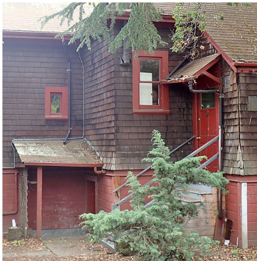
Figure 32. Cellar & service entrances
