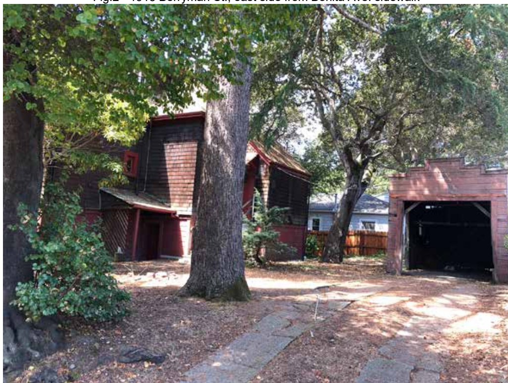
Fig.3 - 1915 Berryman St., rear from Bonita Ave. sidewalk
