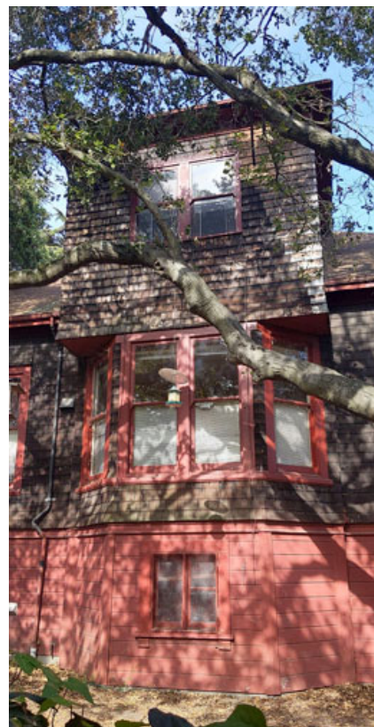
Figure 23. Bay window & second story, west façade
