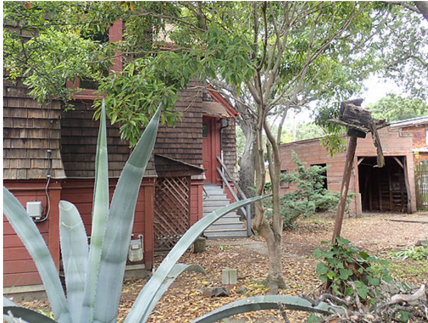
Figure 29. East façade toward the rear & garage
