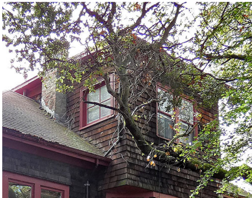
Figure 19. Upper story above west façade
