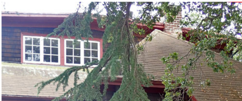
Figure 31. Brick chimney, north side
