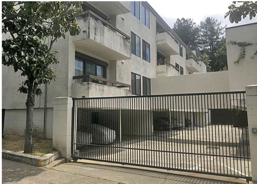
Figure 86. Raj Properties apartments, 1910 Berryman Street
