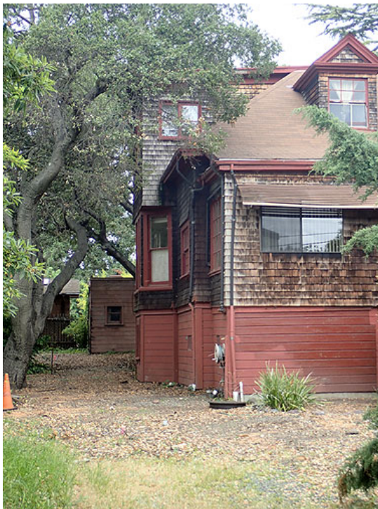
Figure 14. Enclosed porch, southwest corner
