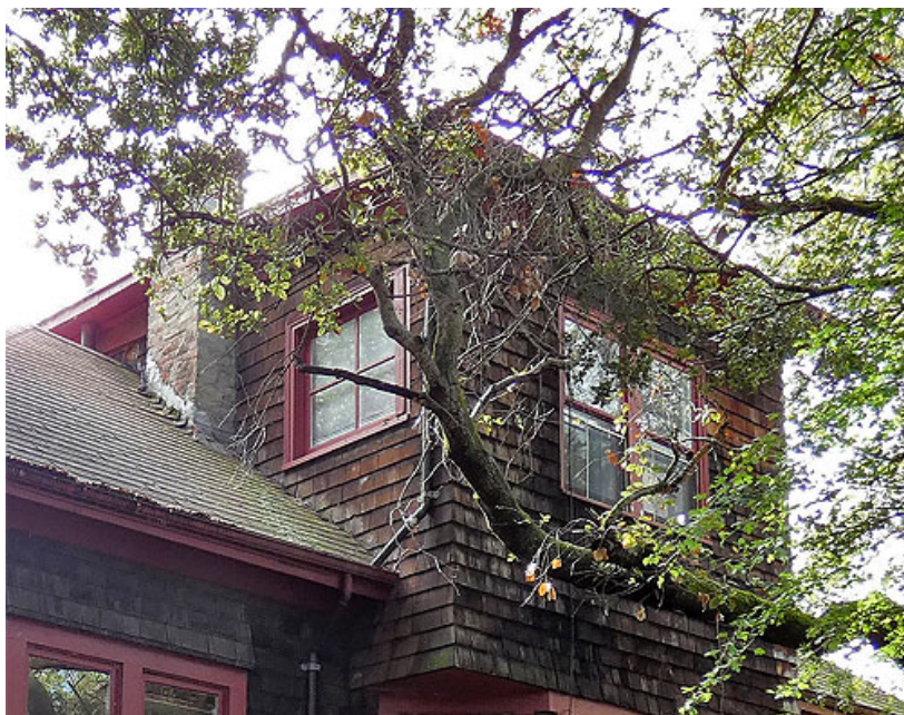
Figure 19. Upper story above west façade
