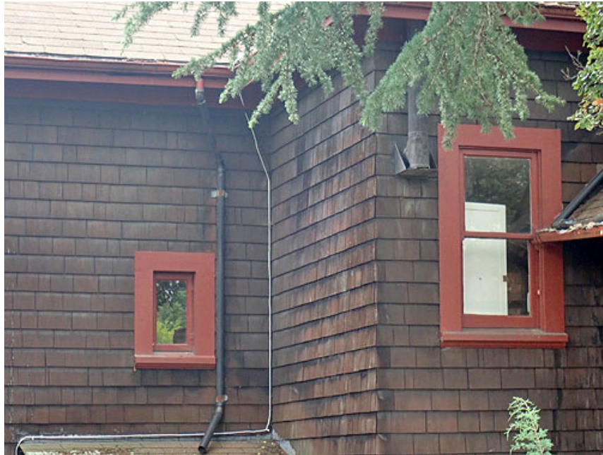
Figure 33. Windows, north façade
