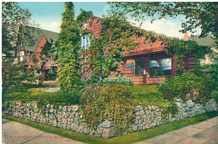
Figure 59. First Unitarian Church (A.C. Schweinfurth, architect, 1898)
