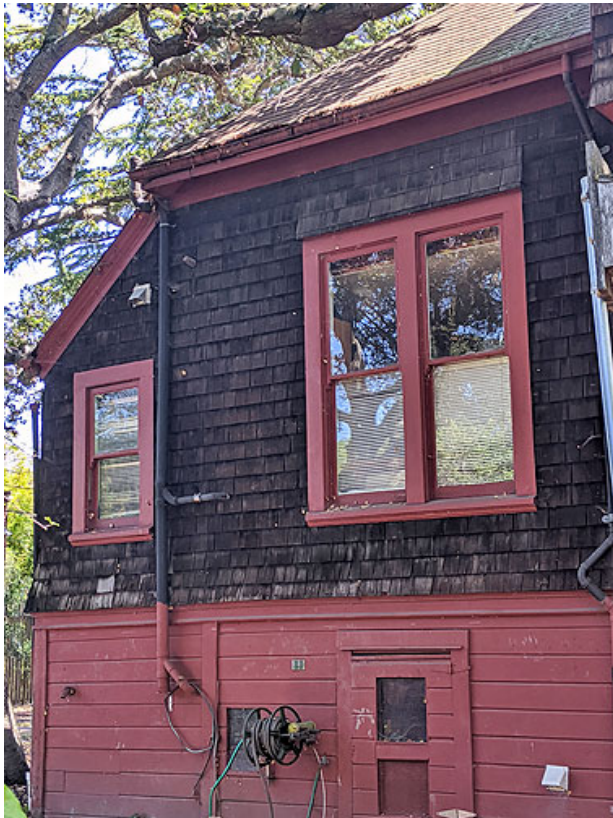
Figure 22. West façade toward the north
