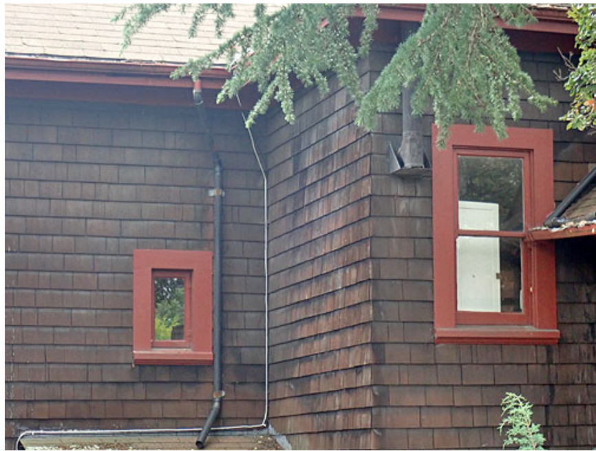
Figure 33. Windows, north façade
