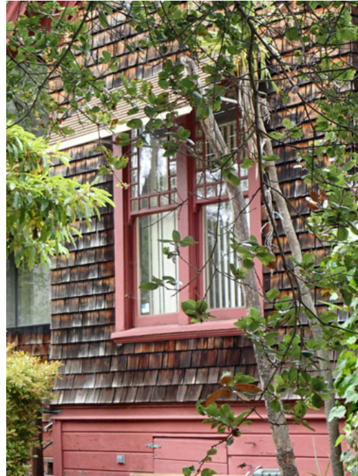
Figure 13. Windows in front wing
