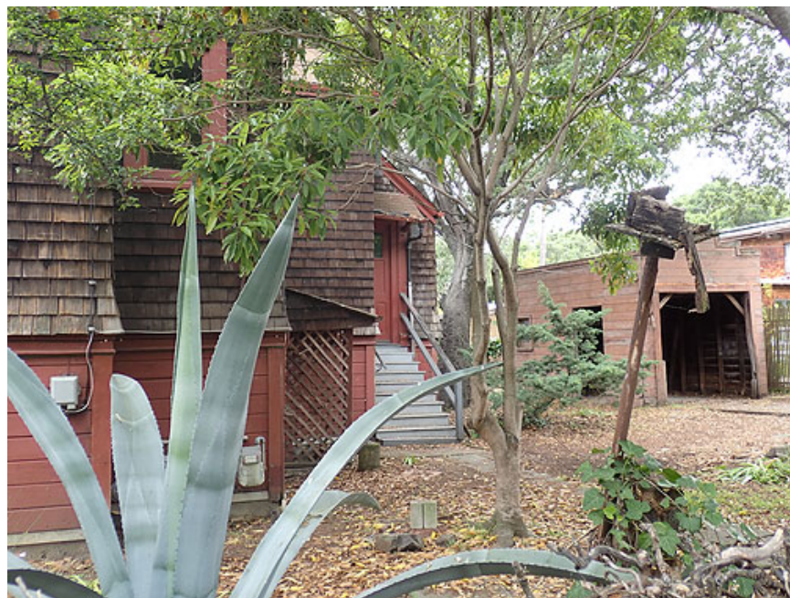
Figure 29. East façade toward the rear & garage
