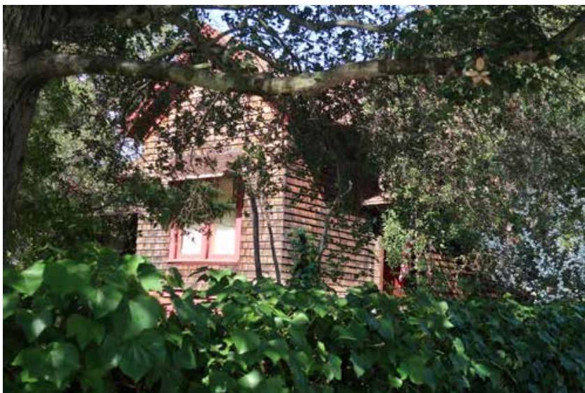
Fig.3 – 1915 Berryman St., view of house from Bonita Ave.
