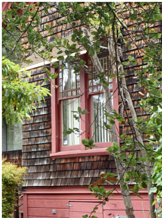
Figure 13. Windows in front wing
