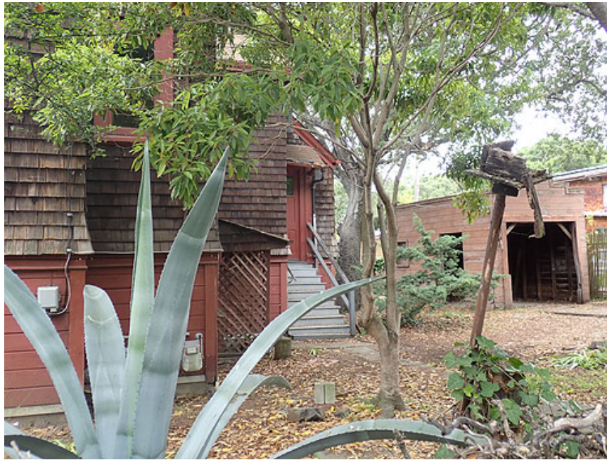
Figure 29. East façade toward the rear & garage
