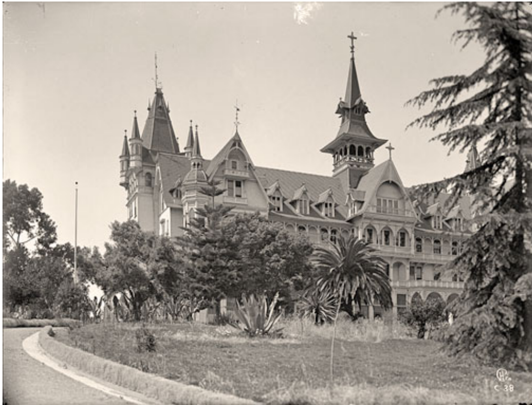
Figure 73. Peralta Park Hotel (Cheney Photo Advertising Agency)
