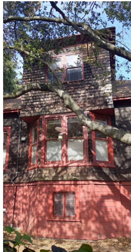
Figure 23. Bay window & second story, west façade
