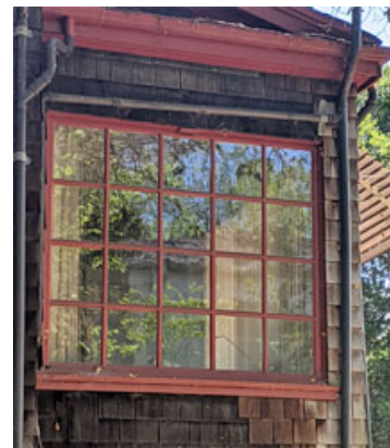
Figure 15. West-facing window in front porch
