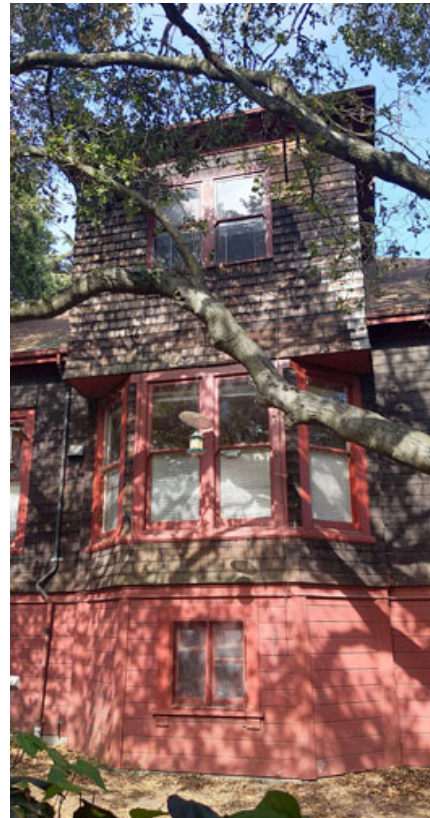
Figure 23. Bay window & second story, west façade
