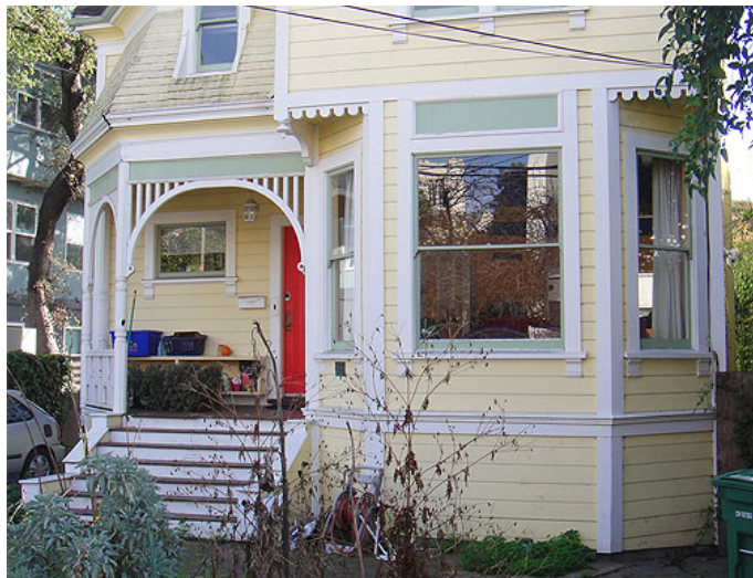
Figure 9. Rustic siding, Luttrell House
