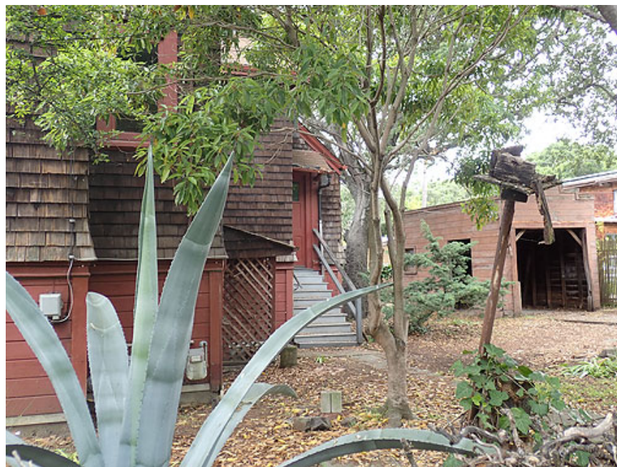
Figure 29. East façade toward the rear & garage
