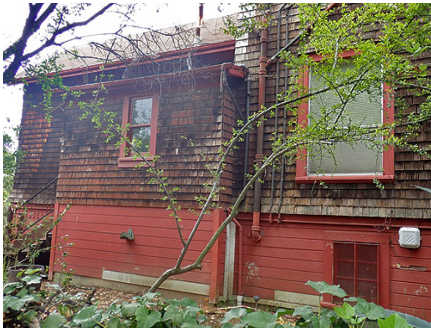
Figure 25. Circa 1940s addition, east façade
