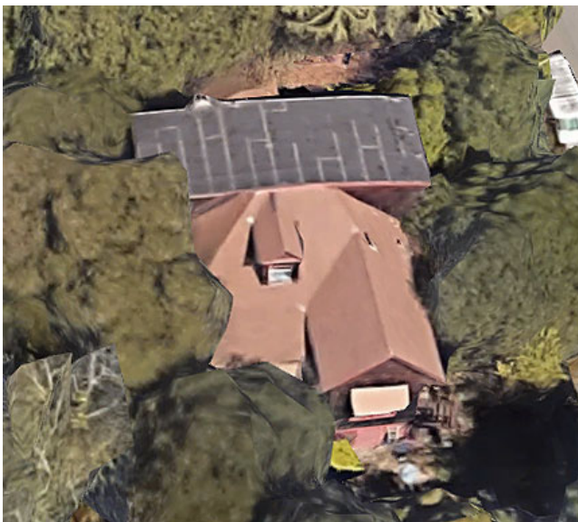
Figure 6. The 1889 hip roof, surmounted by the shallow-pitched roof built in 1925.
