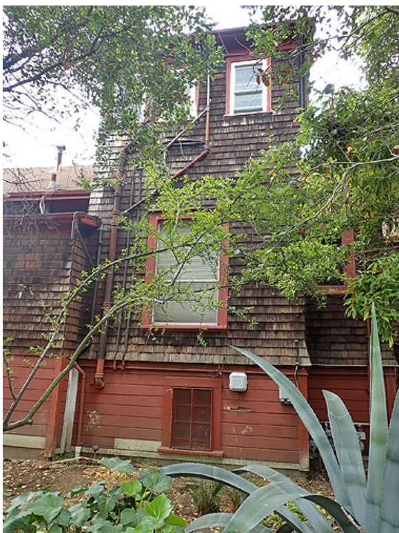
Figure 27. East façade, central section
