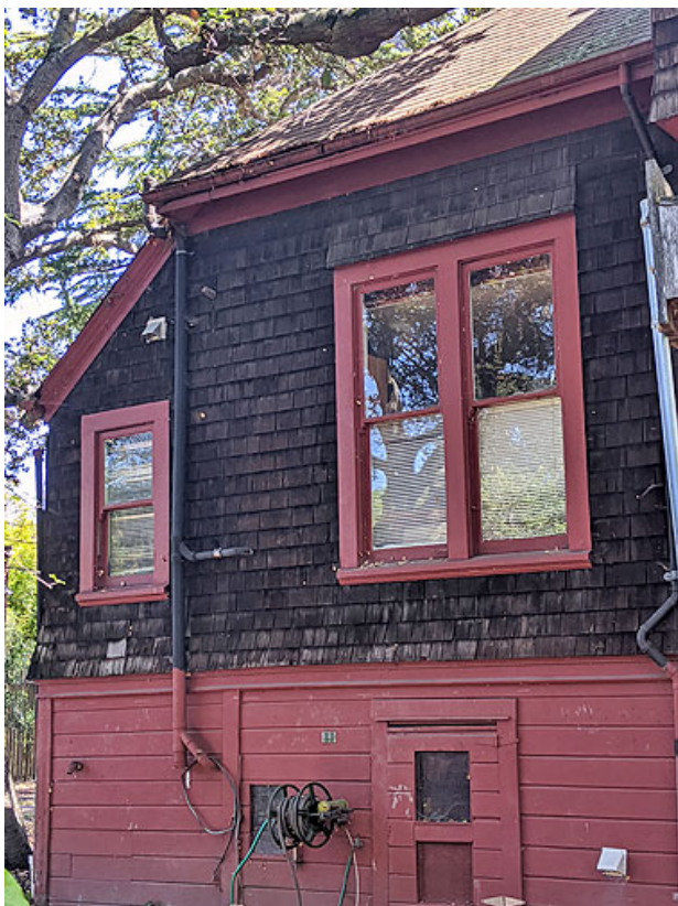
Figure 22. West façade toward the north
