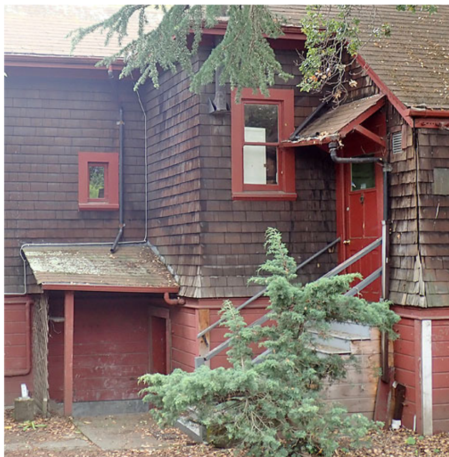
Figure 32. Cellar & service entrances
