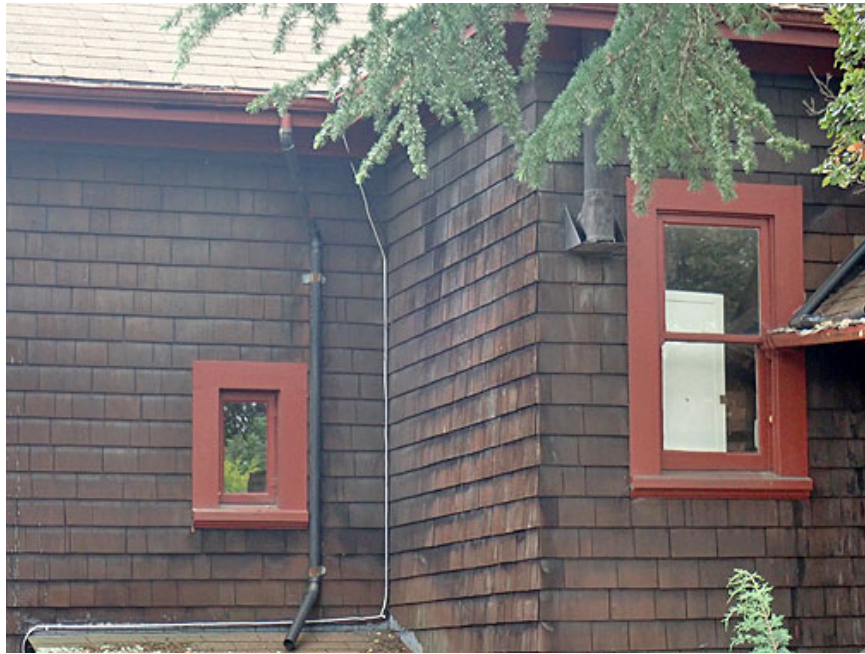
Figure 33. Windows, north façade
