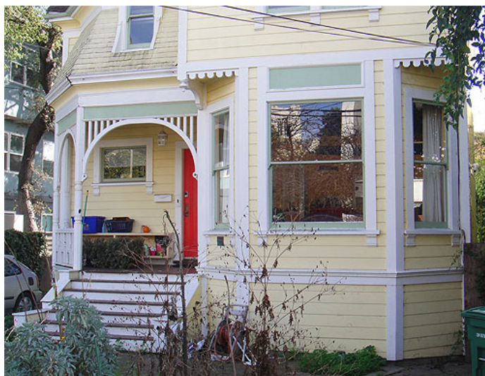
Figure 9. Rustic siding, Luttrell House
