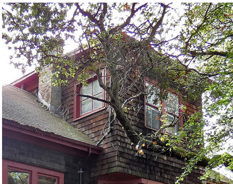
Figure 19. Upper story above west façade
