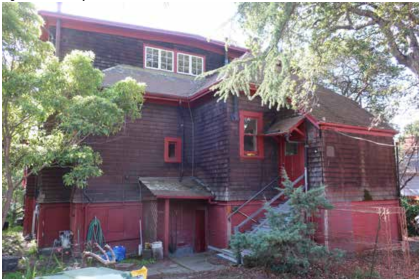
Fig.7 – 1915 Berryman St., rear (north) from rear driveway
