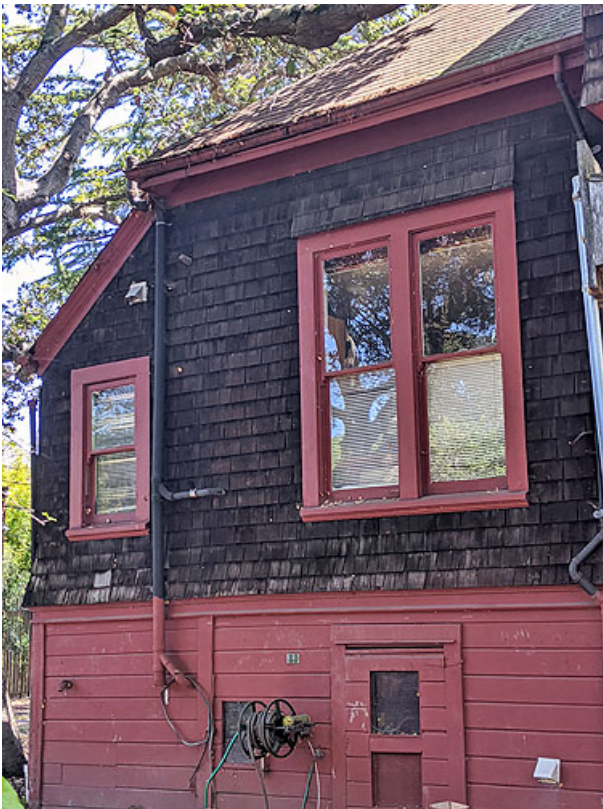
Figure 22. West façade toward the north
