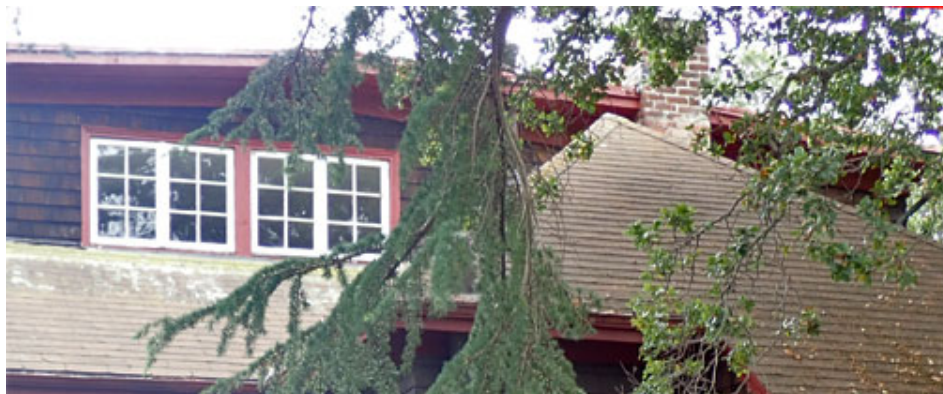
Figure 31. Brick chimney, north side
