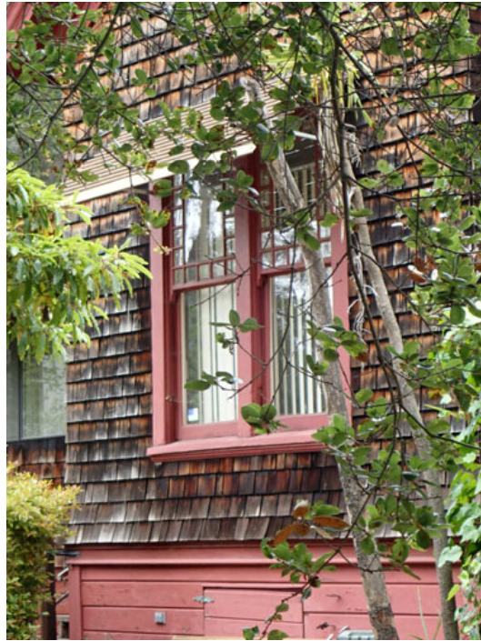
Figure 13. Windows in front wing
