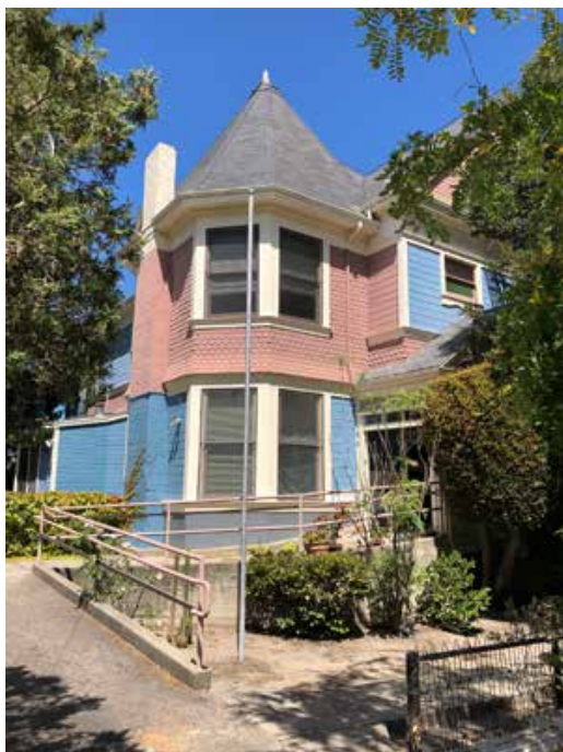
Fig.6 – 1410 Bonita Ave., c1892
