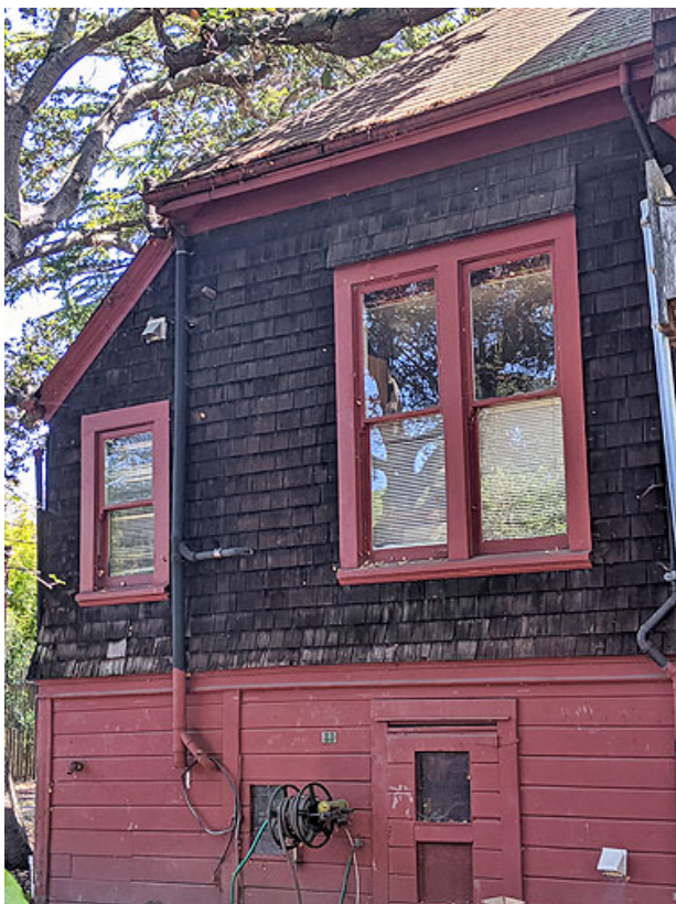
Figure 22. West façade toward the north
