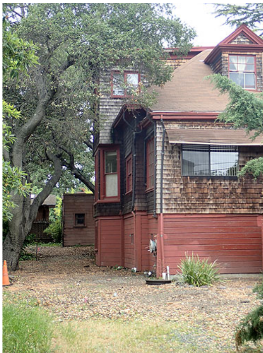
Figure 14. Enclosed porch, southwest corner
