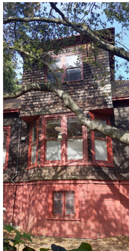
Figure 23. Bay window & second story, west façade
