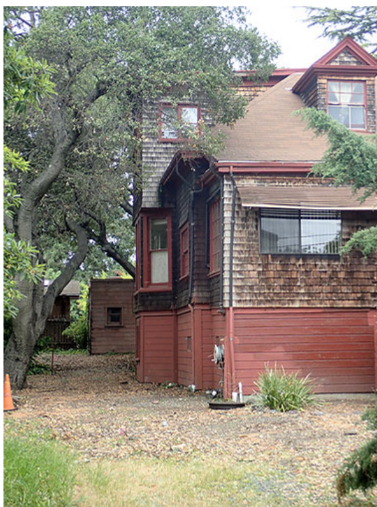
Figure 14. Enclosed porch, southwest corner
