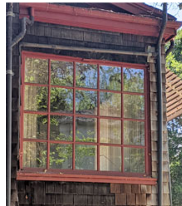
Figure 15. West-facing window in front porch
