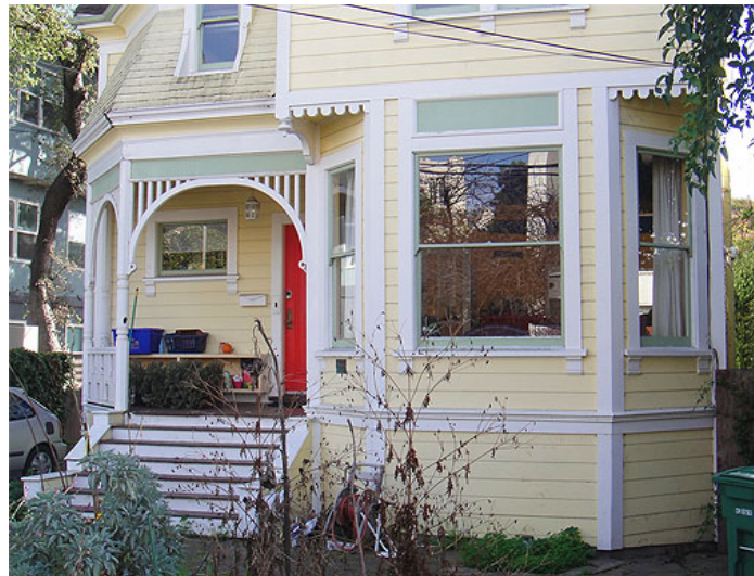
Figure 9. Rustic siding, Luttrell House
