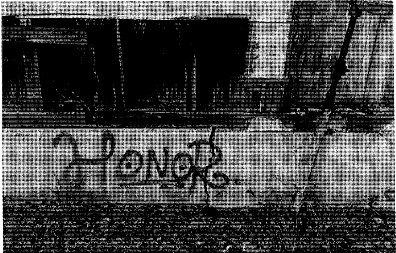
Fig.7 – 639 Arlington Ave. – West side foundations
