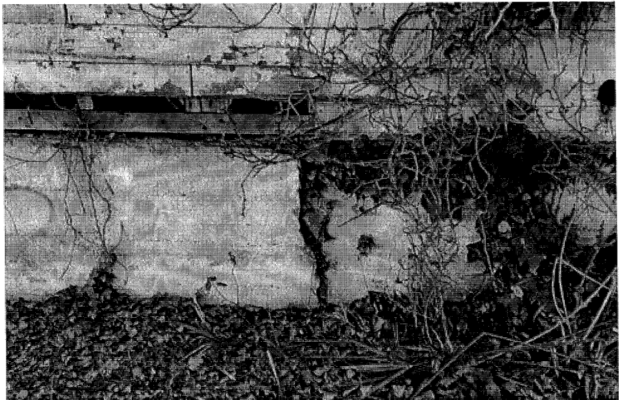
Fig.8 – 639 Arlington Ave. – West side foundations
