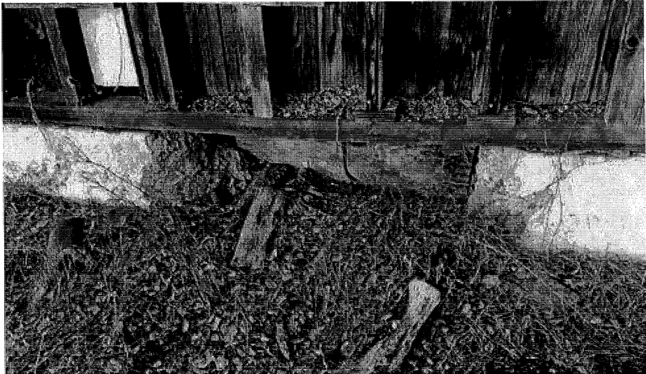
Fig.6 – 639 Arlington Ave. – West side foundations
