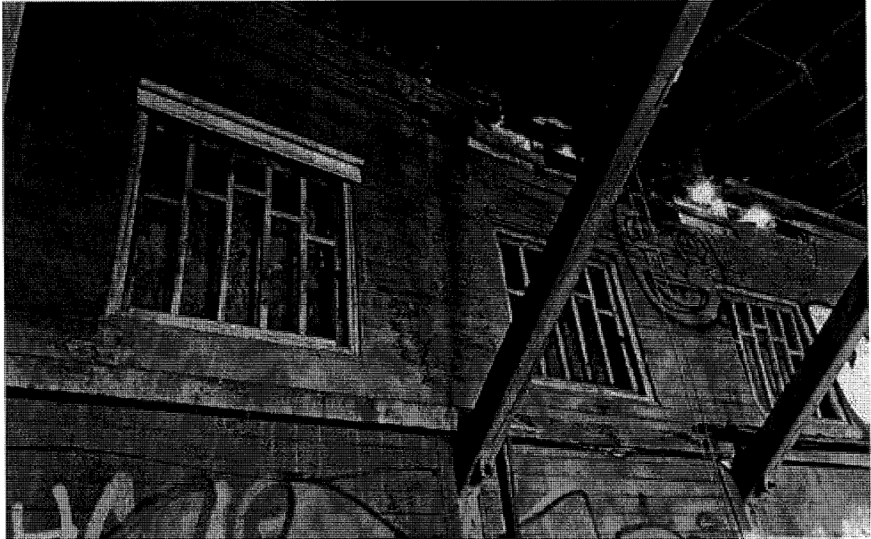
Fig.10 – 639 Arlington Ave. – Interior, east side wall and roof
