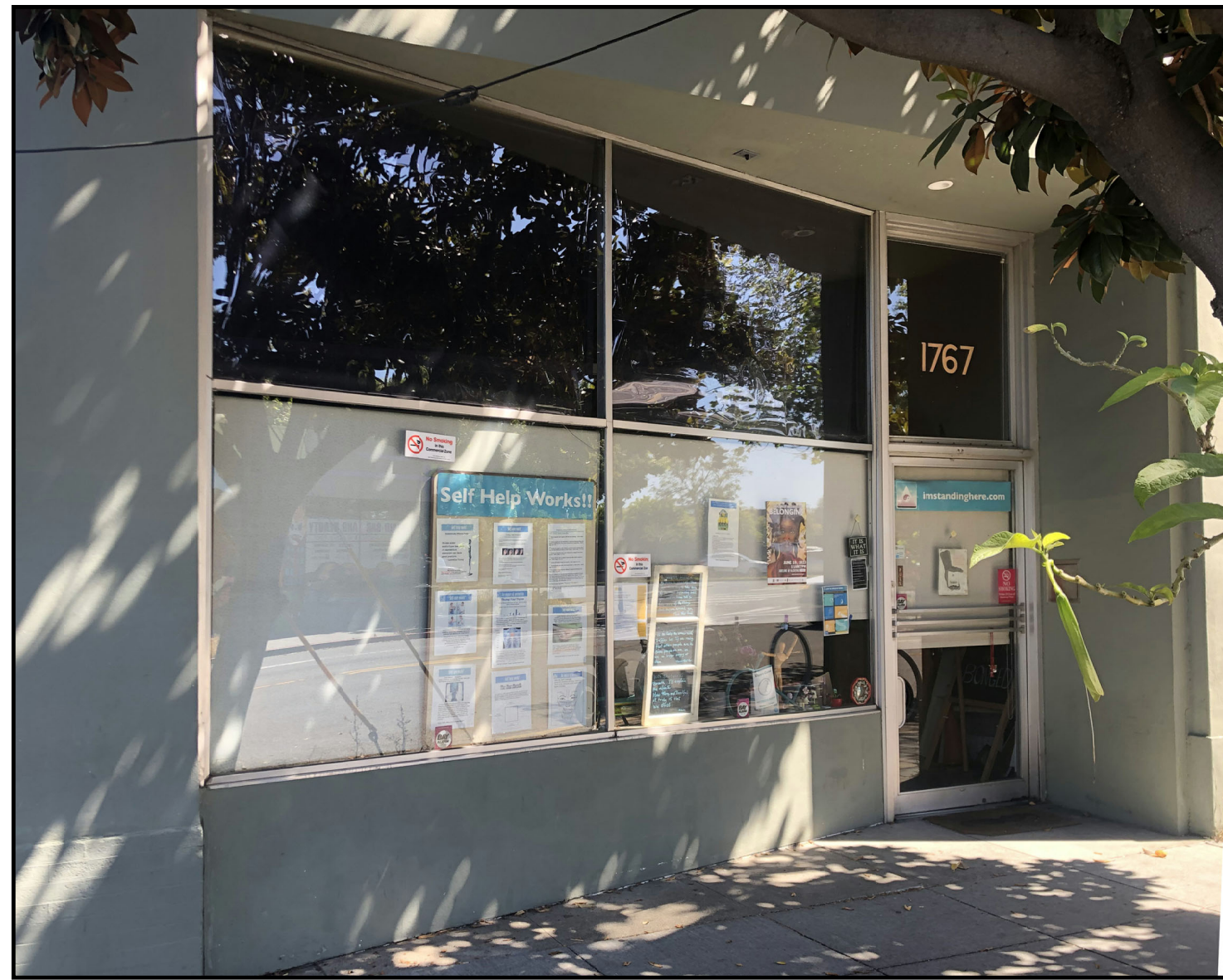
1767 ALCATRAZ - (E) FACADE
