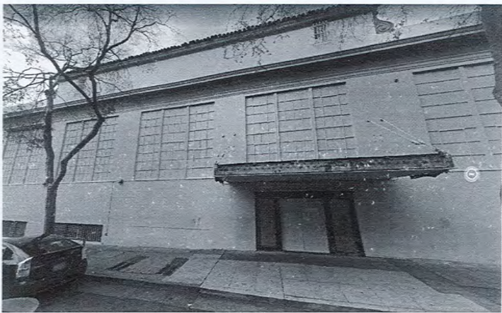
4 SITE PHOTO - KITTREDGE ST FACADE A0-003 12" = 1'-0"
