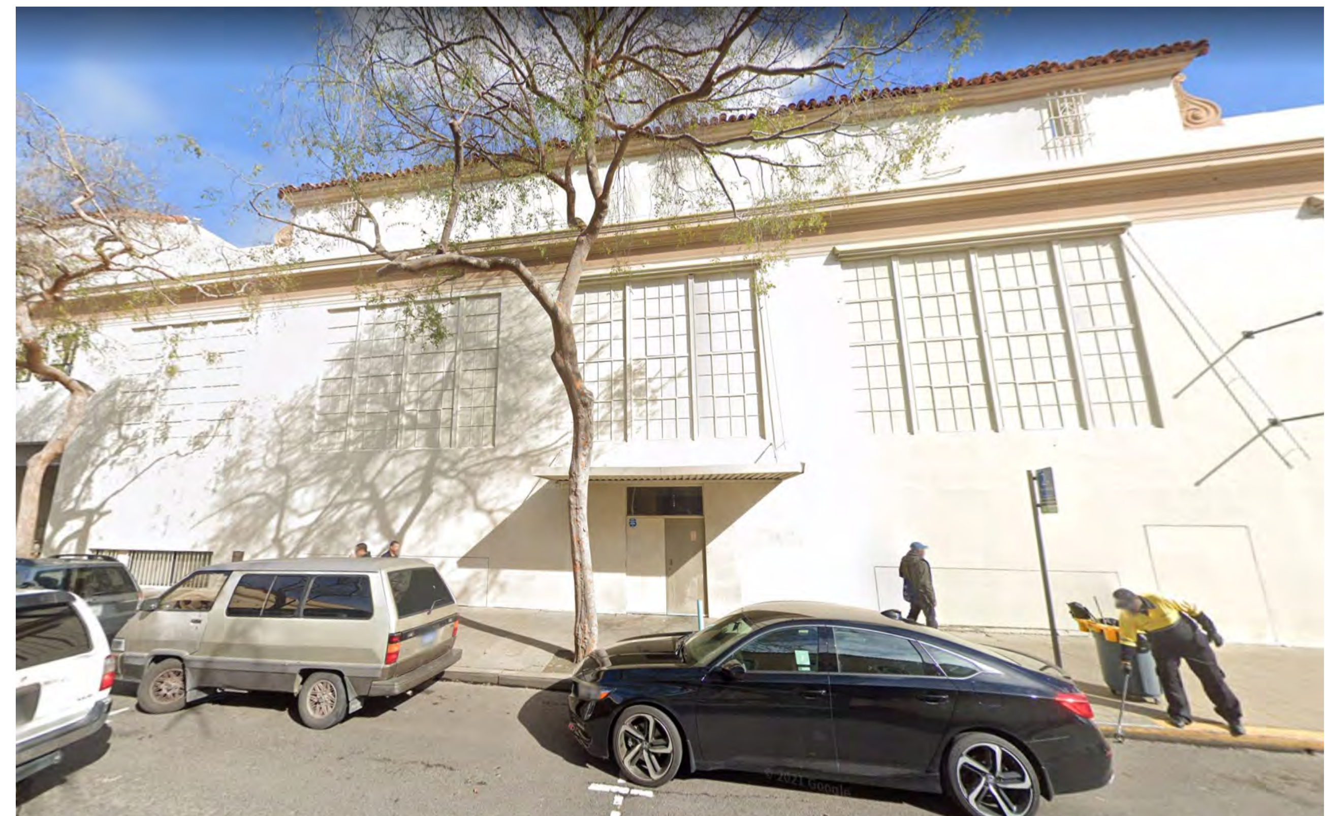
3 SITE PHOTO - HAROLD WAY SOUTH FACADE AD-002 12" = 1'-0"
