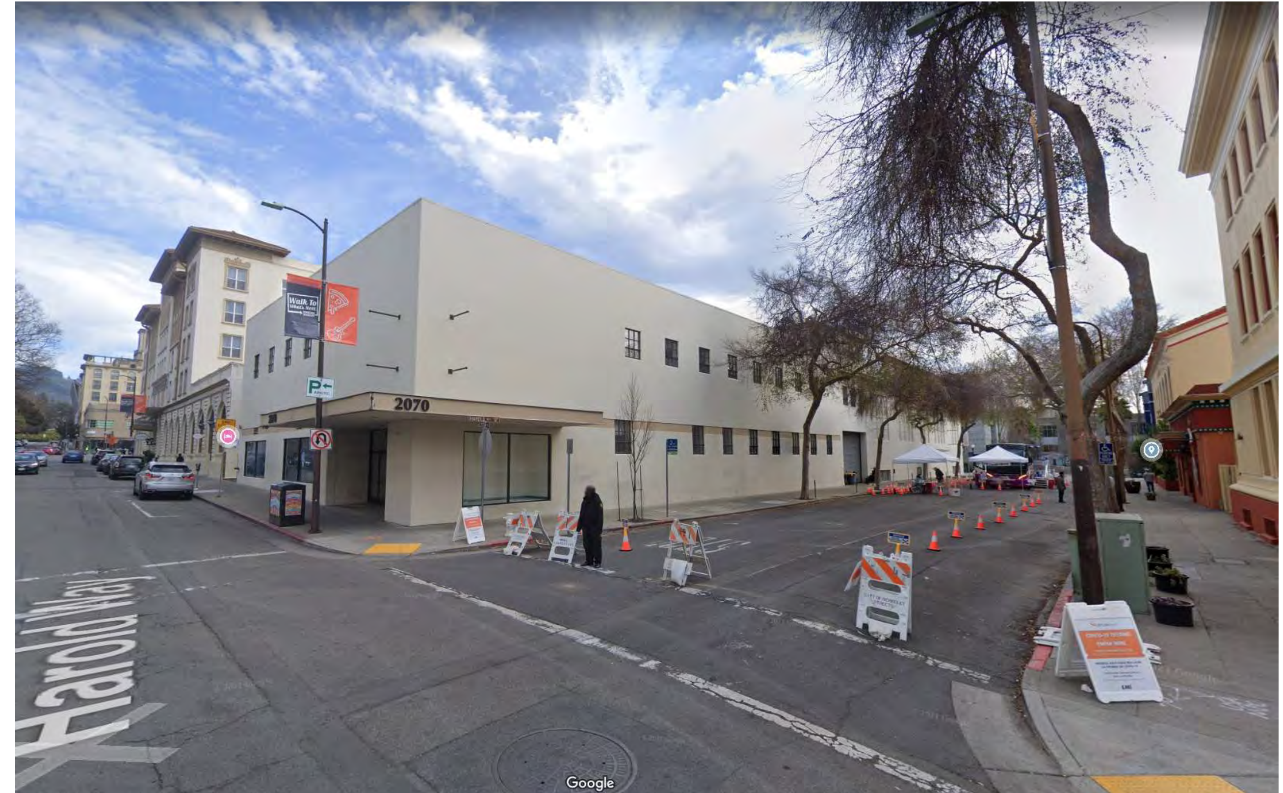
2 SITE PHOTO - ALLSTON WAY AND HAROLD WAY - LOOKING EAST A0-001 12" = 1'-0"
