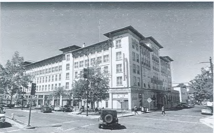
3 SITE PHOTO - SHATTUCK AVE AND ALLSTON WAY - EXISTING HOTEL A0-003 12' x 1'-0"
