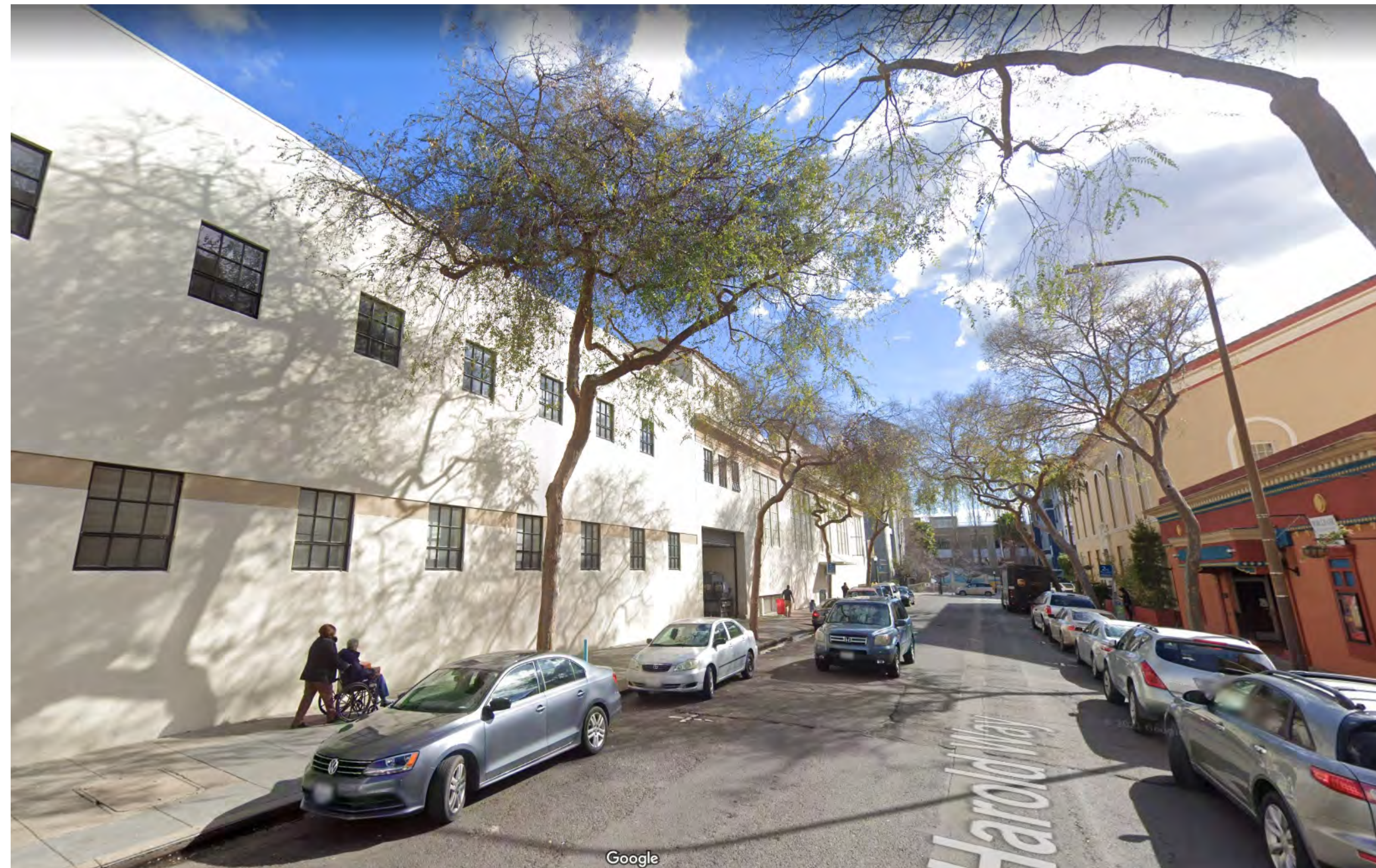
3 SITE PHOTO - HAROLD WAY - LOOKING SOUTH A0-001 12" = 1'-0"
