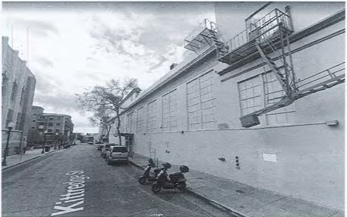
4 SITE PHOTO - KITTREDGE ST - LOOKING WEST (42-00) 12" x 1'-0"
