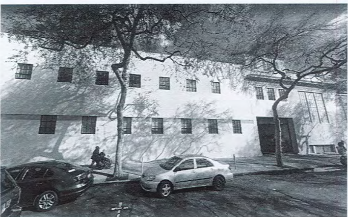
2 SITE PHOTO - HAROLD WAY NORTH FACADE A0-005 12" = 1'-0"
