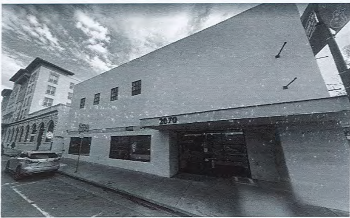
1 SITE PHOTO - ALLSTON WAY FACADE A0-002 12" = 1'-0"
