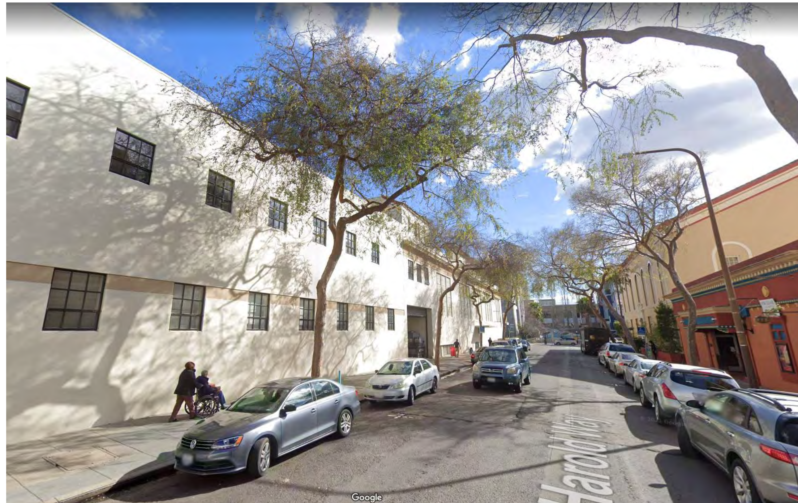
3 SITE PHOTO - HAROLD WAY - LOOKING SOUTH A0-001 12" = 1'-0"
