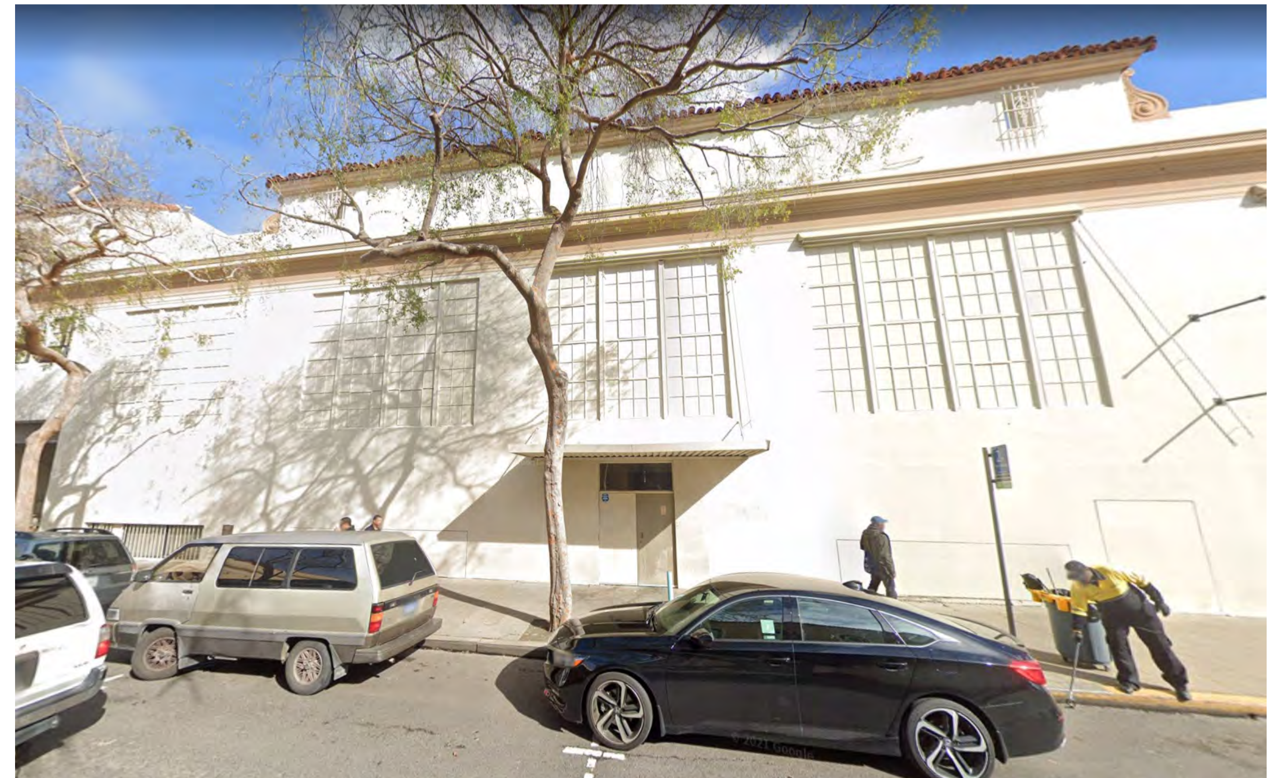
3 SITE PHOTO - HAROLD WAY SOUTH FACADE AD-002 12" = 1'-0"
