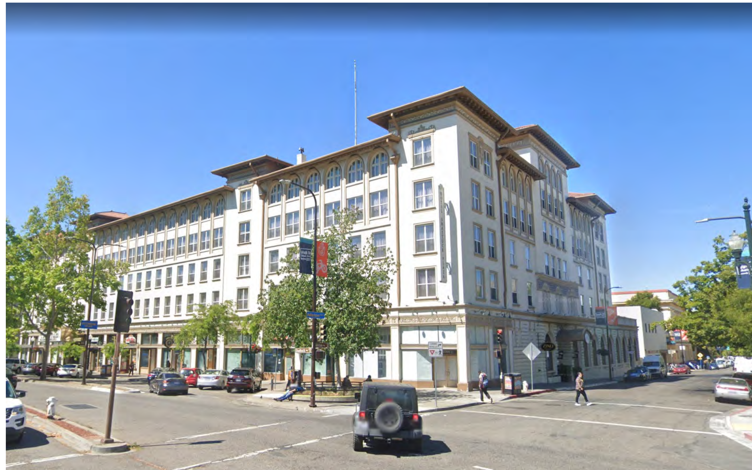
3 SITE PHOTO - SHATTUCK AVE AND ALLSTON WAY - EXISTING HOTEL A0-003 12" = 1'-0"
