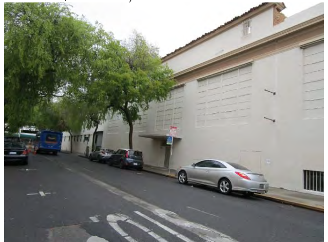
West elevation across Kittridge, view northeast. (Rincon Consultants, March 2022).
