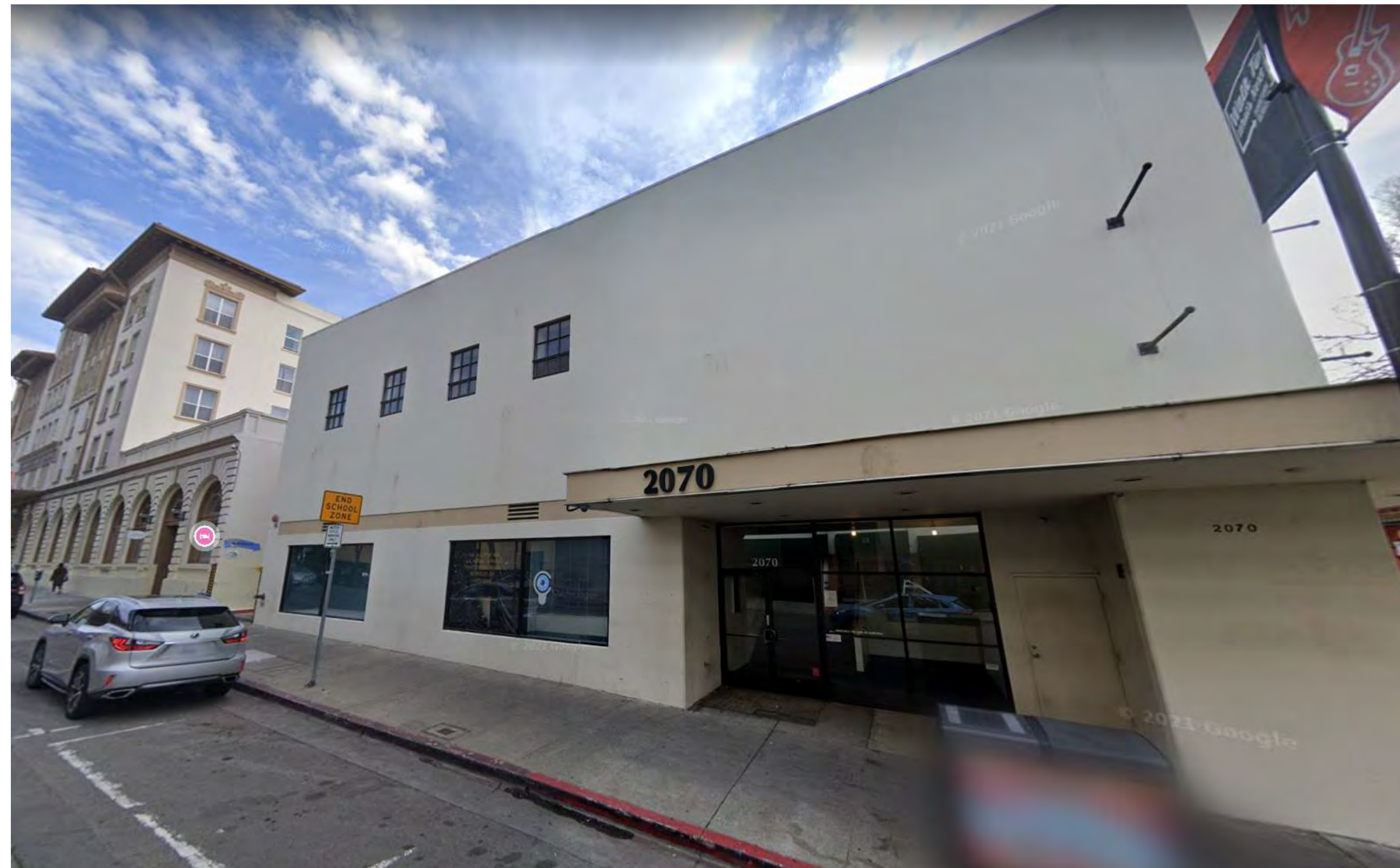
1 SITE PHOTO - ALLSTON WAY FACADE AD-002 12" = 1'-0"
