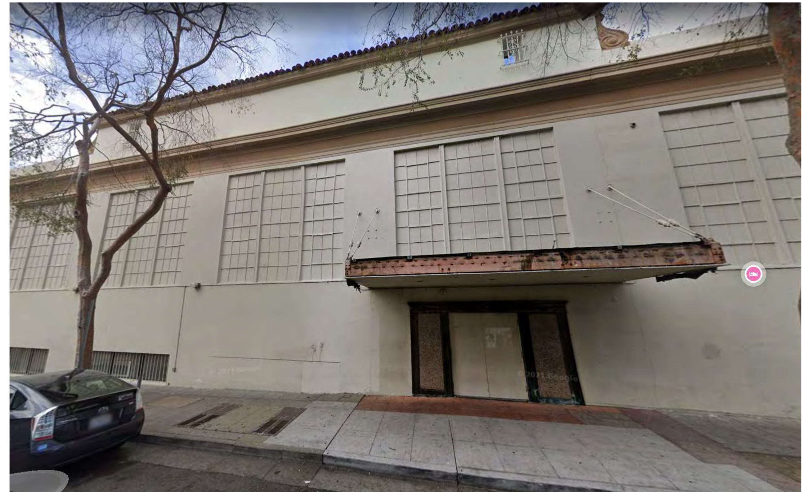
4 SITE PHOTO - KITTREDGE ST FACADE AD-002 12" = 1'-0"
