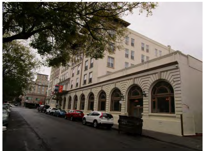
North elevation, view southeast. (Rincon Consultants, March 2022).
