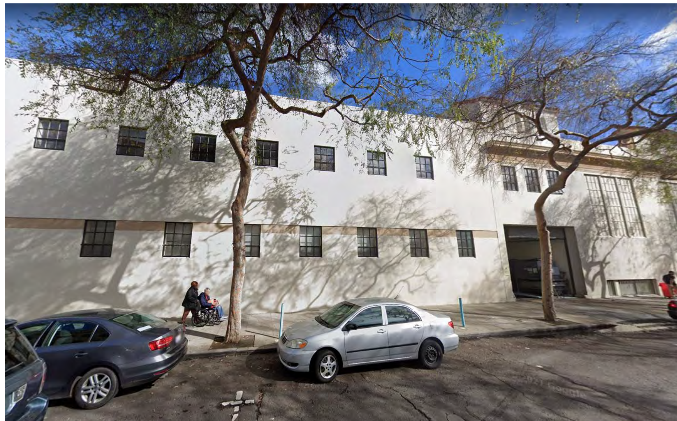
2 SITE PHOTO - HAROLD WAY NORTH FACADE AD-002 12" = 1'-0"
