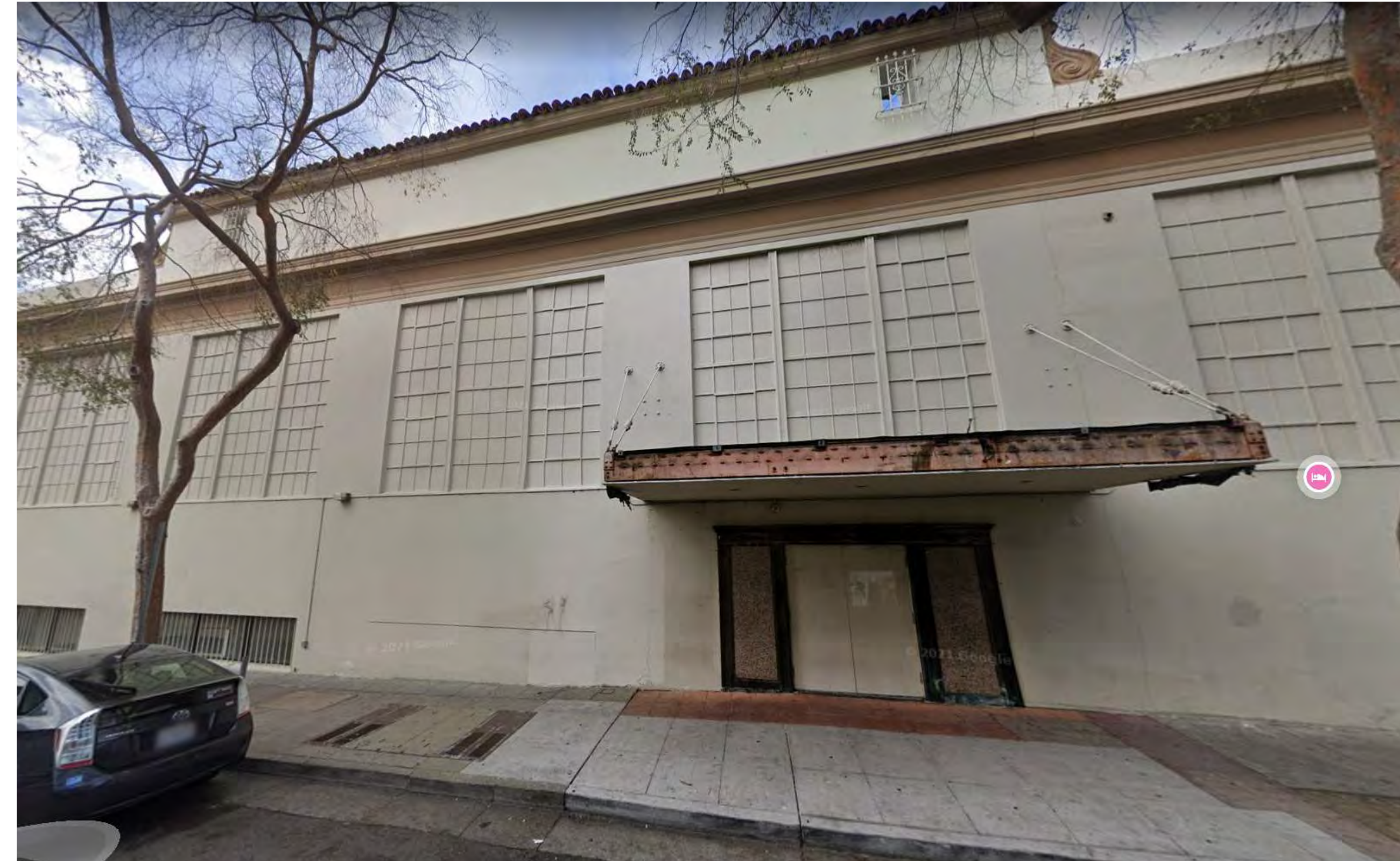
4 SITE PHOTO - KITTREDGE ST FACADE AD-002 12" = 1'-0"
