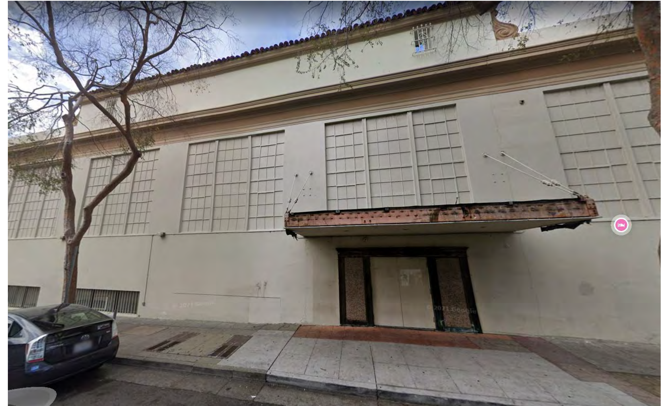
4 SITE PHOTO - KITTREDGE ST FACADE AD-002 12" = 1'-0"
