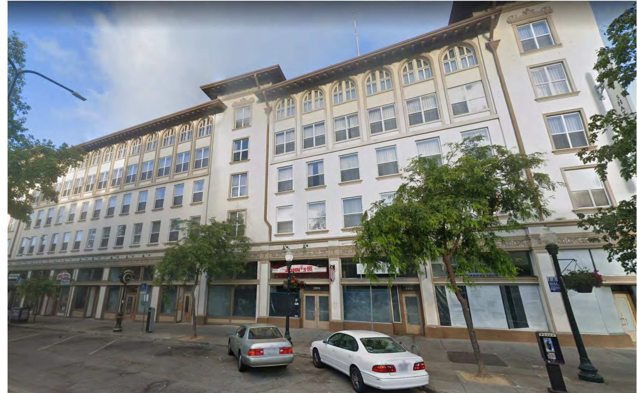
2 SITE PHOTO - SHATTUCK AVE - EXISTING HOTEL A0-003 12" = 1'-0"
