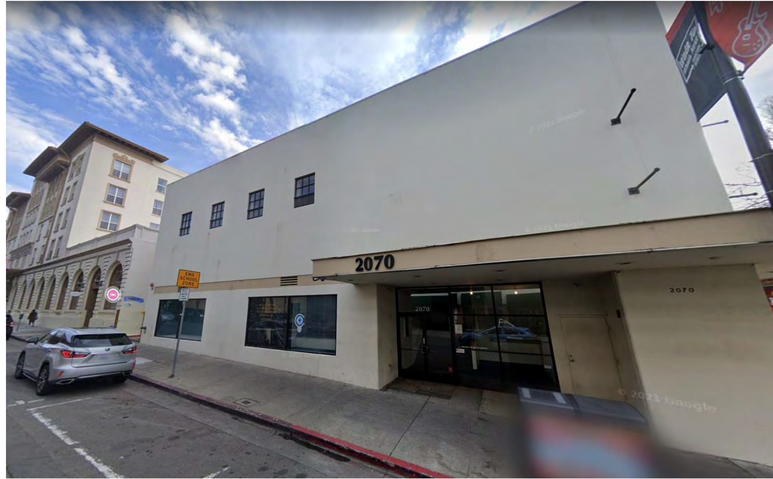
1 SITE PHOTO - ALLSTON WAY FACADE AD-002 12" = 1'-0"
