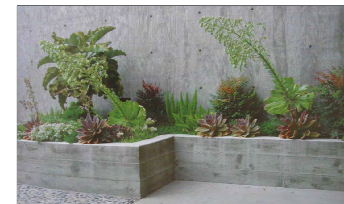
BUILT-IN CONCRETE WALLS WITH HORIZONTAL BOARDFORM FINISH
