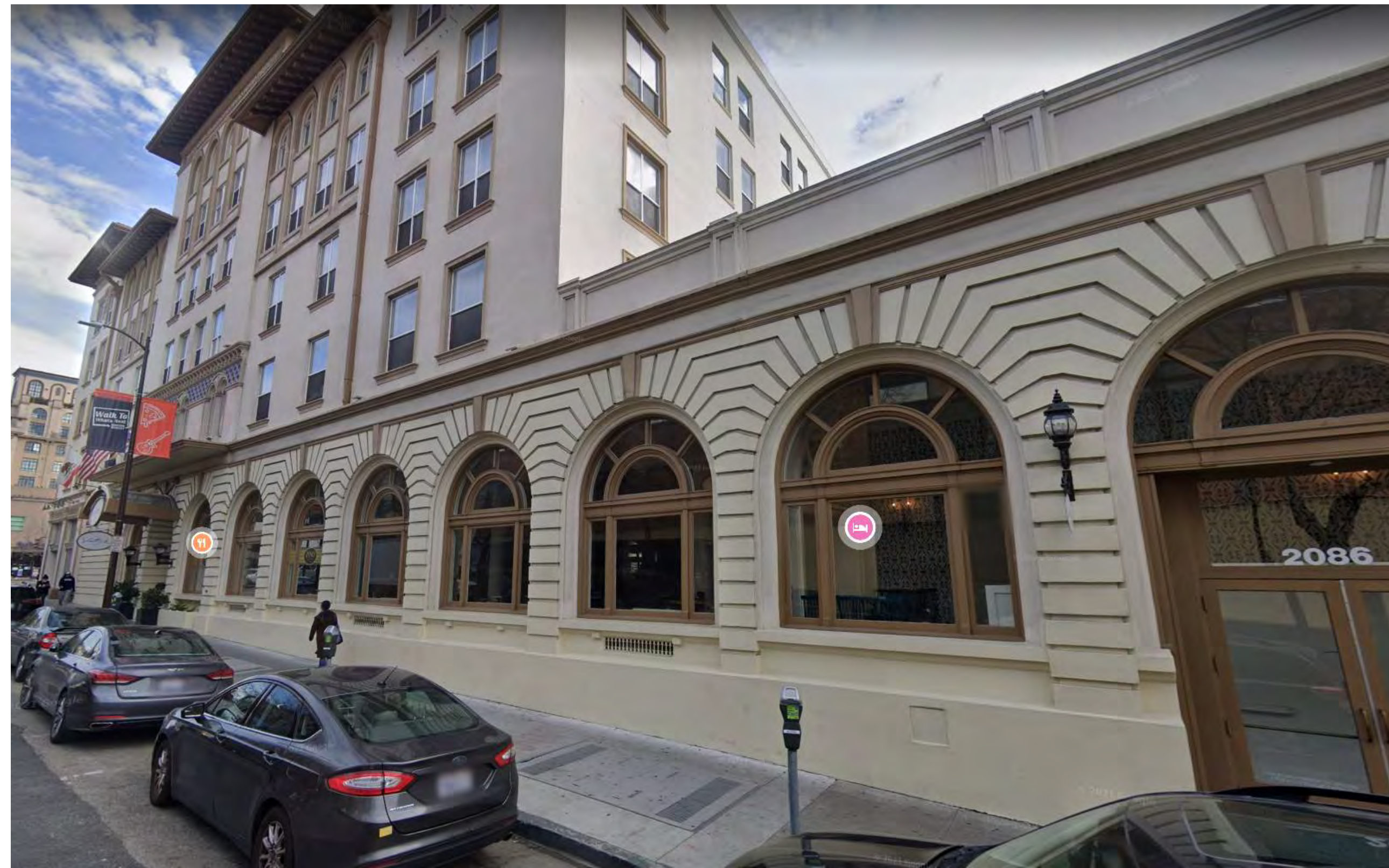
1 SITE PHOTO - ALLSTON WAY - EXISTING HOTEL A0-003 12" = 1'-0"
