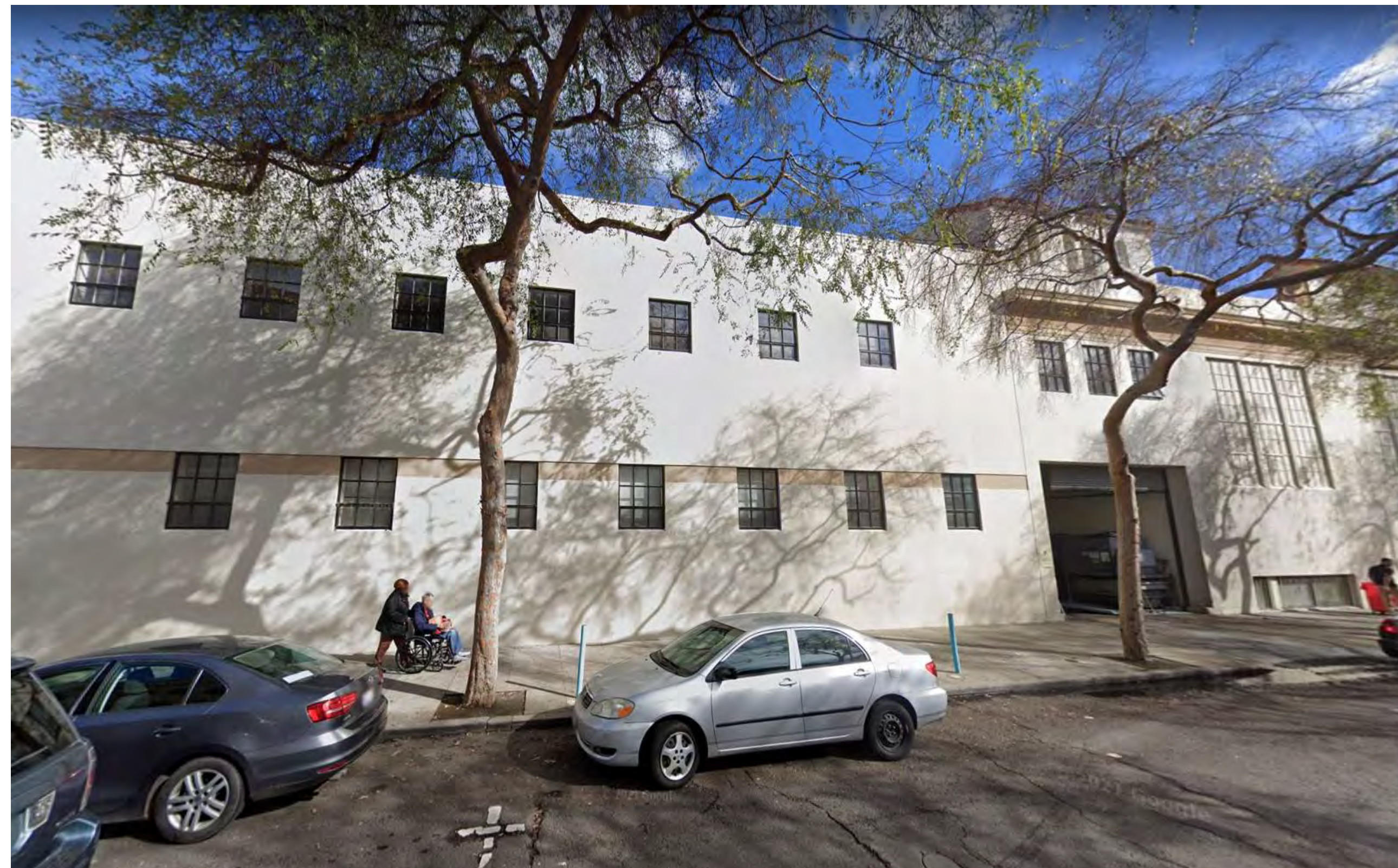
2 SITE PHOTO - HAROLD WAY NORTH FACADE AD-002 12" = 1'-0"
