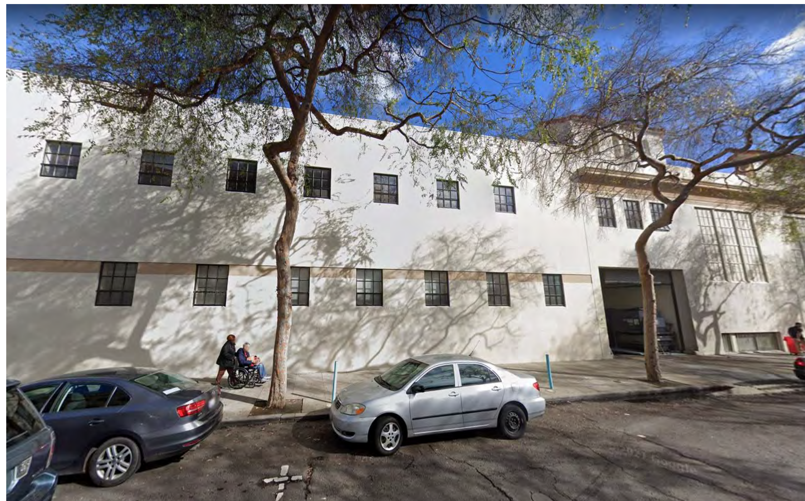
2 SITE PHOTO - HAROLD WAY NORTH FACADE AD-002 12" = 1'-0"
