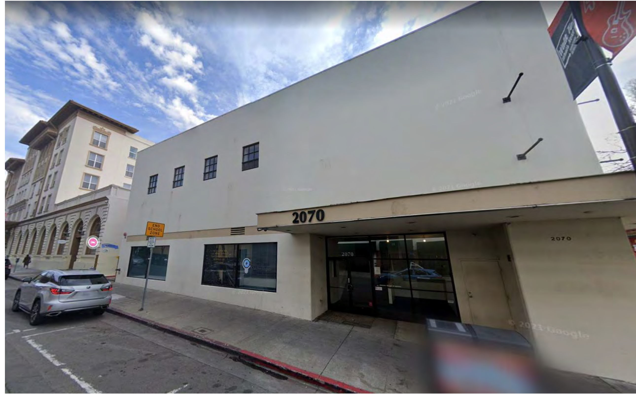
1 SITE PHOTO - ALLSTON WAY FACADE AD-002 12" = 1'-0"
