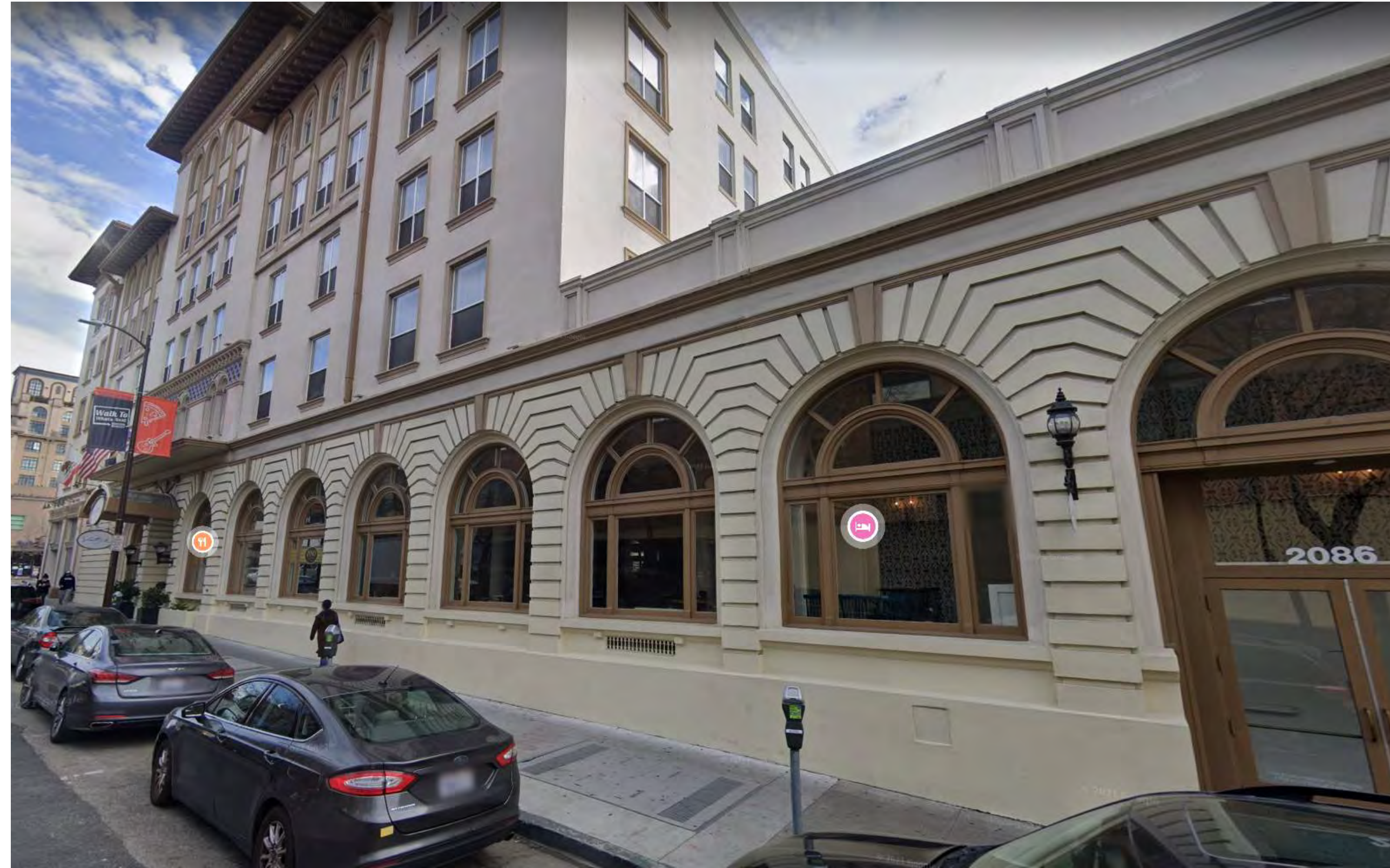
1 SITE PHOTO - ALLSTON WAY - EXISTING HOTEL A0-003 12" = 1'-0"
