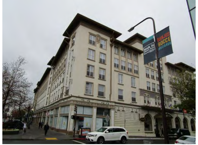
Detail of northeast corner of Shattuck Hotel. (Rincon Consultants, March 2022)
