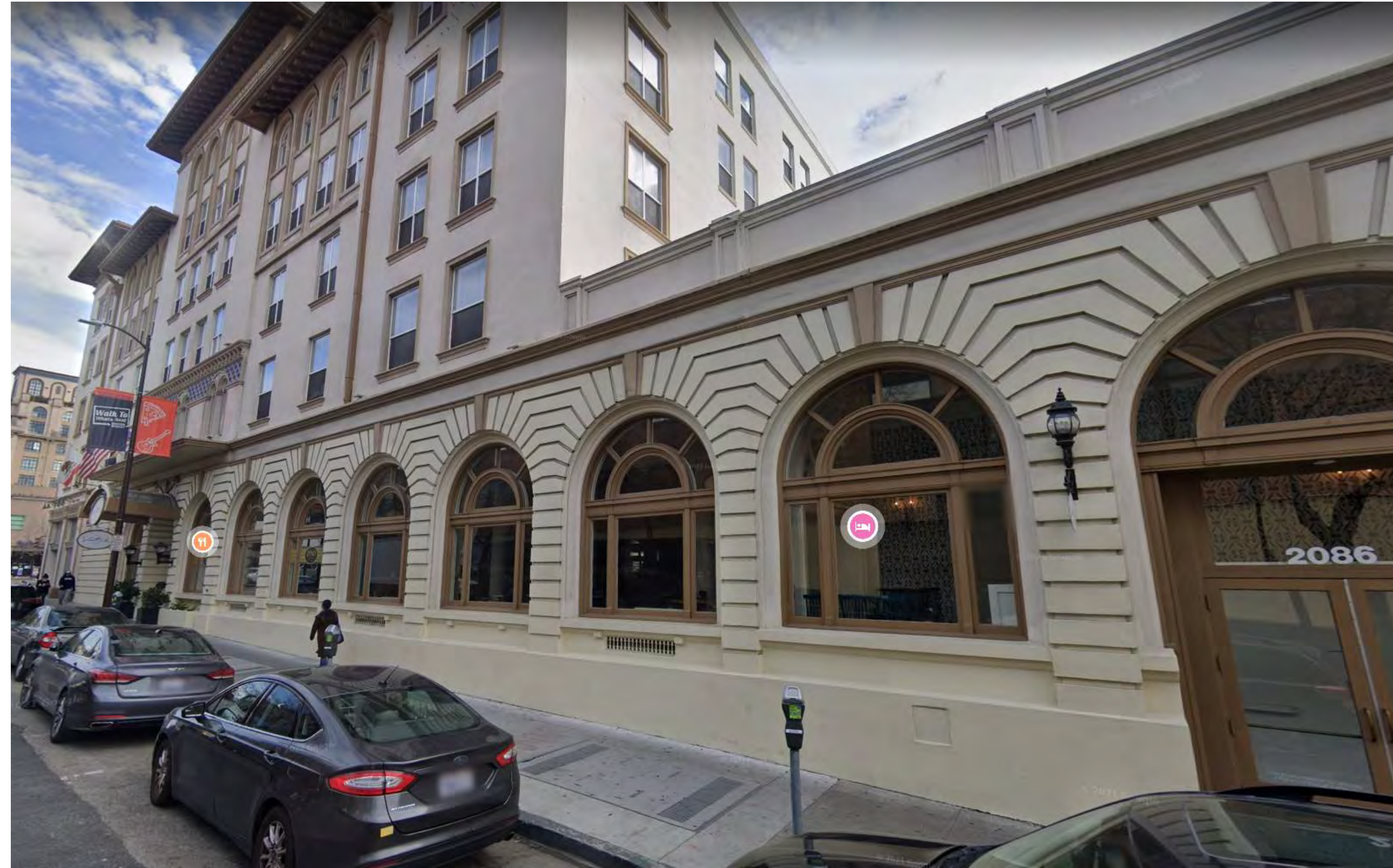
1 SITE PHOTO - ALLSTON WAY - EXISTING HOTEL A0-003 12" = 1'-0"
