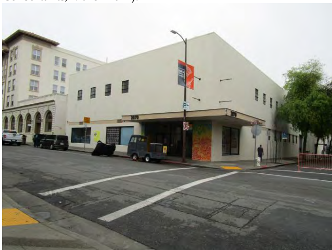
North elevation with Hink's Building (non-contributing) in foreground, view southeast. (Rincon Consultants, March 2022)
