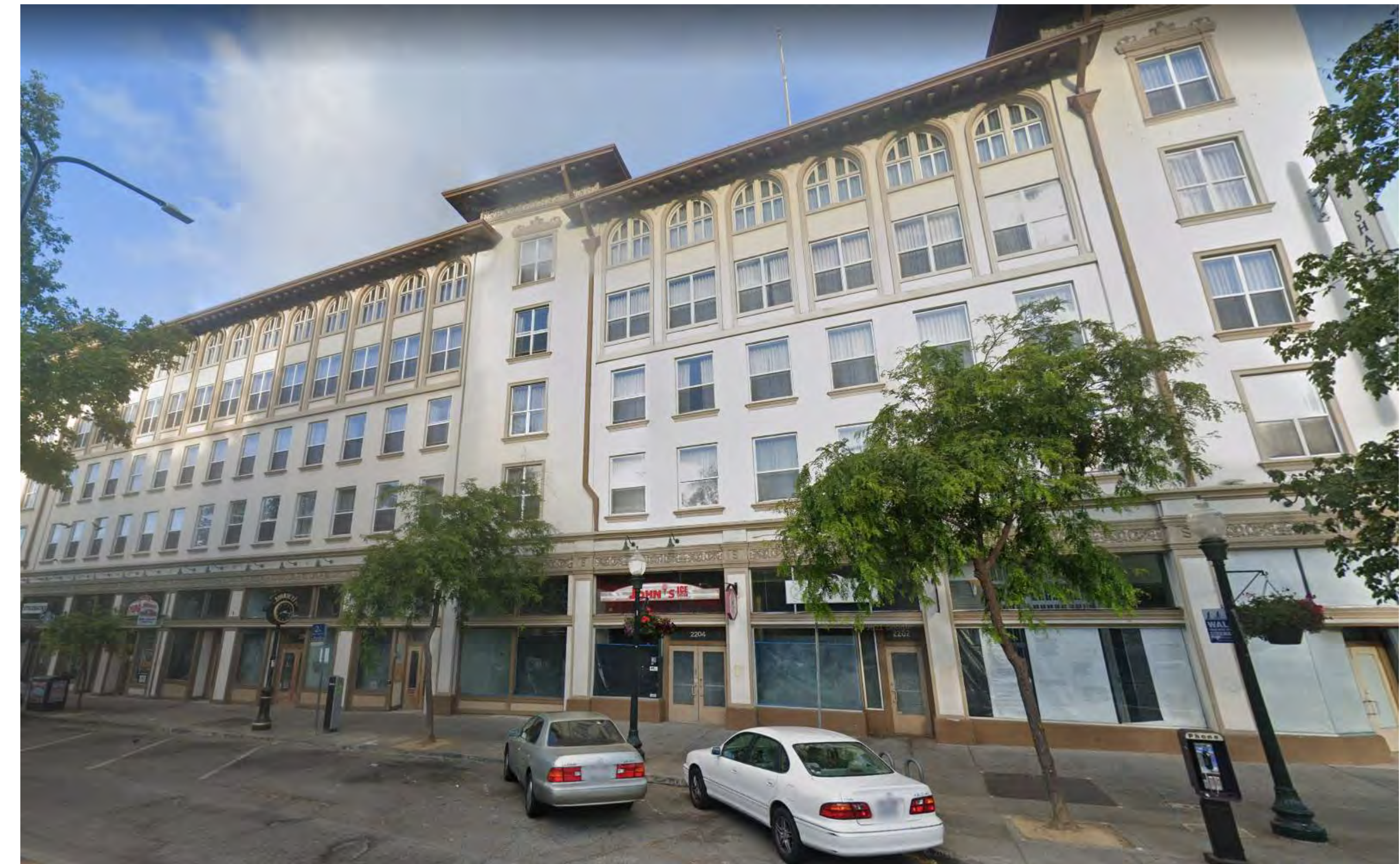
2 SITE PHOTO - SHATTUCK AVE - EXISTING HOTEL A0-003 12" = 1'-0"
