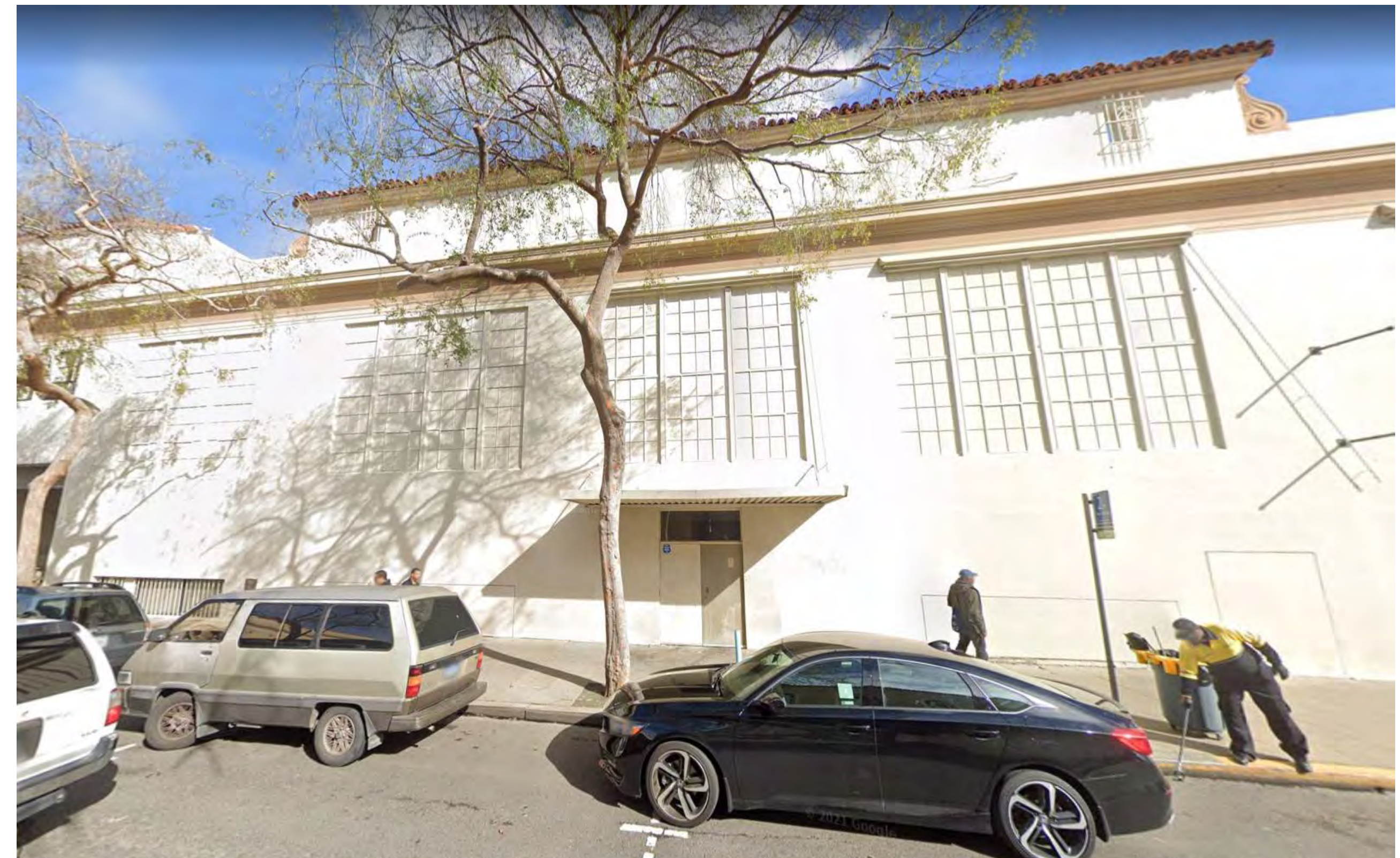
3 SITE PHOTO - HAROLD WAY SOUTH FACADE AD-002 12" = 1'-0"
