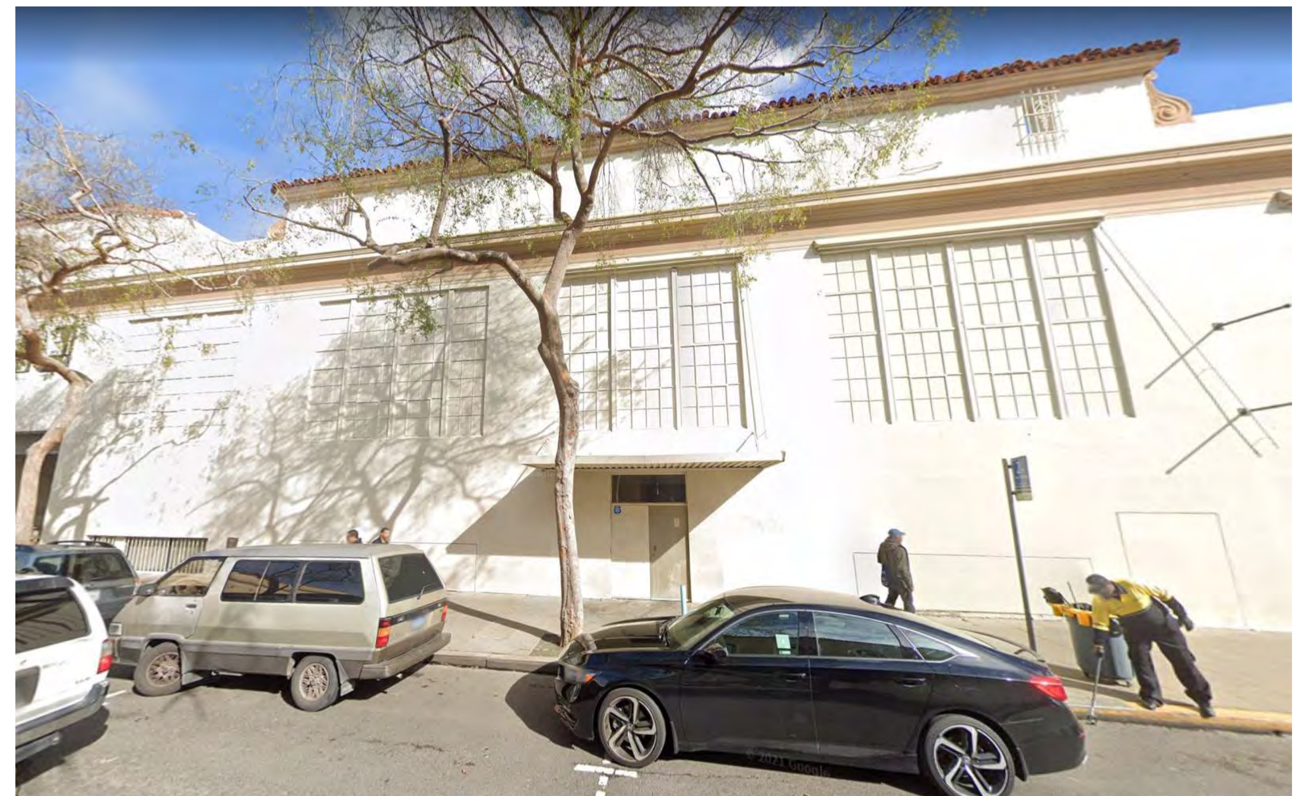
3 SITE PHOTO - HAROLD WAY SOUTH FACADE AD-002 12" = 1'-0"
