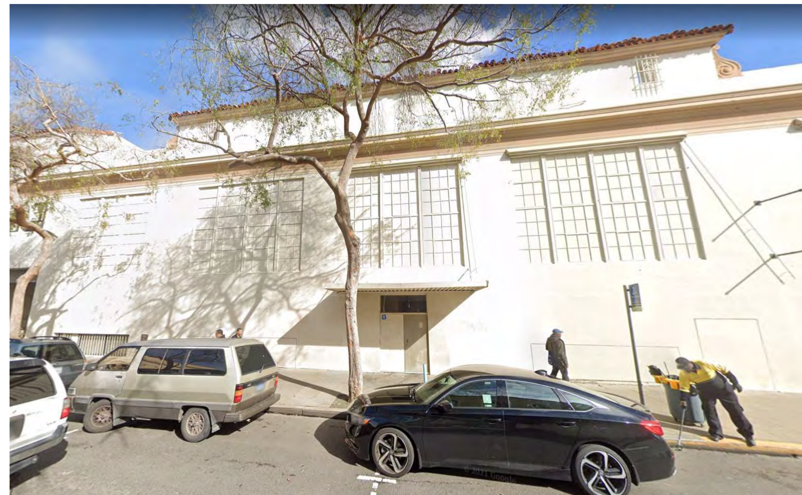
3 SITE PHOTO - HAROLD WAY SOUTH FACADE AD-002 12" = 1'-0"
