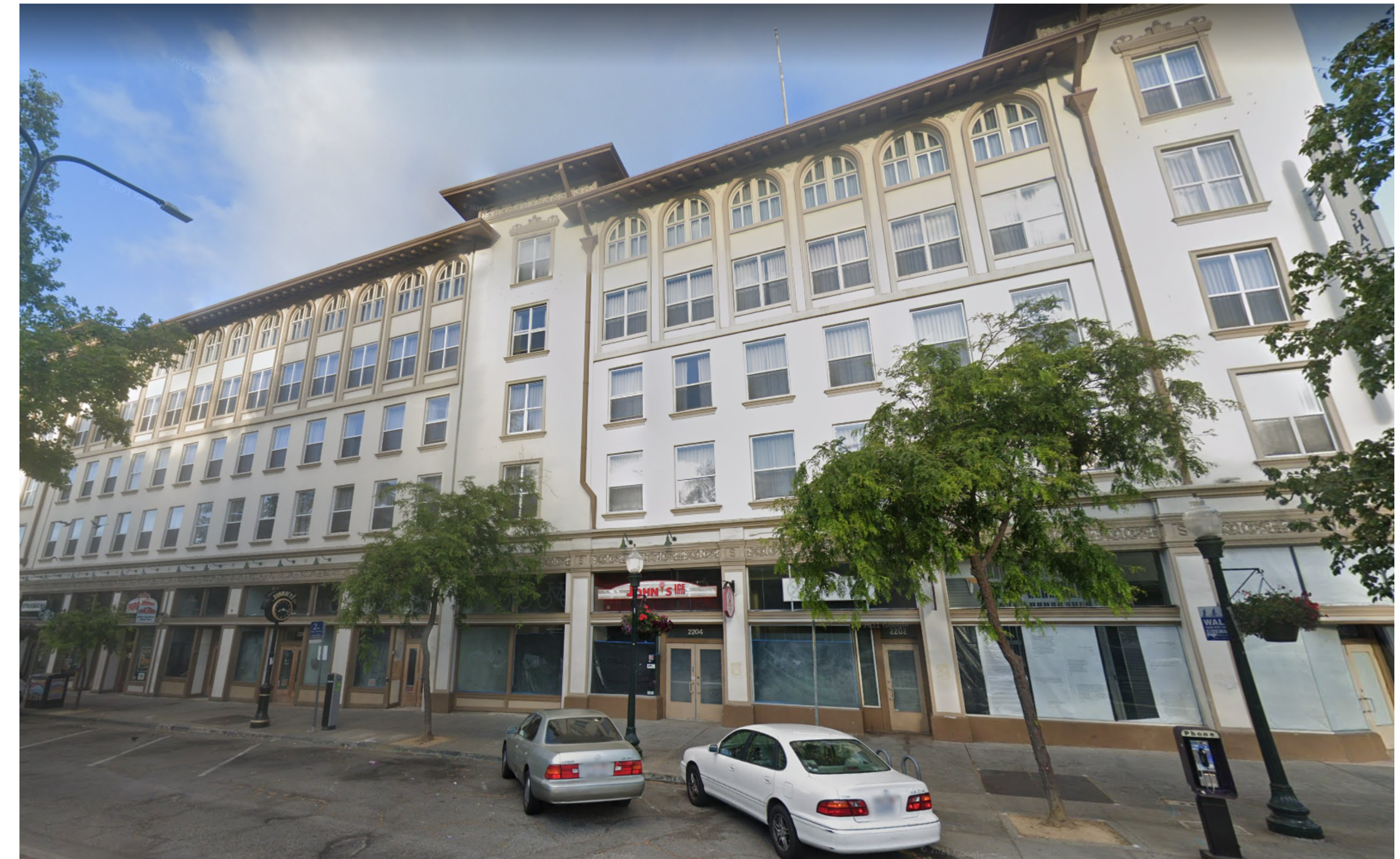
2 SITE PHOTO - SHATTUCK AVE - EXISTING HOTEL A0-003 12" = 1'-0"
