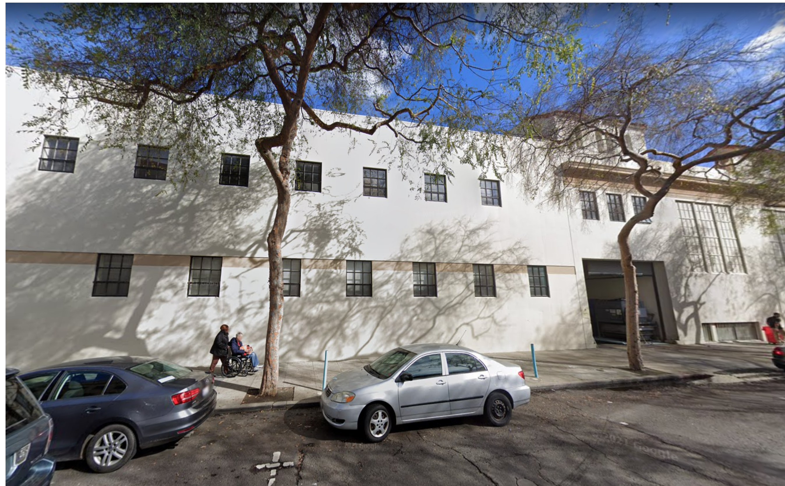
2 SITE PHOTO - HAROLD WAY NORTH FACADE A0-002 12" = 1'-0"
