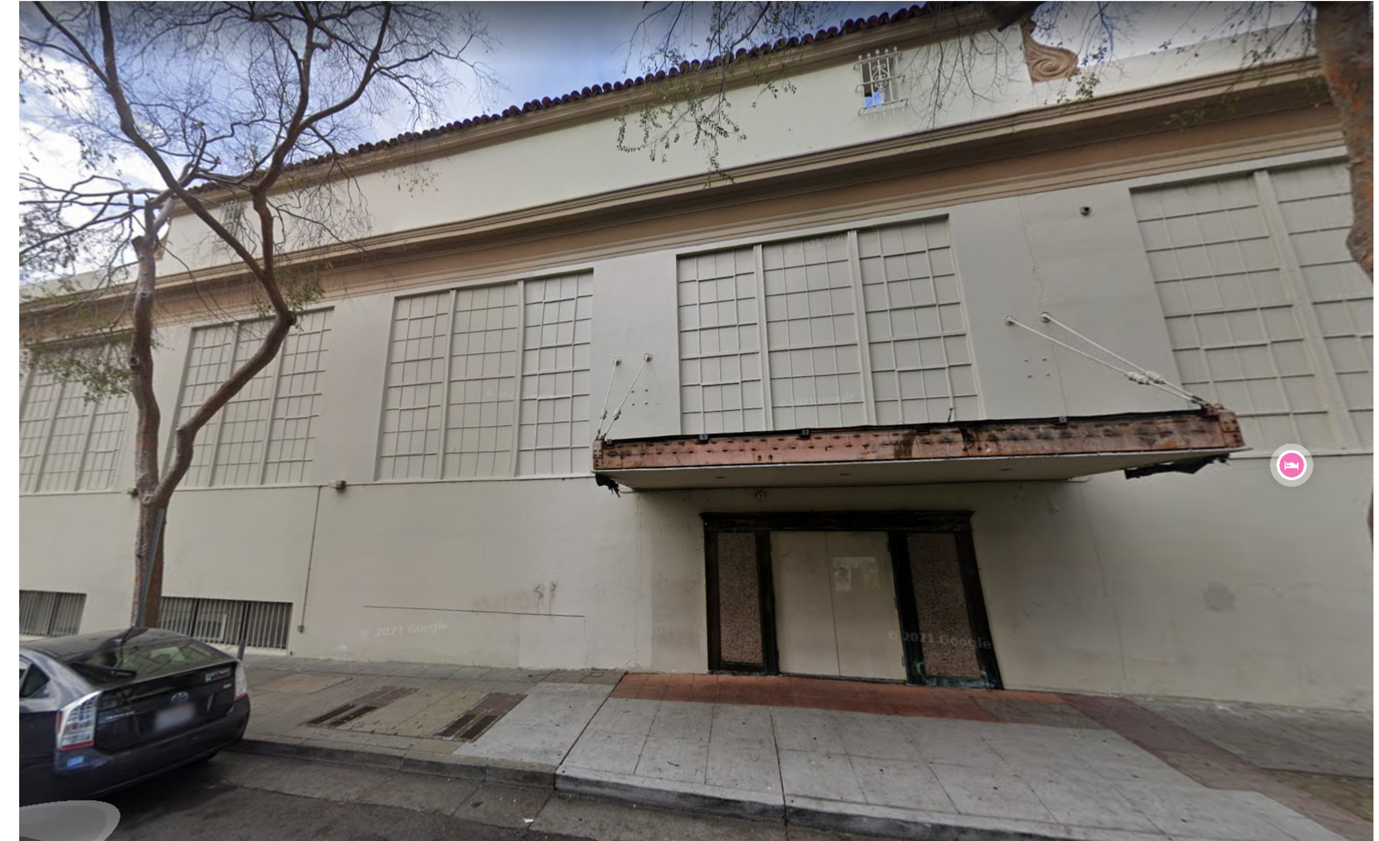
4 SITE PHOTO - KITTREDGE ST FACADE A0-002 12" = 1'-0"
