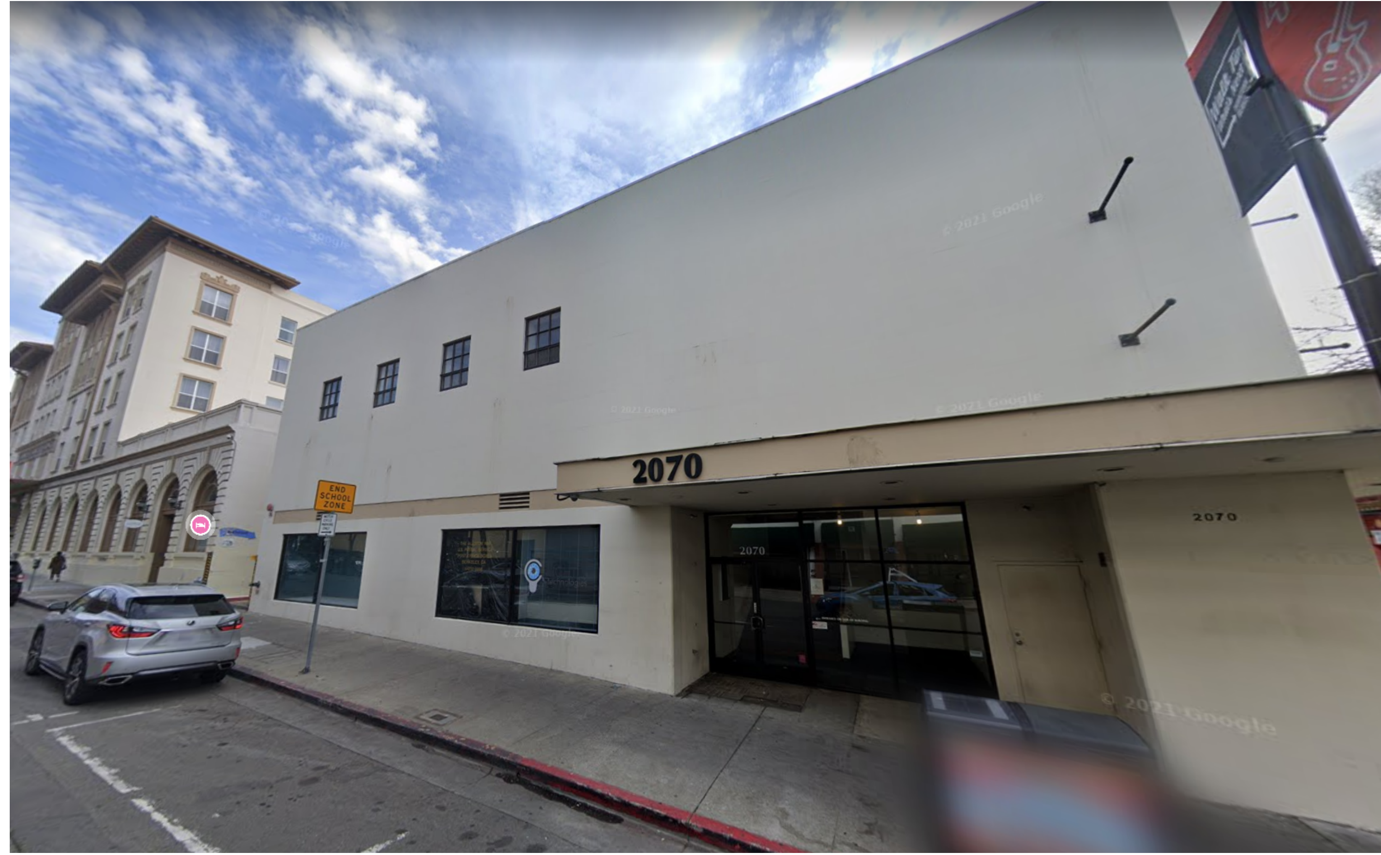
1 SITE PHOTO - ALLSTON WAY FACADE A0-002 12" = 1'-0"
