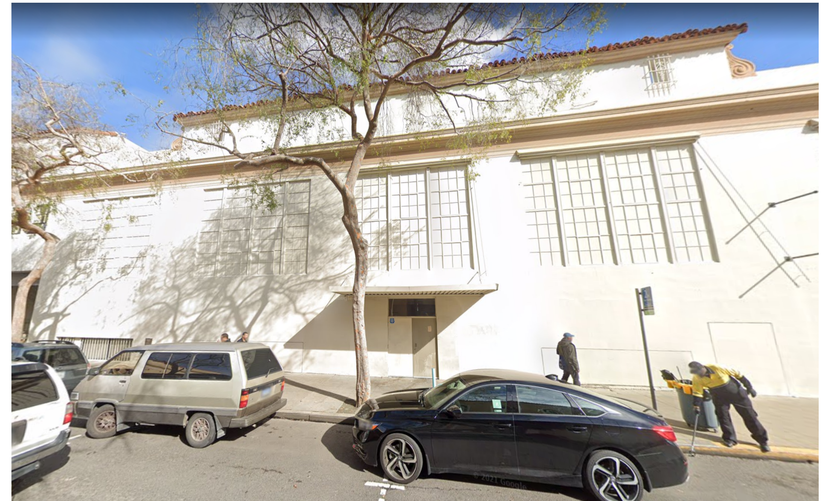
3 SITE PHOTO - HAROLD WAY SOUTH FACADE A0-002 12" = 1'-0"
