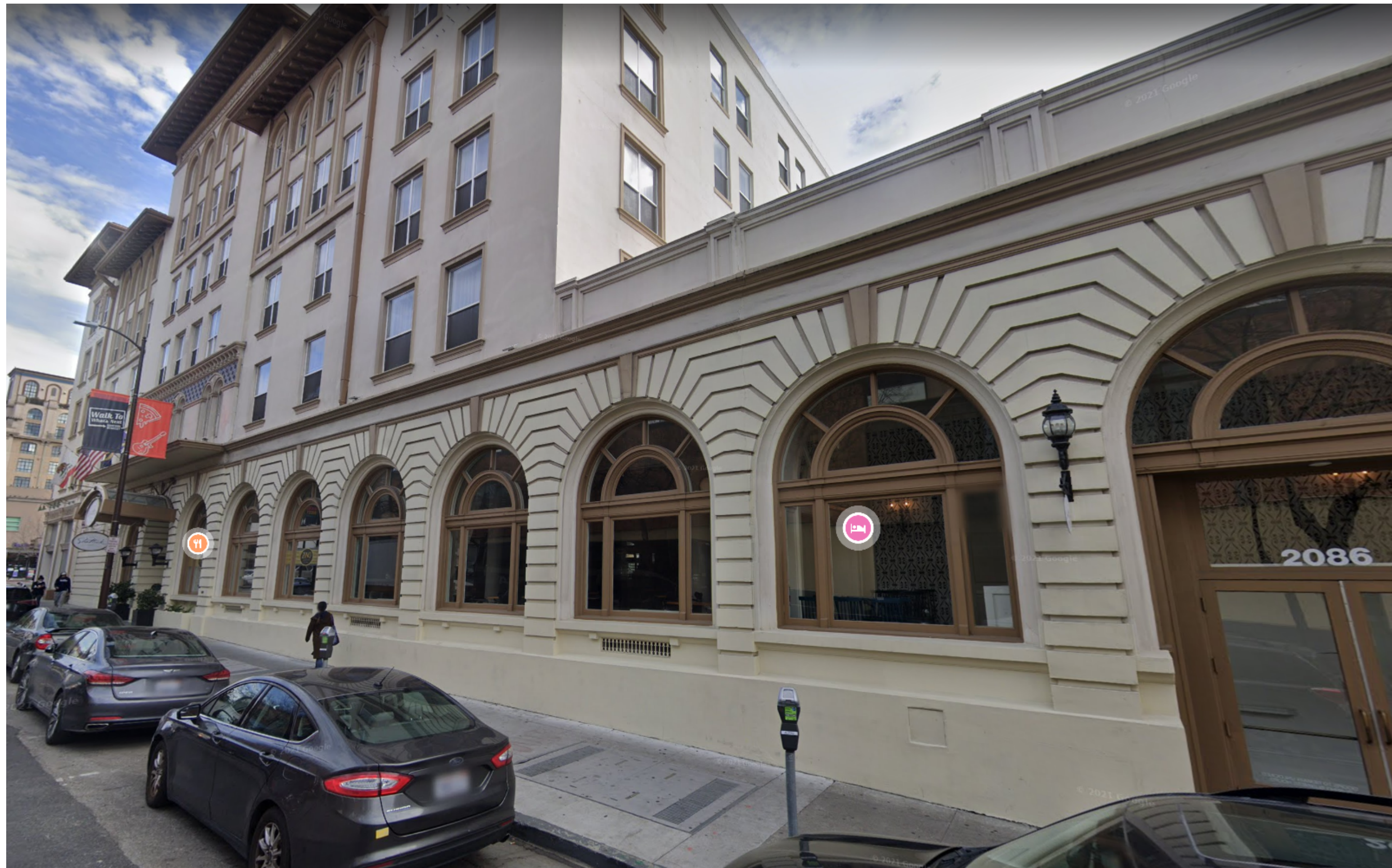
1 SITE PHOTO - ALLSTON WAY - EXISTING HOTEL A0-003 12" = 1'-0"
