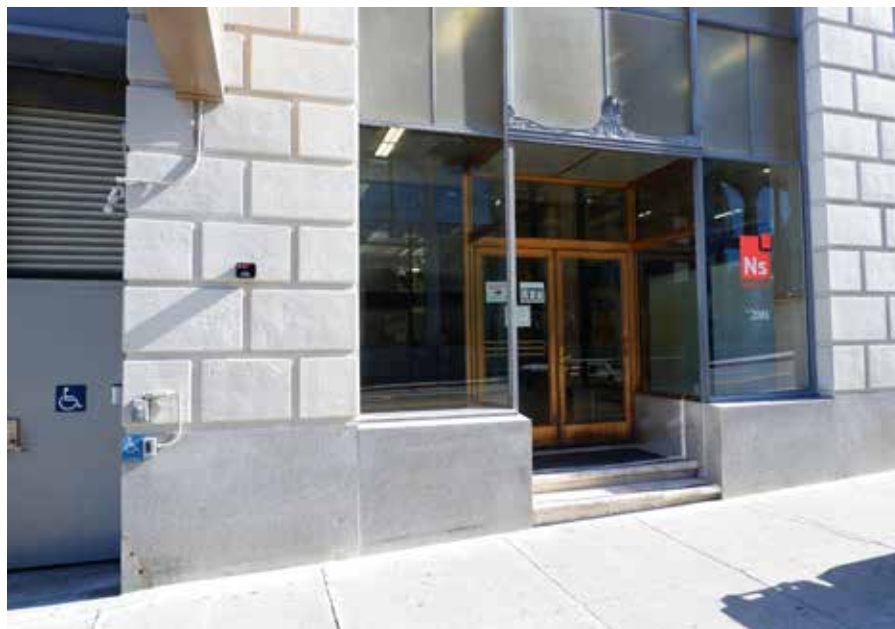
7. View of existing pedestrian entrance on Center Street. Note existing accessible entry on the left side of photo.
