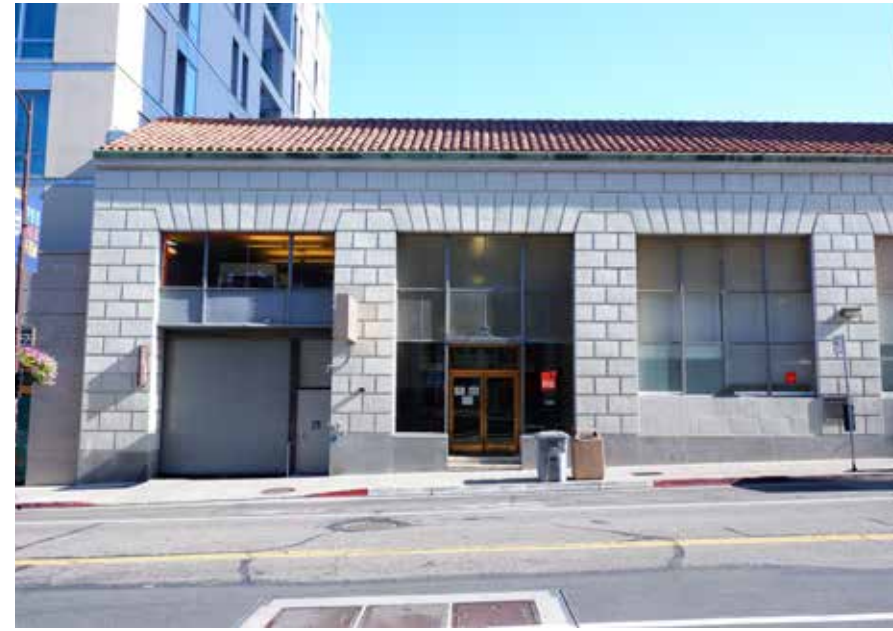
2. View of existing Center Street entrances. Accessible entrance is located immediately adjacent the vehicle entrance.
