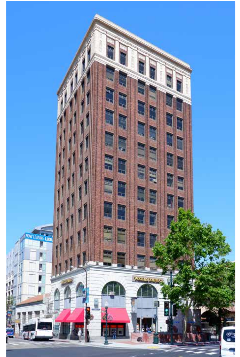
4. View of office tower, looking northwest from Shattuck Avenue.
