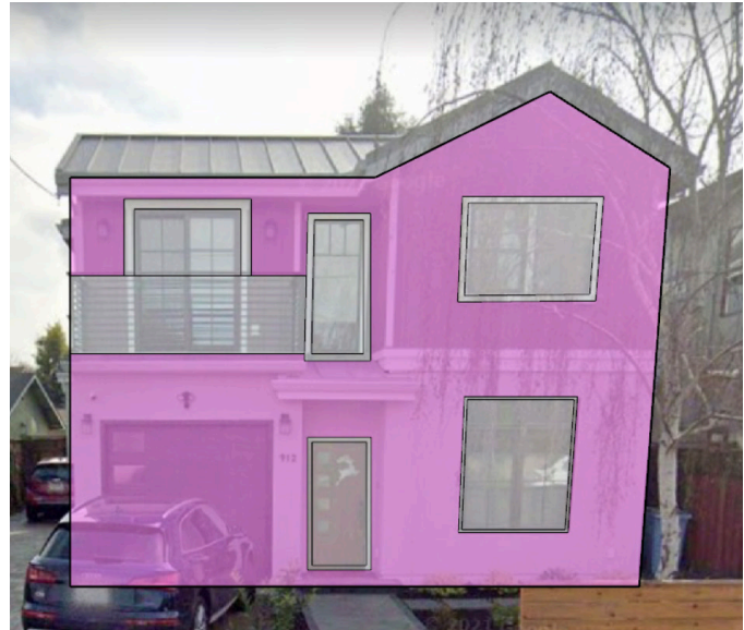
908 Cedar, Berkeley Openings are approximately 30%
