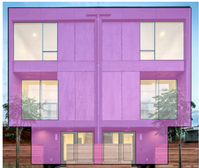
1030 Grayson, Berkeley Openings are approximately 32%
