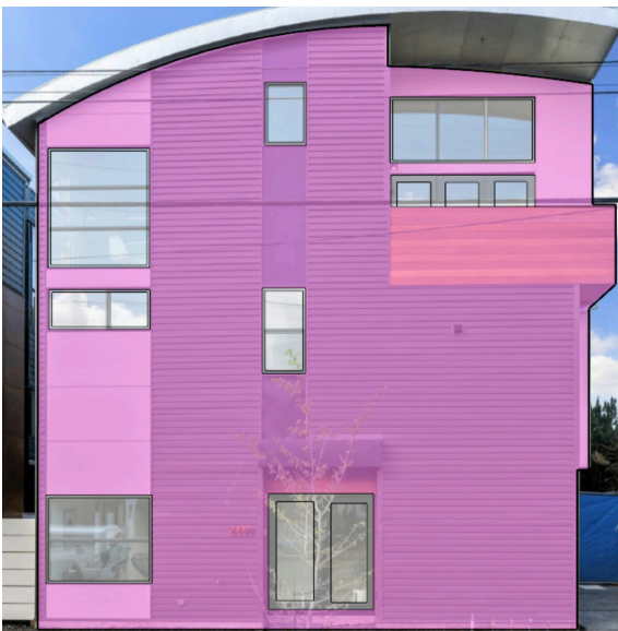
1444 Fifth Street, Berkeley Openings are approximately 19%
