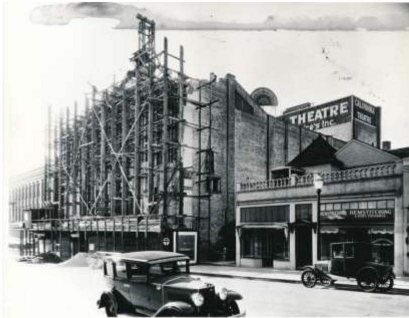
Figure 17. California Theatre under construction, 1929 or 1930 Swingle Collection, BAHA archives.
