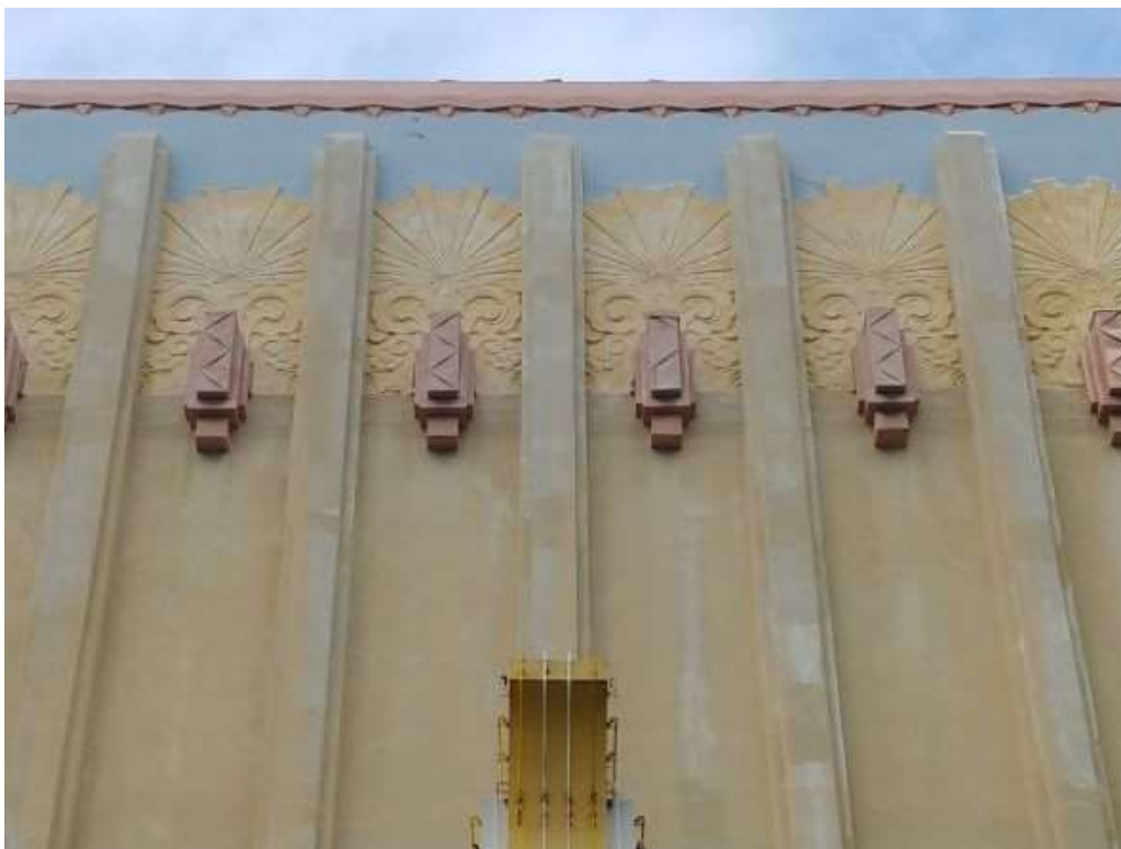
Figure 4. Art Deco details on façade, including piers, rectangular corbels, and “frozen fountain” bas-reliefs, November 2021. Photo: Therese Poletti
