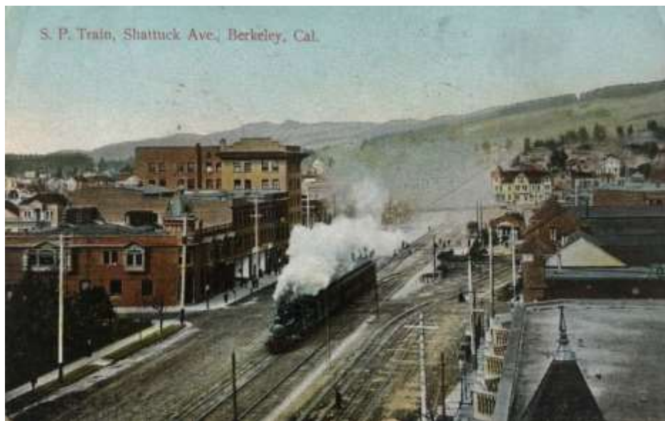
Figure 9. Southern Pacific station on Shattuck Avenue, circa 1909
