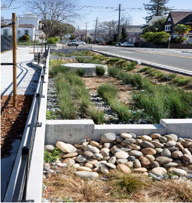
Green infrastructure installation at Woolsey Street
