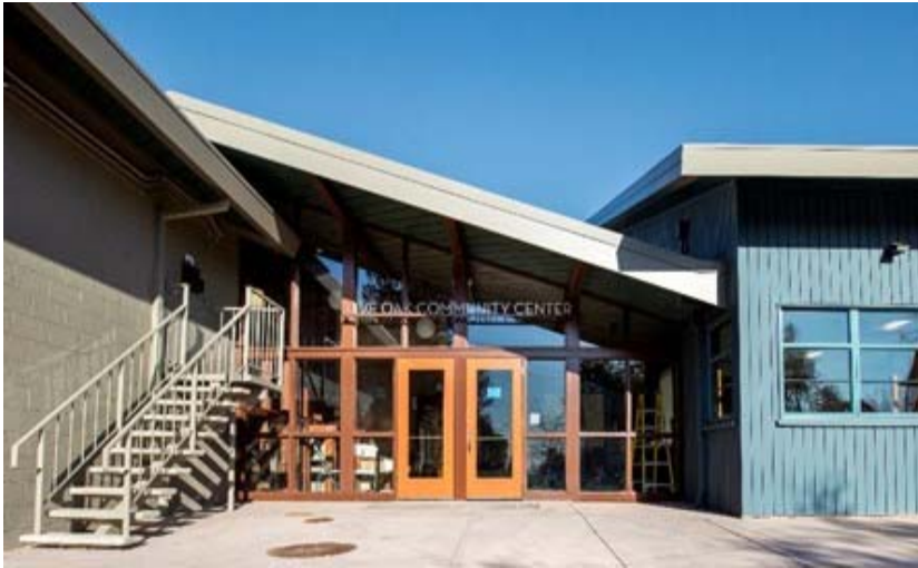
Renovated Live Oak Community Center
