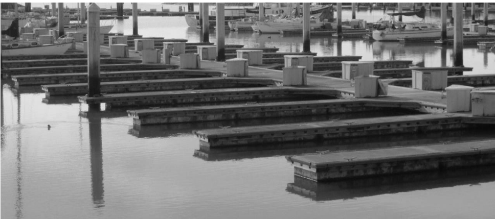
Former San Leandro Marina
