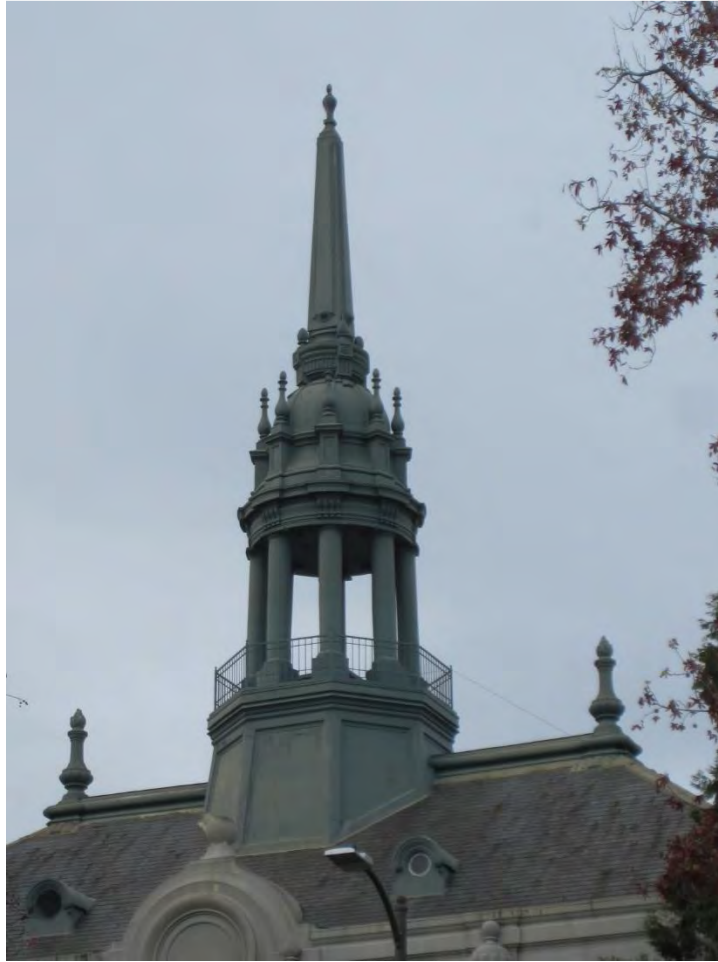
Figure 9. Tall Roof Spire with very light steel framing from 1909.
