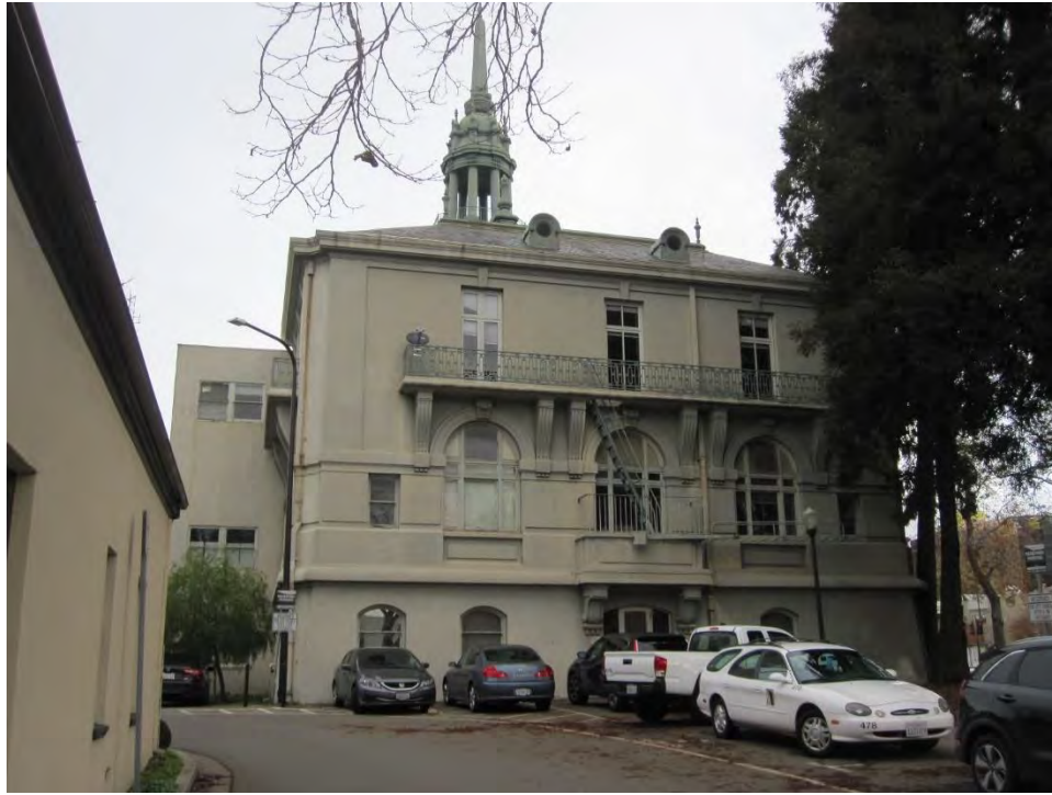
Figure 7. View looking north (south elevation)
