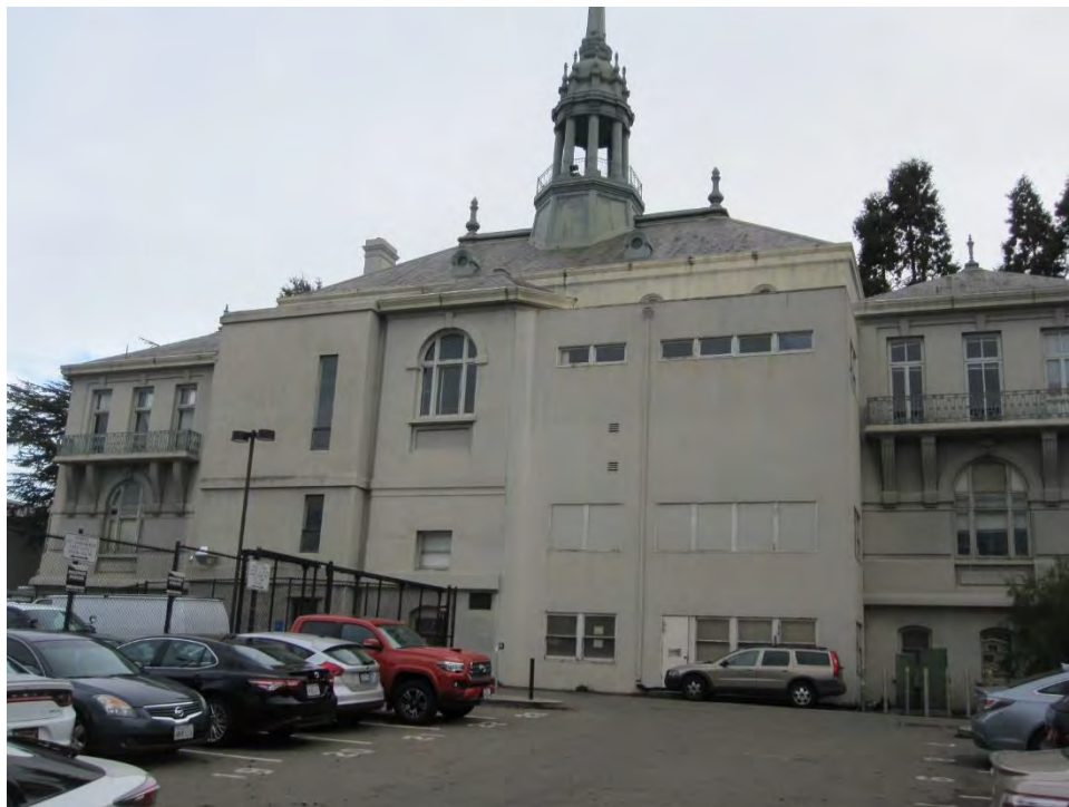
Figure 8. Rear view (west elevation), additions at center
