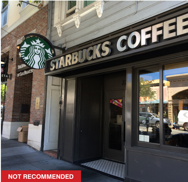
Design, including colors, finish, and texture, is inconsistent with the surrounding buildings.
