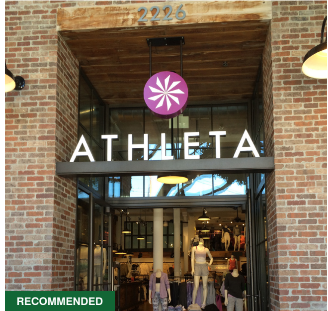
Sign does not extend out and beyond the width of the storefront opening.
