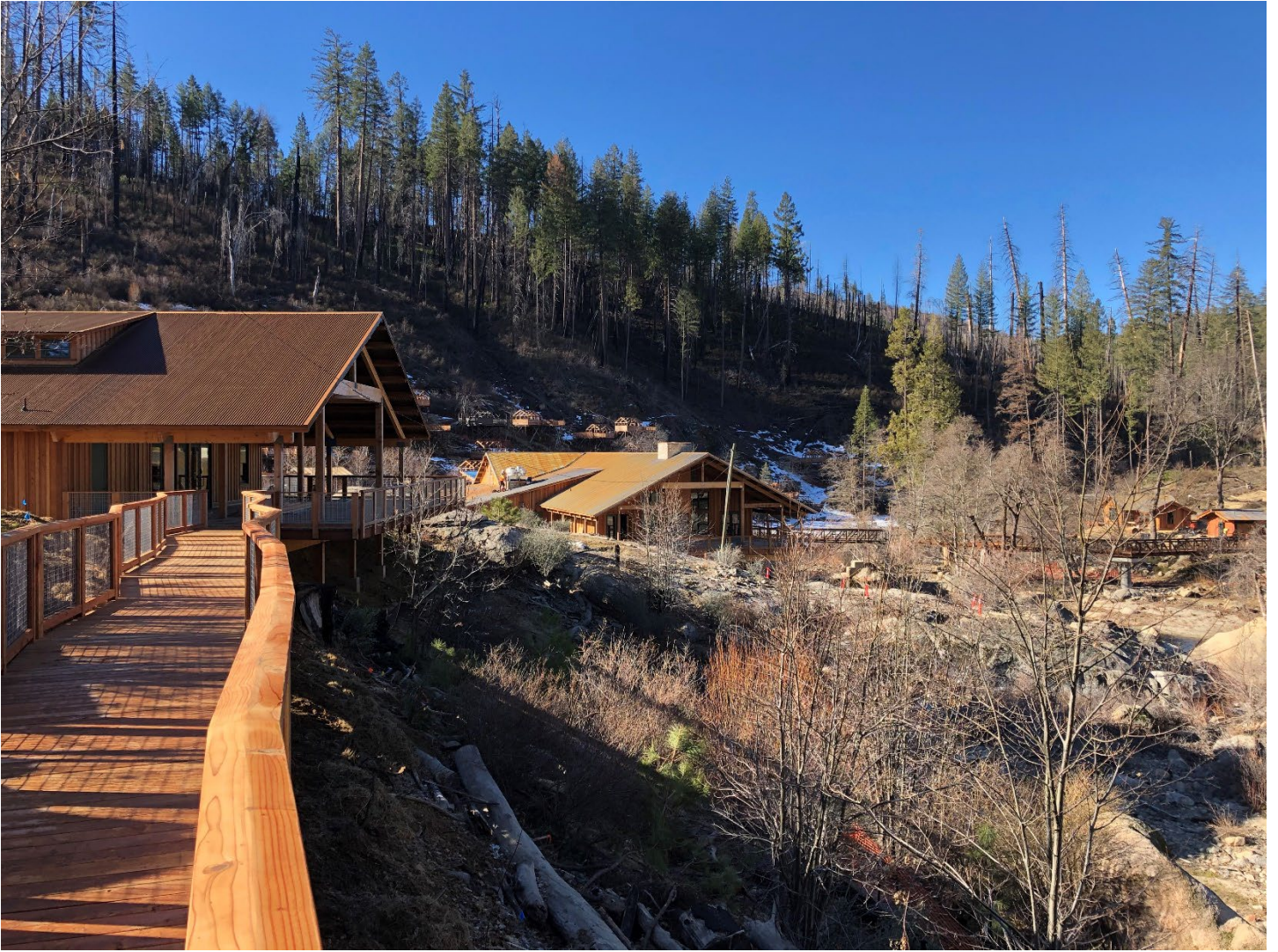
Boardwalk to Recreation Hall, Dining Hall in Background
