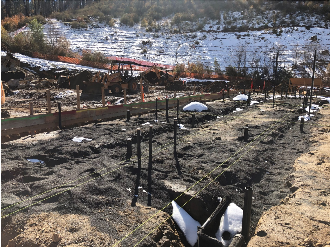
Preparing to Pour Concrete for Dining Hall Foundation
