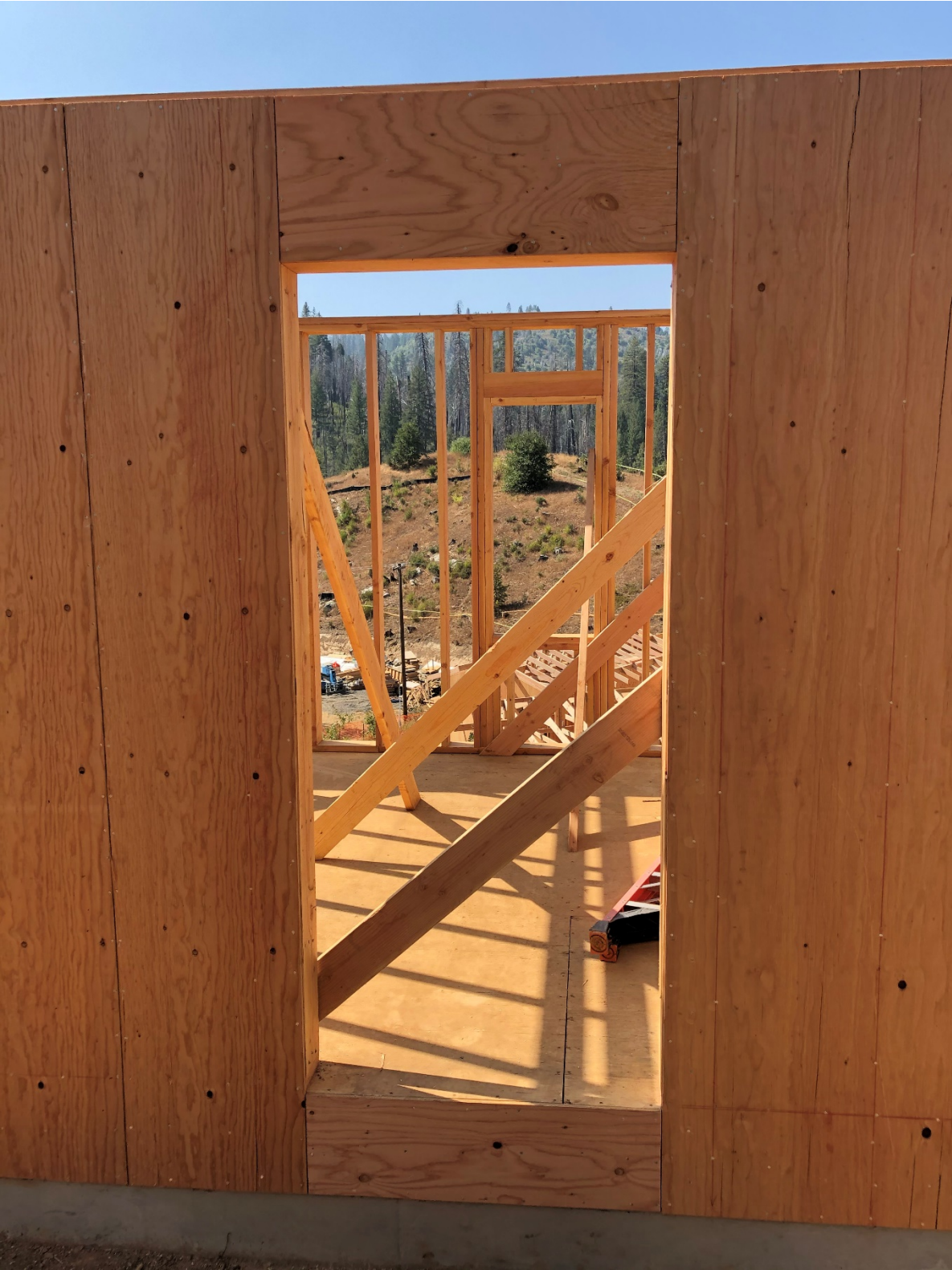
Staff Cabin Front Door
