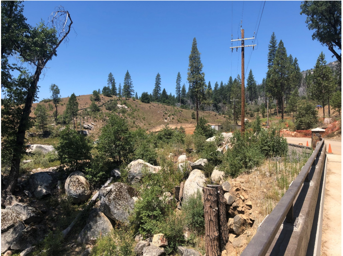
Looking towards Staff Camp from Hardin Flat Road Bridge
