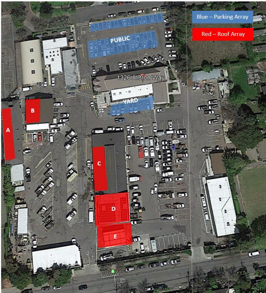
Figure 17: Potential locations for Solar PV Arrays
