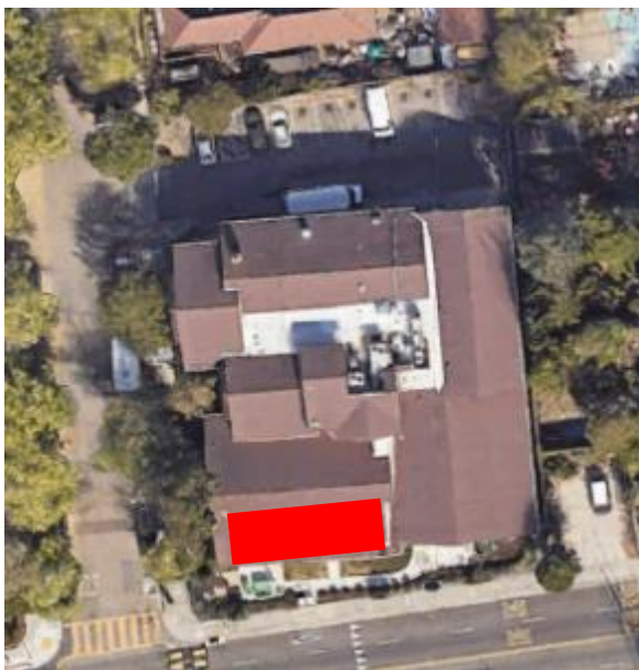
Figure 27 South Berkeley Senior Center facility aerial view
