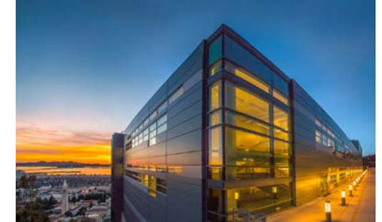
Activate Berkeley at Cyclotron Road
