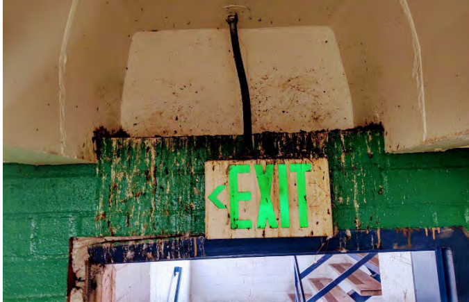
Layers of droppings on parking level
