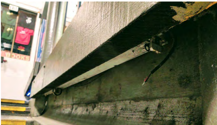
Unused light fixture with exposed wires
