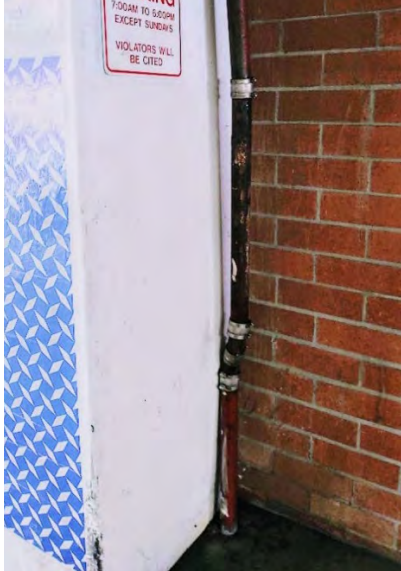
Leaking old drain pipe
