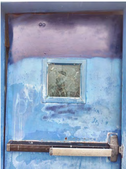
Heavily dented door with broken glass
