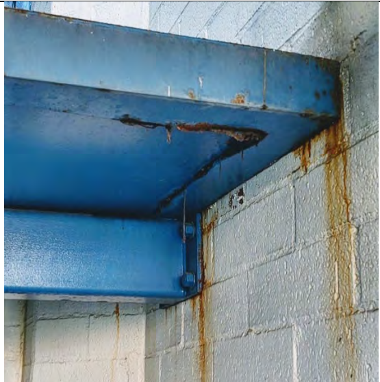
Significant water intrusion through bldg. seams
