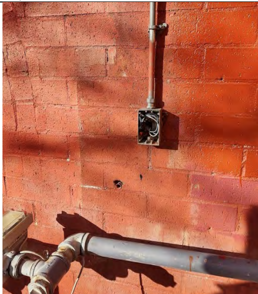
Exposed wires on exterior next to sidewalk
