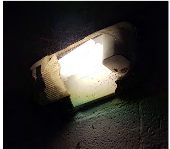
Broken light fixture
