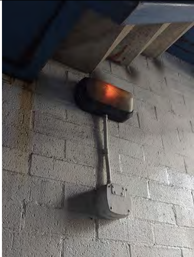
Unused light fixture with exposed wires
