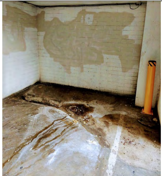
Sludge accumulated around floor drain near elevators
