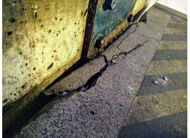
Crumbling concrete on steps
