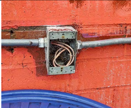
Exposed wires on exterior next to sidewalk
