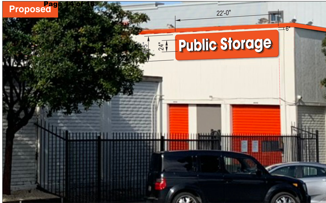
CORNER OF 2ND ST & HARRISON ST BLDG F & A - STORAGE NEW REVERSE PAN CHANNEL HALO LED ILLUM'D LETTERS - PANEL SIGN
