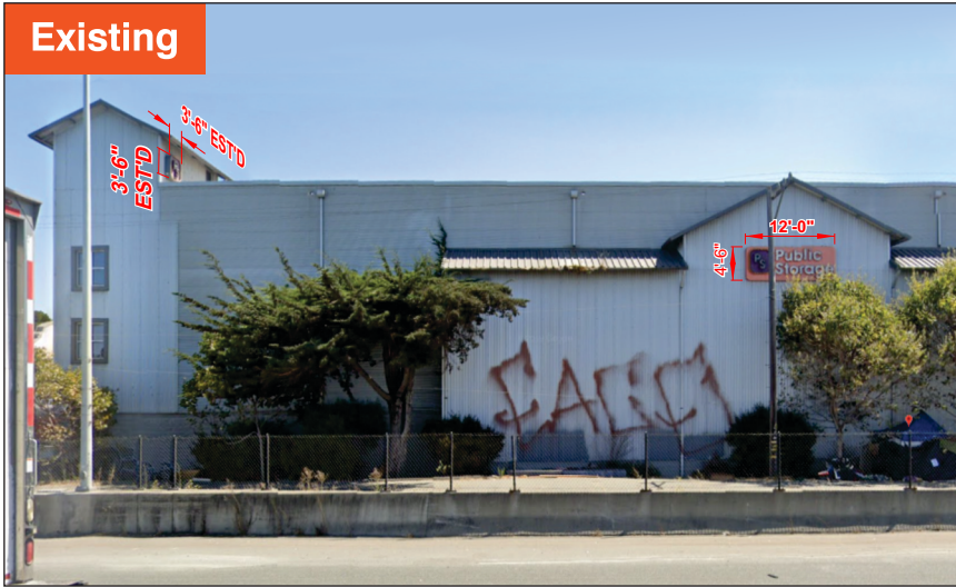
WEST ELEVATION BLDG C - STORAGE REMOVE & DISCARD EXISTING OPEN FACE CL SIGN
