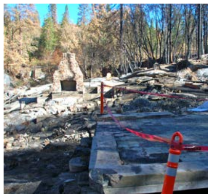
Dining Hall after fire (10/30/13)
